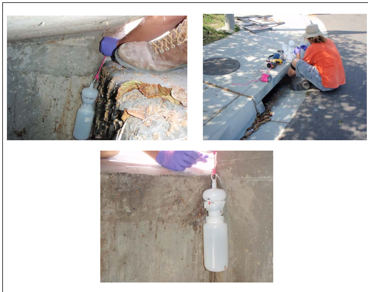
Figure 2-2. Example of Nalgene Sampler Installation
