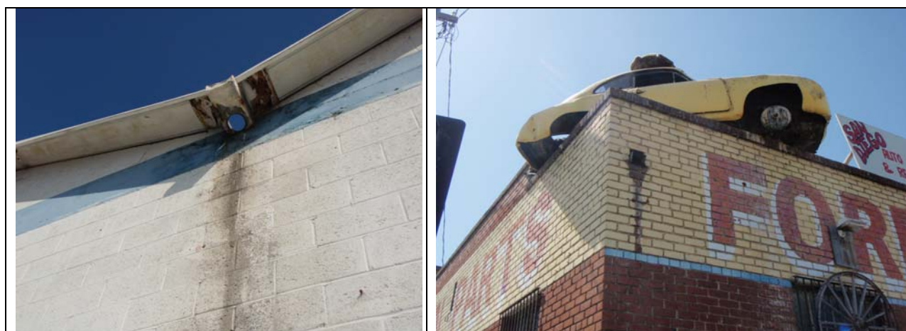
Figure 3-11. Facilities with Staining on Parcels from Rooftops Draining Directly to City Streets
