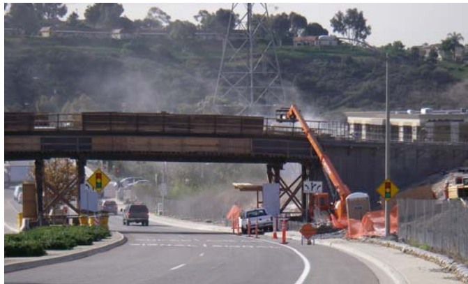
Sandblasting Photo. Source: WESTON, 2006.
