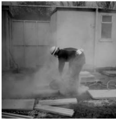
Concrete Cutting Photo Source: Health and Safety Executive (CIS No. 54)
