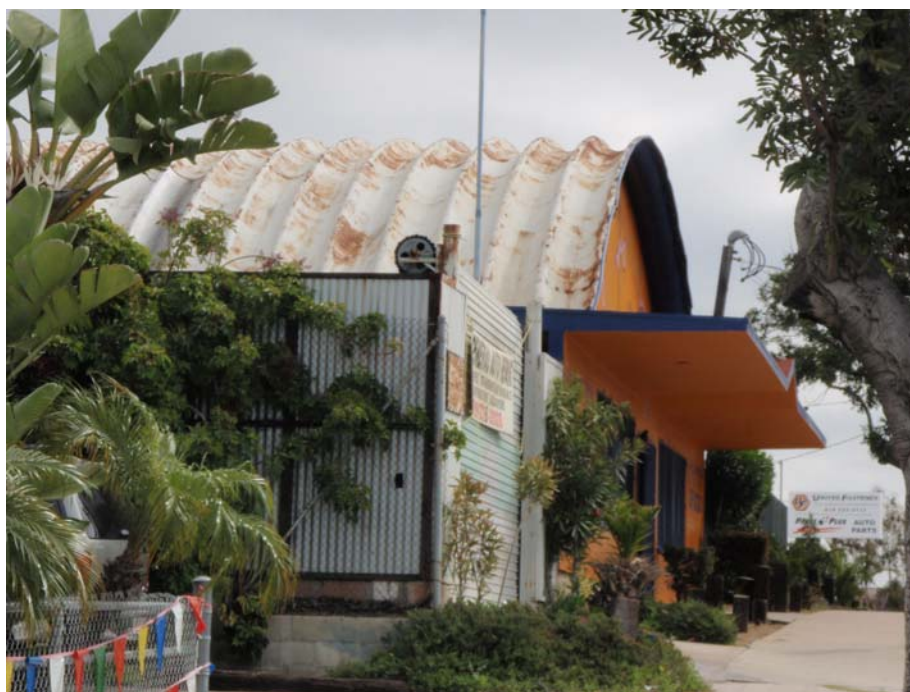
Figure 5-3. Example of Area of Influence on High Zinc Concentrations in Storm Water Runoff from a Commercial/Industrial Drainage Area in Priority Sector 1
