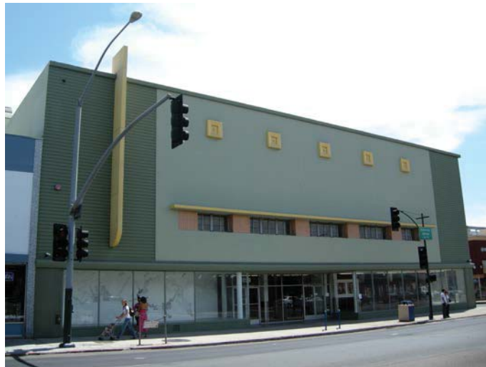
J.C. Penney Co. Building, 3029 University Avenue.
