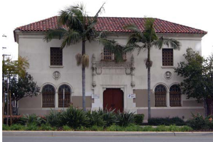
San Diego Gas & Electric Co. Substation F, 3169 El Cajon Boulevard.
