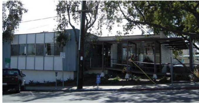
University Heights Branch Library, 4193 Park Boulevard.
