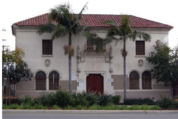
San Diego Gas & Electric Co. Substation F.
