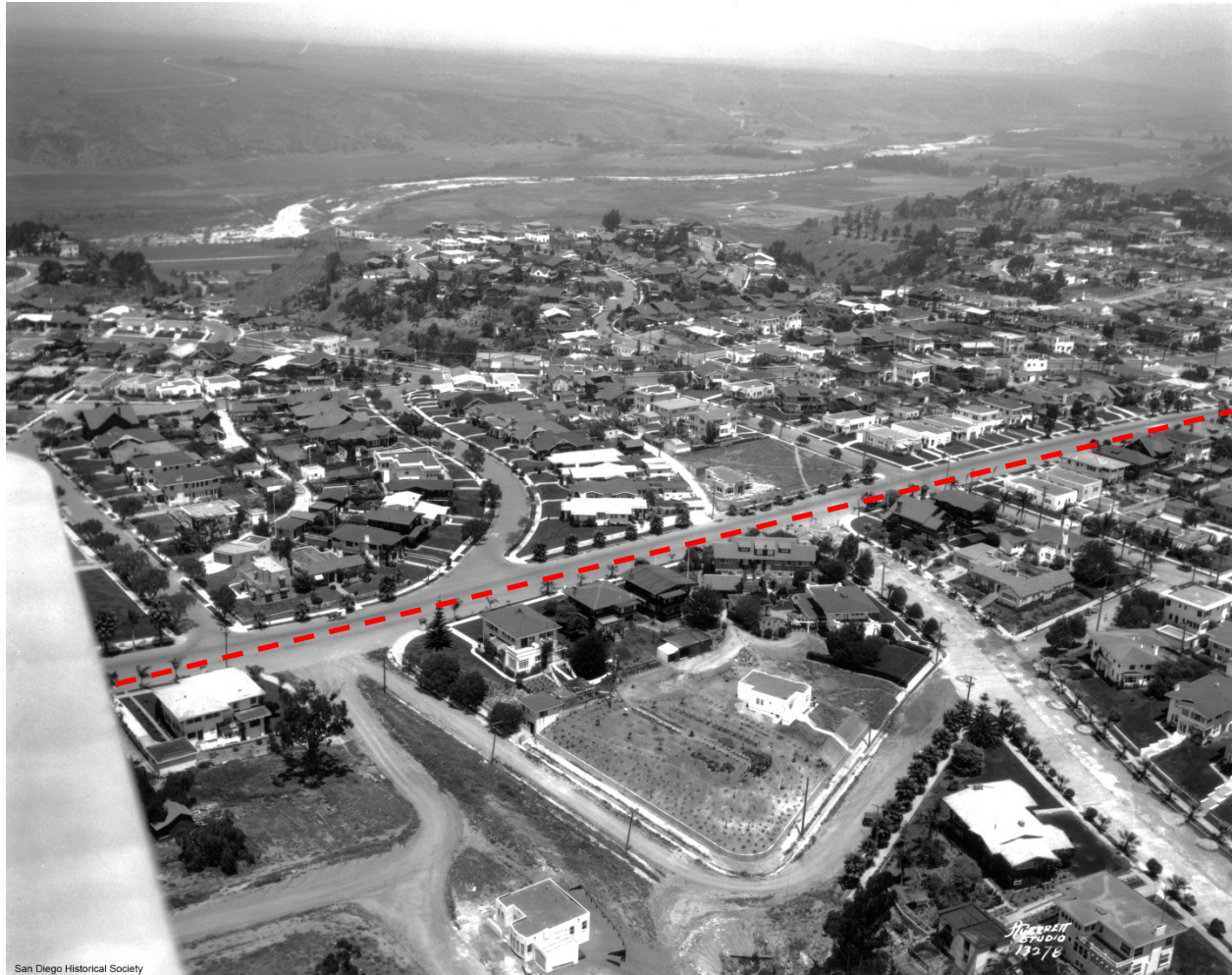
Figure 8 Aerial view, Inspiration Heights below/south of the dashed red line (corresponds with Sunset Boulevard), 1927, view northeast. San Diego History Center.
