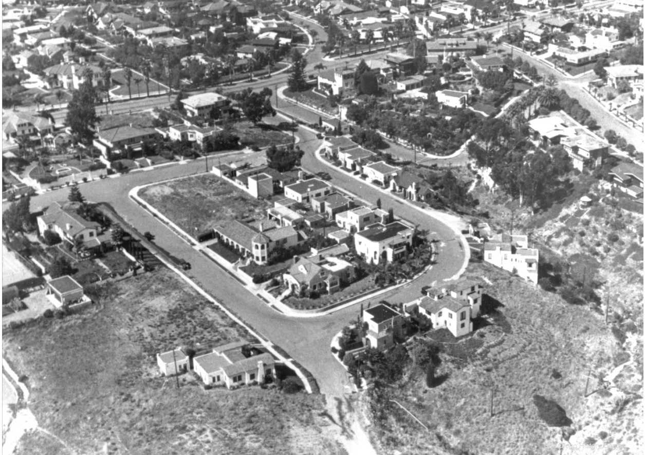
Figure 9 Aerial view, Miller Street and Arden Way in foreground, circa 1930s, view northeast. San Diego History Center.
