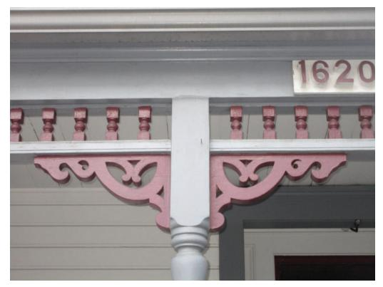
Figure 3-7: Detail photo showing the decorative wood spindlework and decorative column brackets at the front porch.
