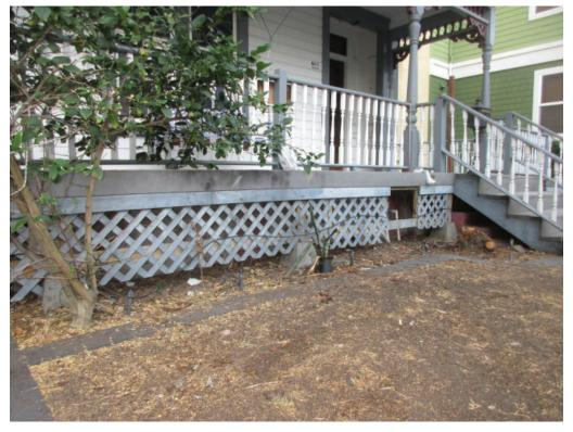
Figure 3-10: Looking northwest at the front porch, front porch stairs and railing. The front porch is non-historic and has been replaced with OSB boards.
