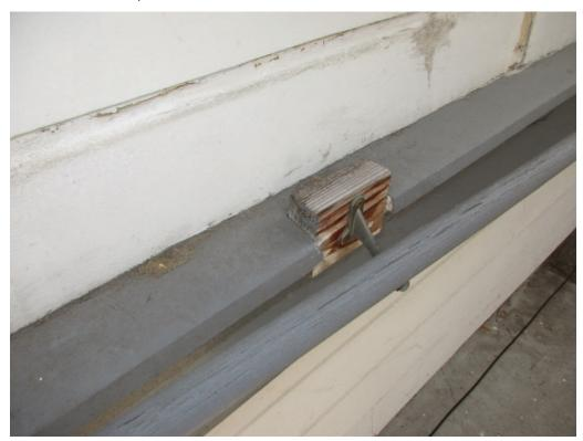
Figure 3-14: Detail photo showing the impact to the base trim boards from the accessibility ramp handrail atachments.
