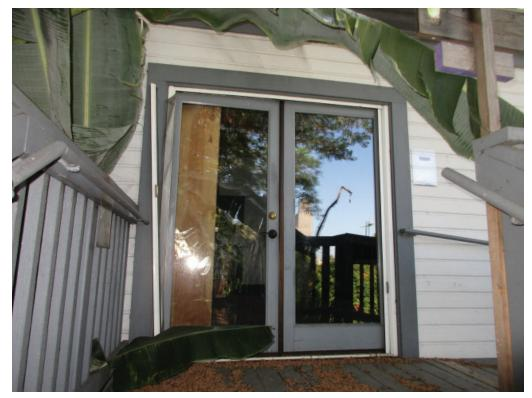
Figure 3-17: Looking east at the west facade showing the non-historic pair of wood french doors.
