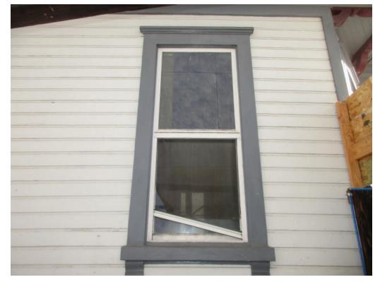
Figure 3-15: Detail photo showing a typical replacement clad wood window with dual glazing and vinyl window screens.
