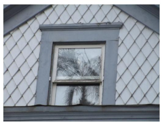
Figure 3-6: Looking west at the gable end of the east facade showing the diamond shaped wood shingles and replacement double hung window.
