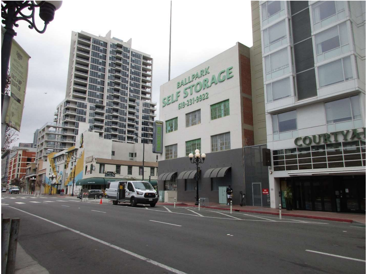
05 CONTEXT VIEW LOOKING NORTHEAST AT THE WEST FAÇADE. A SMALL PORTION OF THE SOUTH FAÇADE IS VISIBLE SHOWING THE CONCRETE POST AND BEAM FRAMING WITH BRICK INFILL.
