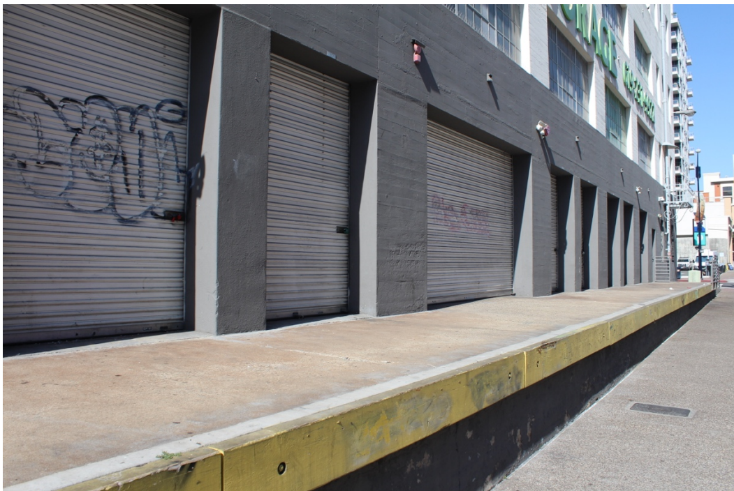
Figure 8: Concrete loading dock and steel roll-up doors on the east side. The dock will be reconstructed with railings and planters added. The doors will be replaced with new glazed storefronts to serve the new uses.
