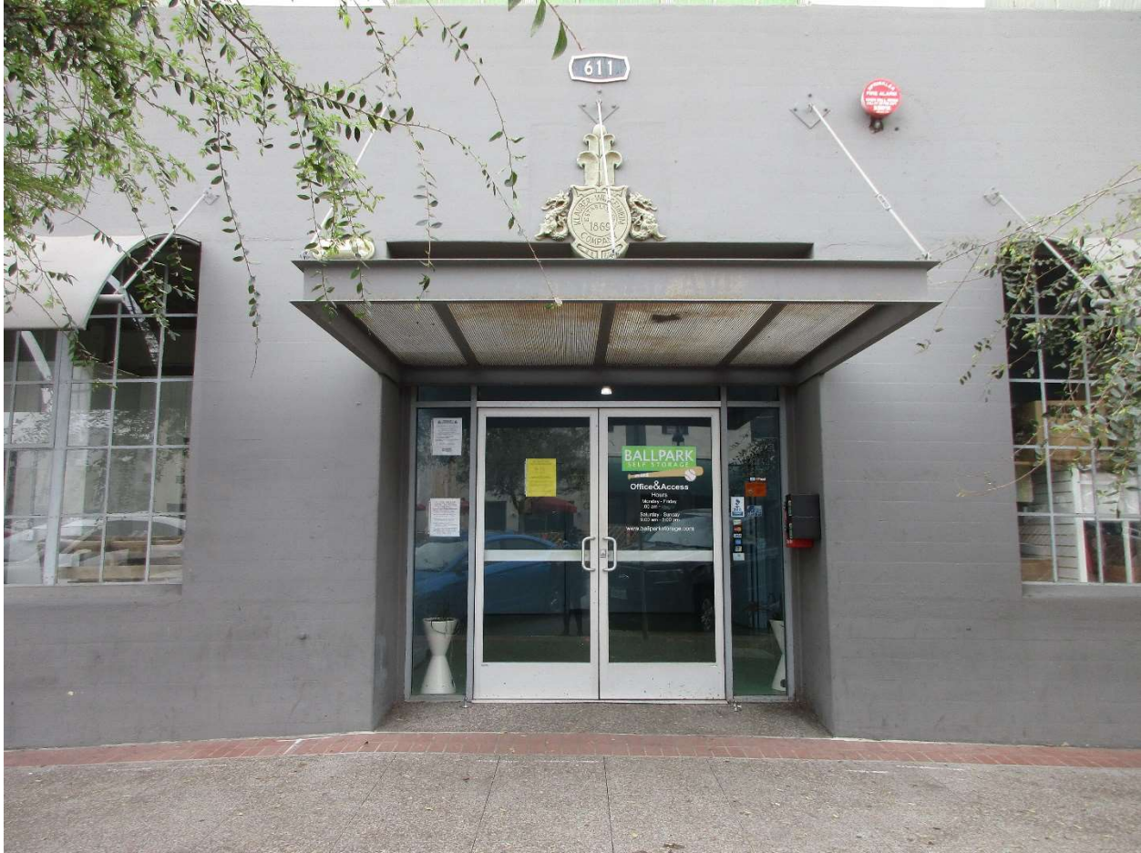
06 LOOKING SOUTH AT THE PRIMARY ENTRANCE AT THE NORTH FAÇADE. THE ENTRY CONSISTS OF CONTEMPORARY ALUMINUM STOREFRONT DOORS WITH SIDELITES AND AN ADDED STEEL CANOPY.
