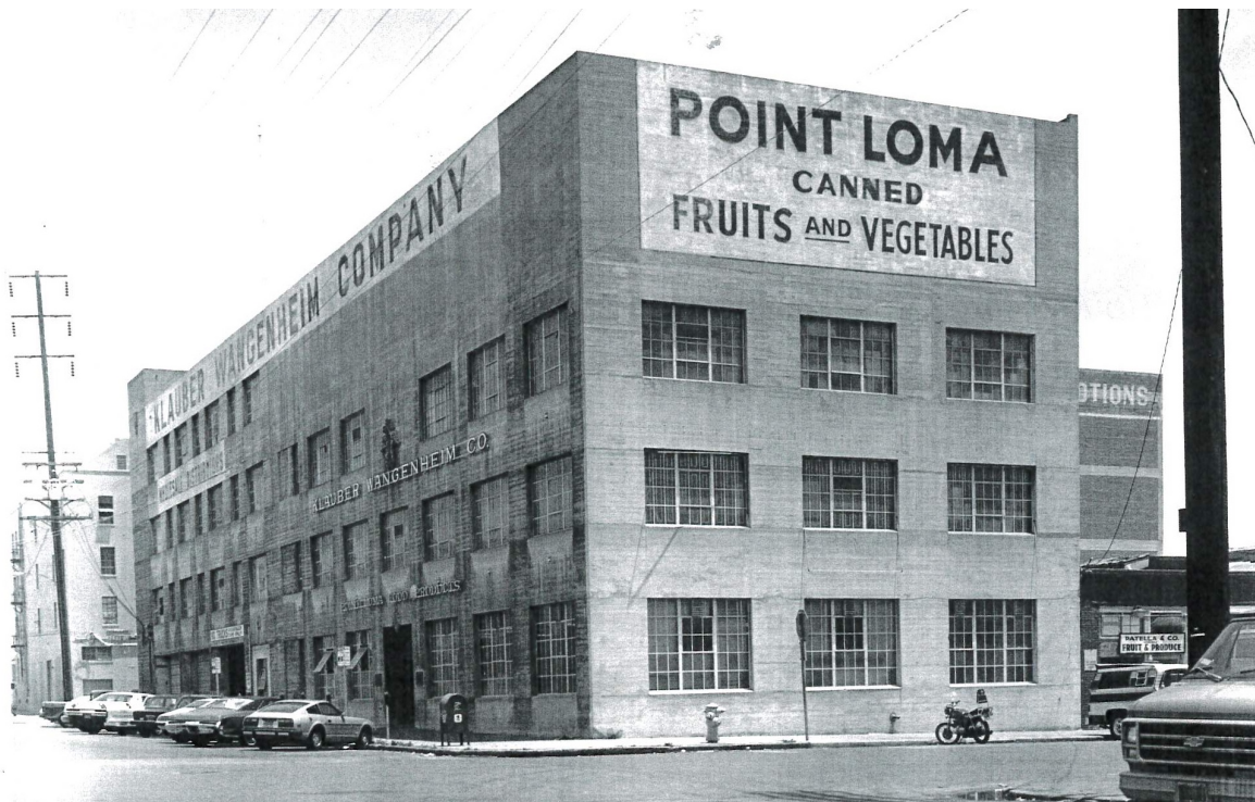
Figure 4: 1980 Photo looking southeast. Note the upper floor addition and added signage.
