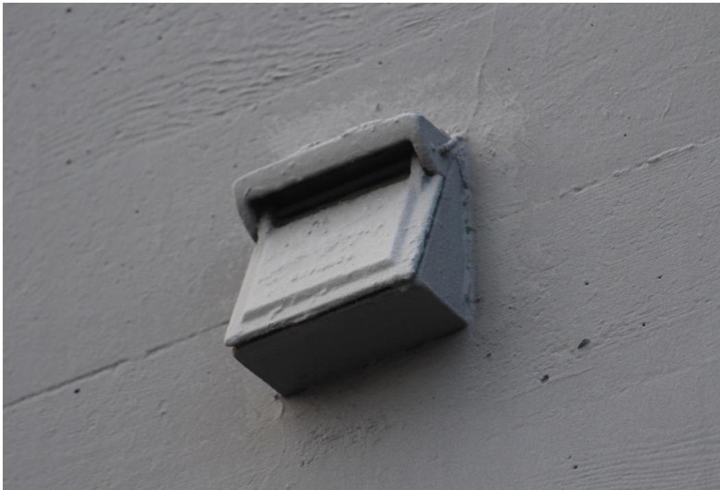
Figure 16: A cast-iron floor scupper with a hinged door. These facade features will be protected-in-place.
