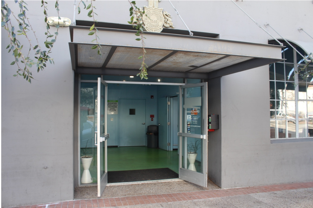
Figure 9: The main entry at the north facade has non-historic aluminum doors and transoms. The steel canopy is also contemporary. The shield above is historic (see Figure 13).
