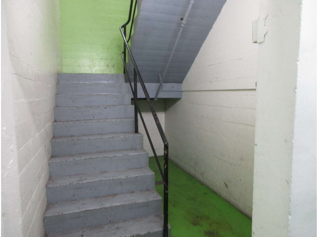
16 CAST-IN-PLACE CONCRETE STAIRS WITH METAL RAILING. STAIR CORE WALLS ARE CONSTRUCTED FROM BOARD-FORMED CONCRETE. LOOKING NORTH IN THE CENTRAL STAIR CORE AT THE FIRST FLOOR.
