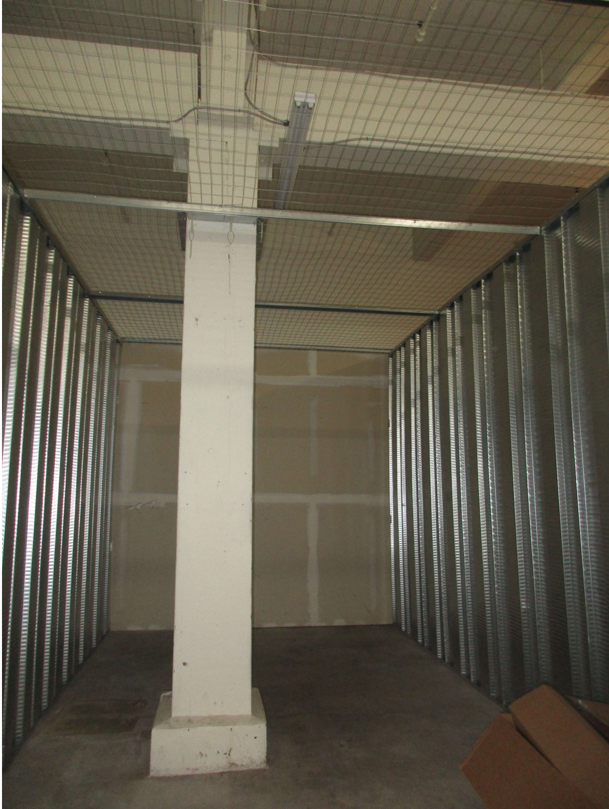
14 LOOKING SOUTH AT THE INTERIOR OF A TYPICAL CORRUGATED STEEL WALL SELF-STORAGE UNIT ON THE FIRST FLOOR.
