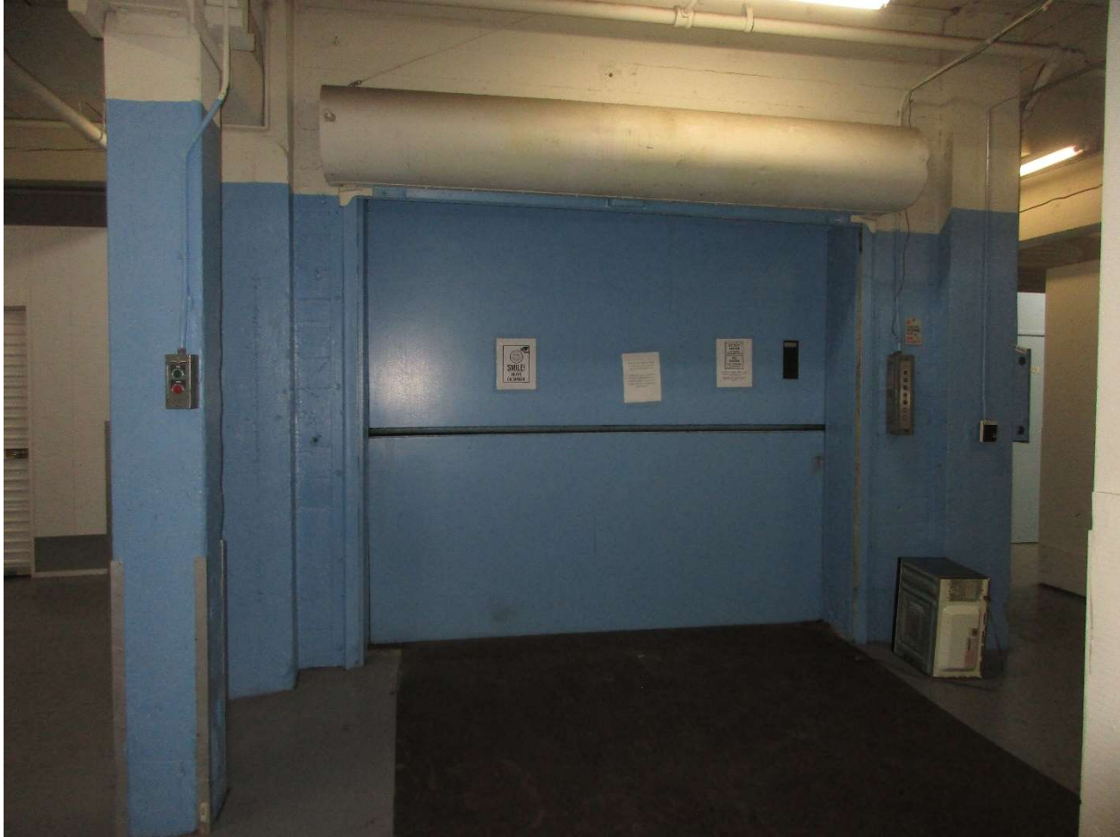
18 LOOKING EAST AT THE EAST FREIGHT ELEVATOR ON THE SECOND FLOOR.
