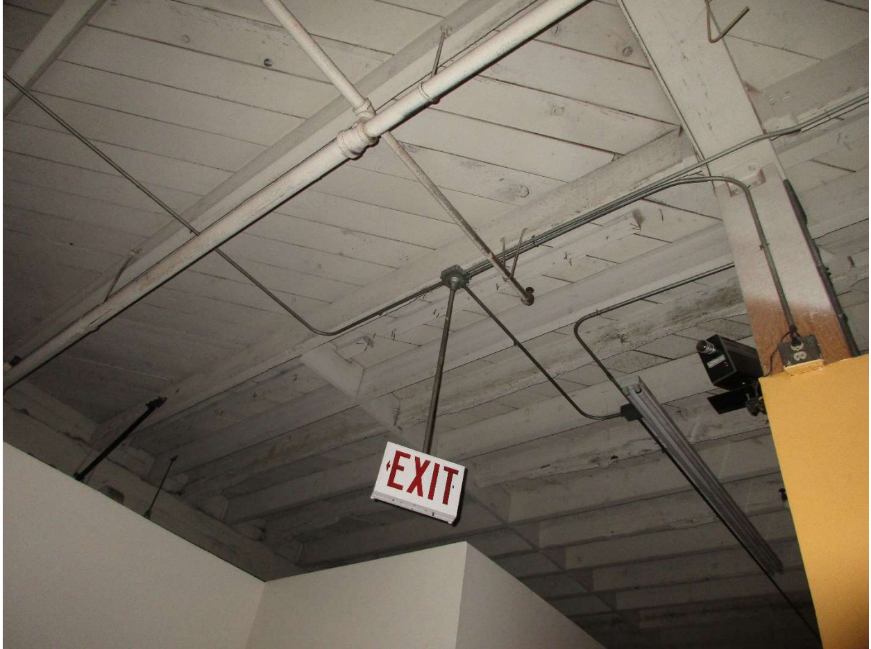
17 LOOKING SOUTHWEST AT THE ROOF FRAMING AT THE WEST WING FORTH FLOOR.
