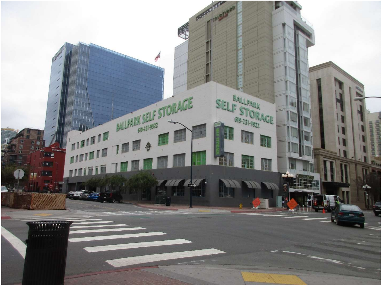
01 LOOKING SOUTHEAST ACROSS ISLAND AVE AND SIXTH STREET INTERSECTION AT THE BALLPARK STORAGE BUILDING.
