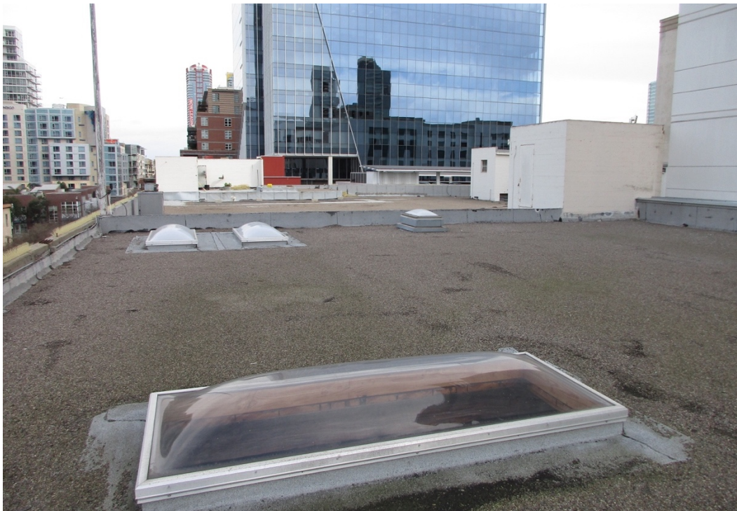
Figure 18: Rooftop view looking east. The roofing, added skylights and penthouses will be removed. The wood flagpole on the left will be retained or replaced in-kind.
