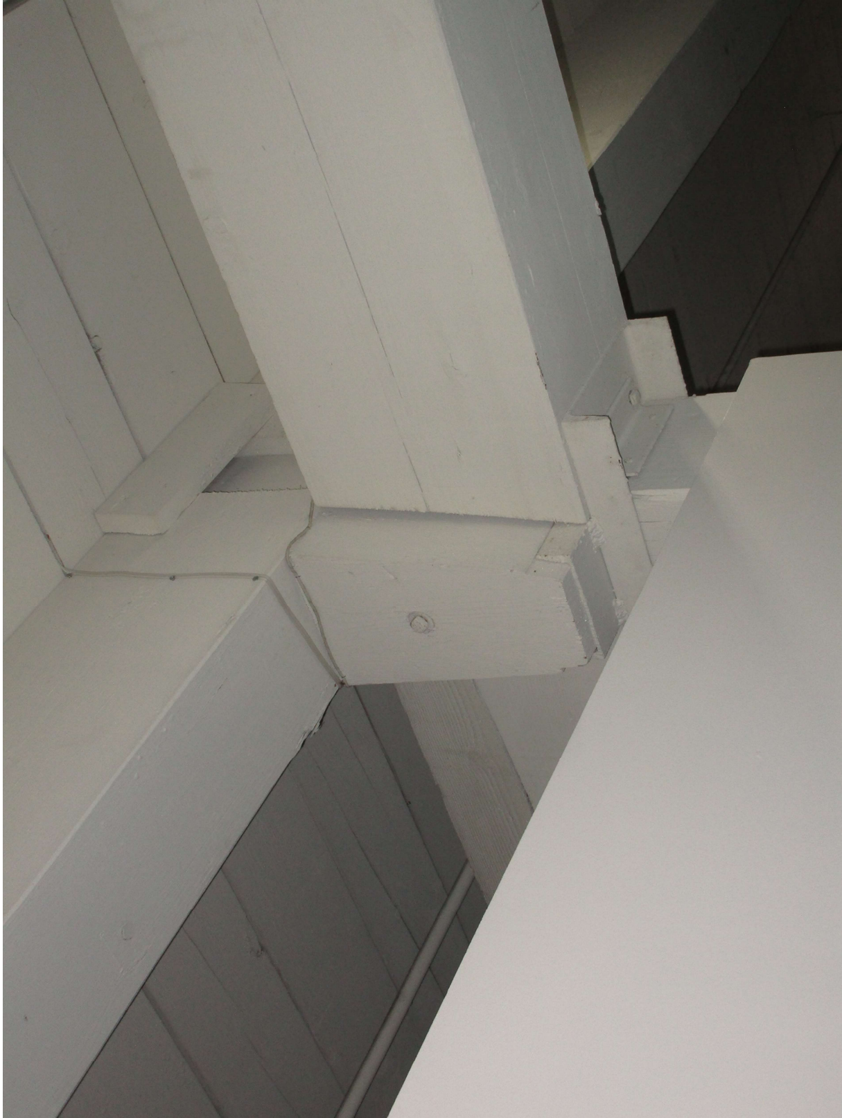
12 TYPICAL WOOD TIMBER COLUMN AND BEAM CONNECTION WITH STEEL CHANNELCAPITALS SUPPORTING THE WOOD TIMBER BEAMS.
