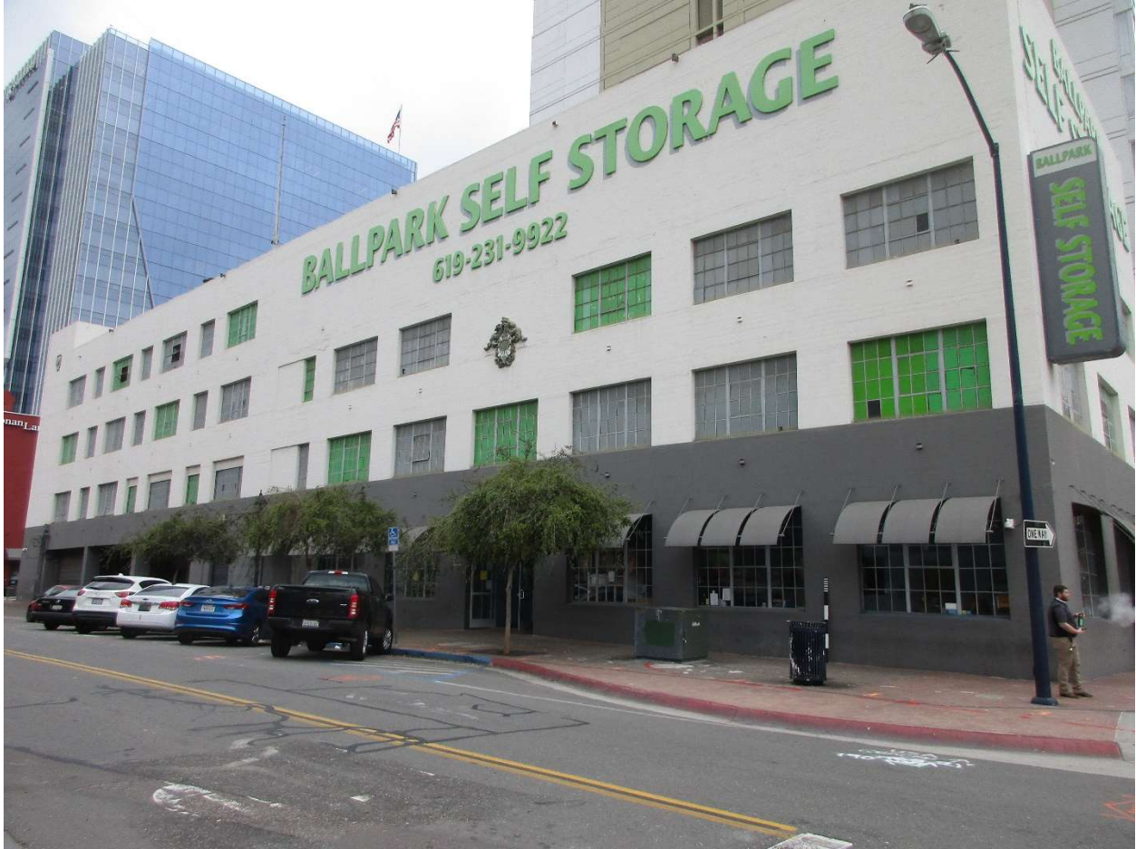
03 LOOKING SOUTH ACROSS ISLAND AVE. AT THE PRIMARY NORTH FAÇADE (WITH SCALE STICK).
