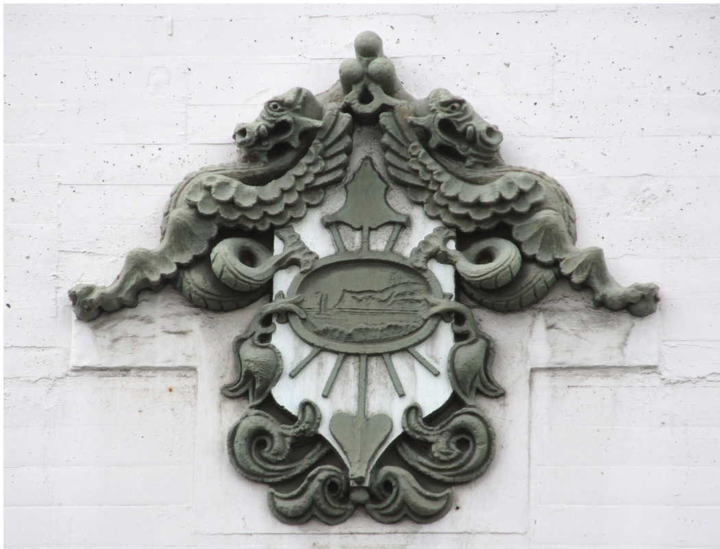
Figure 12: This cast-stone shield features sea monsters and an image of Point Loma. It is on the north facade and will be protected-in-place.
