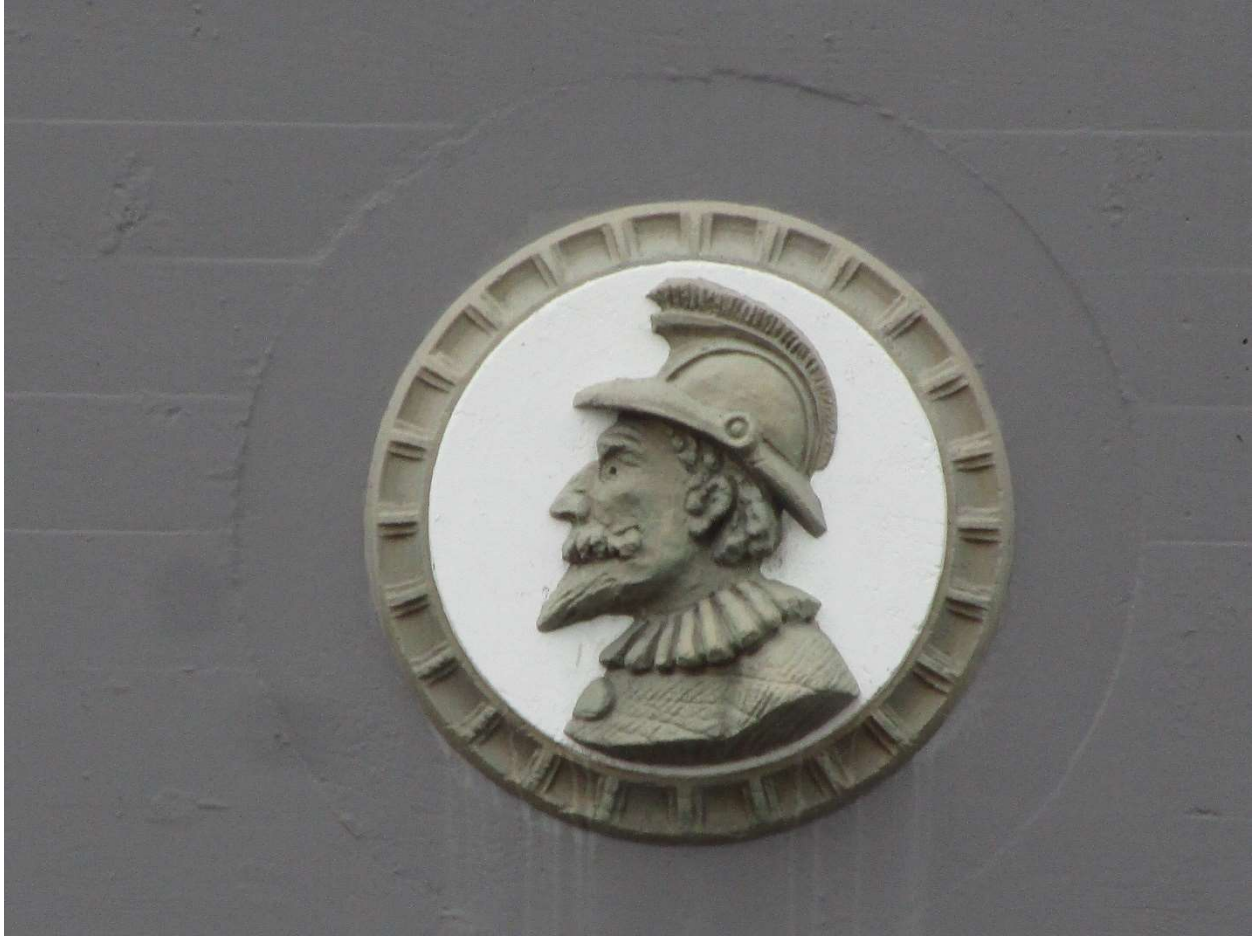
08 CAST-STONE DECORATIVE “CABRILLO” SHIELD LOCATED ABOVE THE FIRST FLOOR ON THE NORTH FAÇADE.
