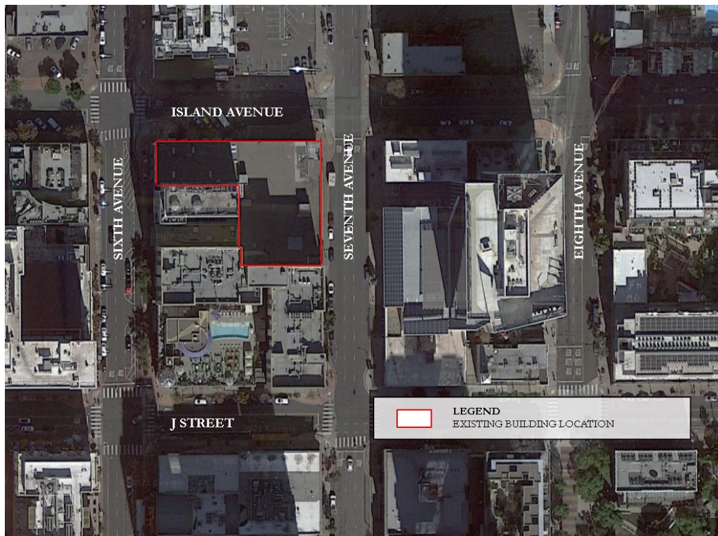
Figure 2: Existing building site at 611 Island Avenue.
