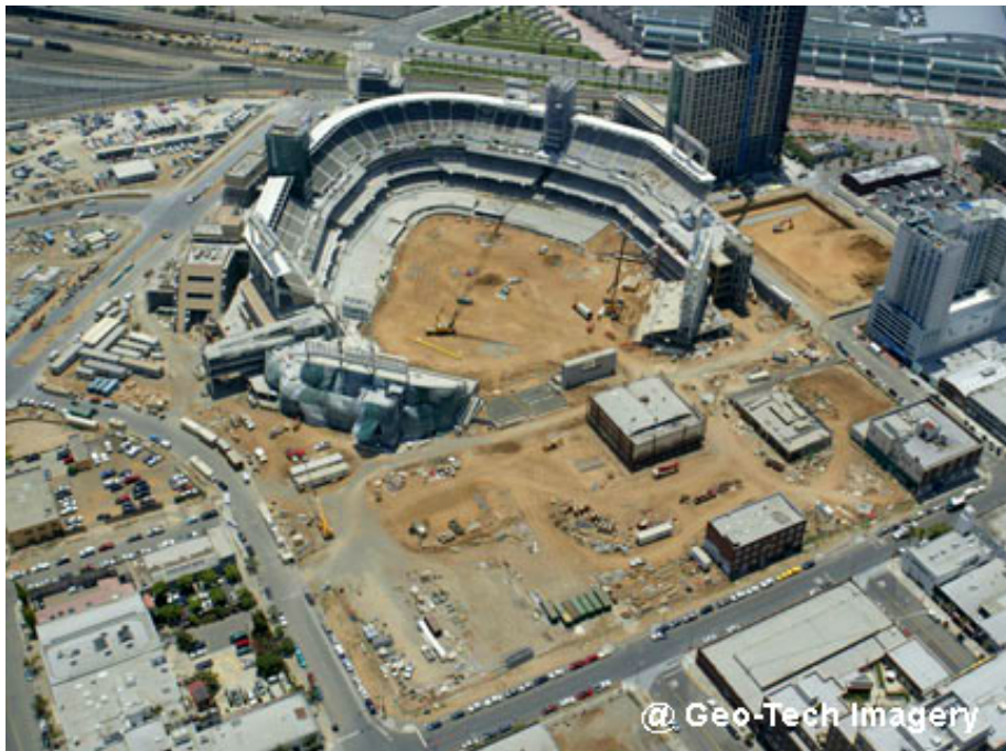
Petco Park under construction 2003
