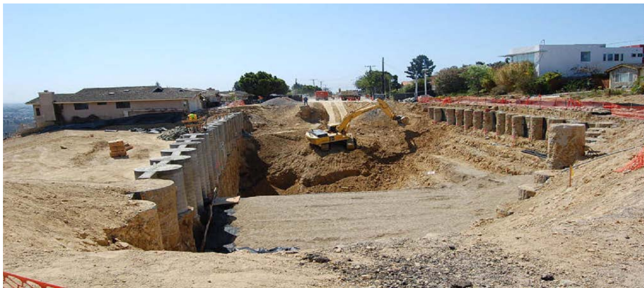
Soledad Mountain Road repair
