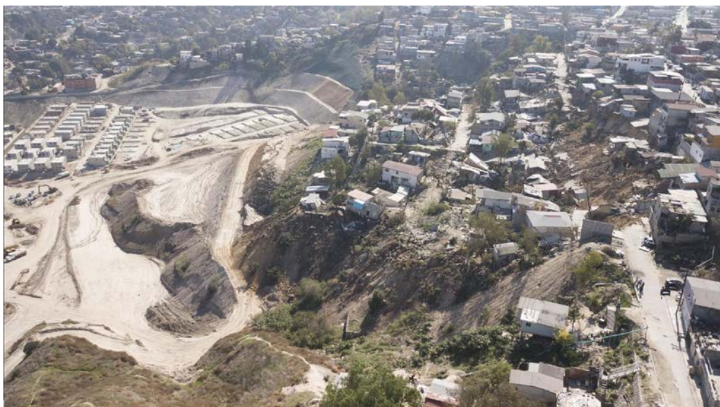
Landslide in the Lomas del Rubi neighborhood of Tijuana, 2018. Note recent grading.
