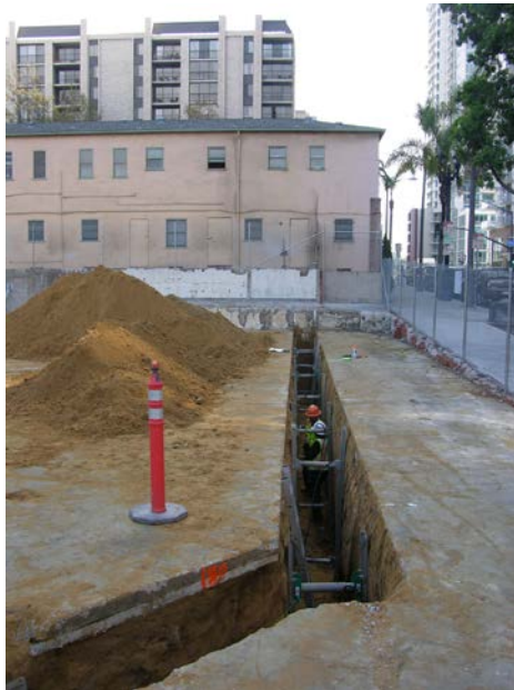
Trench excavated for fault investigation in downtown San Diego.
