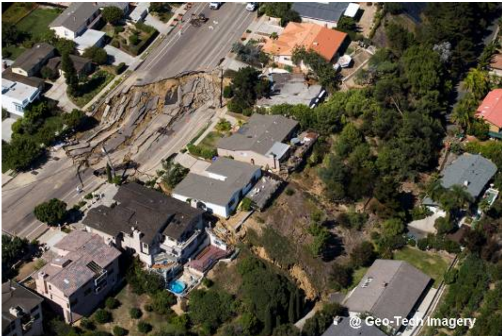
Soledad Mountain Road Landslide October 2007
