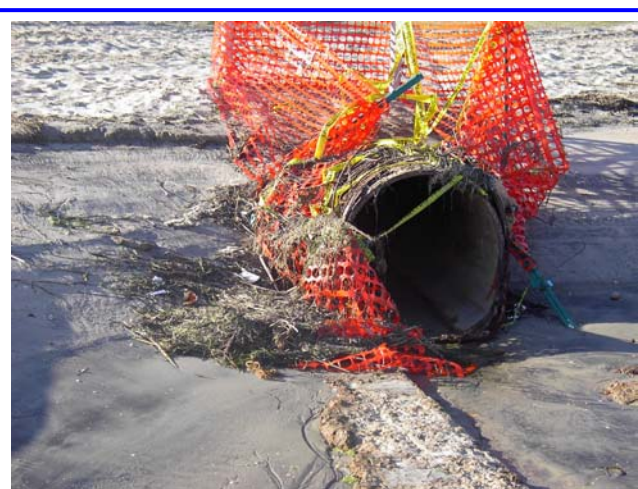
Storm drain SD5-2 at Wildlife Refuge
