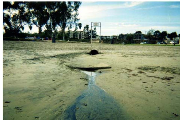
Groundwater spring below storm drain SD5-2
