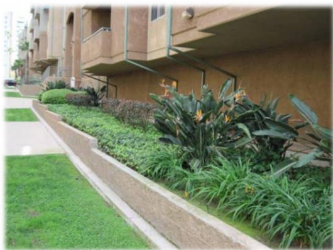
Figure I-4. Planter box adjacent to building
