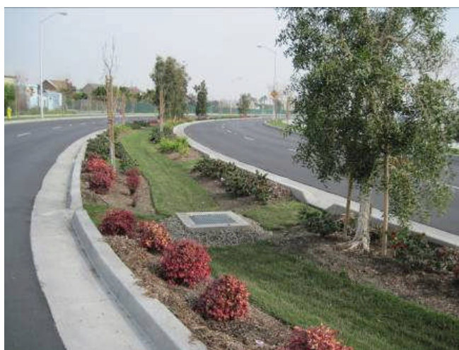
Figure I-3. Road median bioswale
