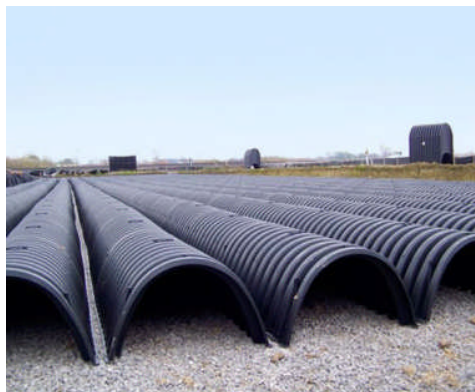
Figure I-13. Example of an infiltration gallery during construction
