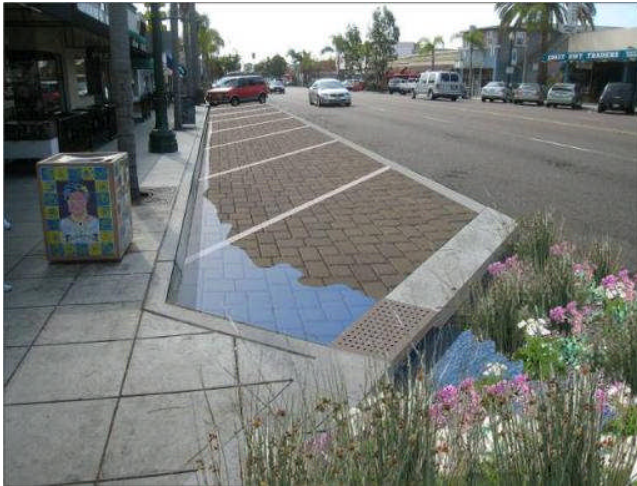
Figure I-5. Permeable pavement parking area in the right-of-way
