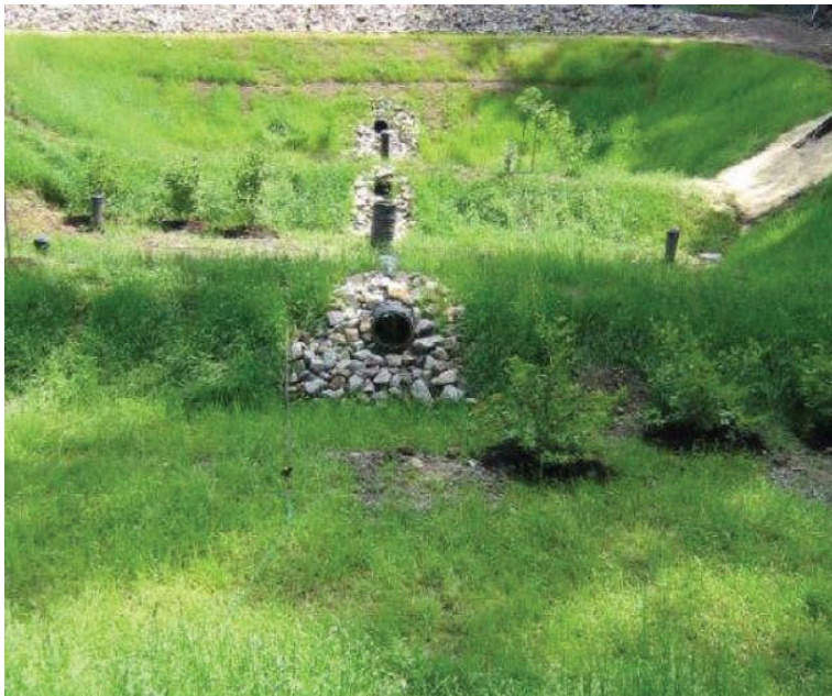
Figure I-17. Example of a subsurface flow wetland
