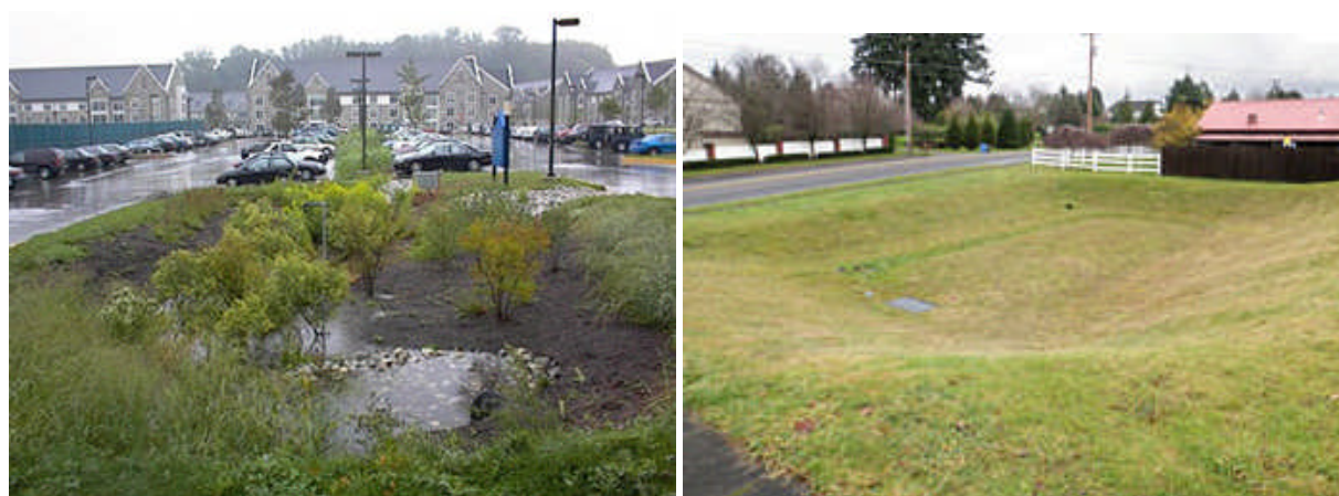
Figure I-12. Typical surface infiltration basins
