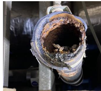
Father Joe's Villages Paul Mirabile Center Plumbing Renovation
