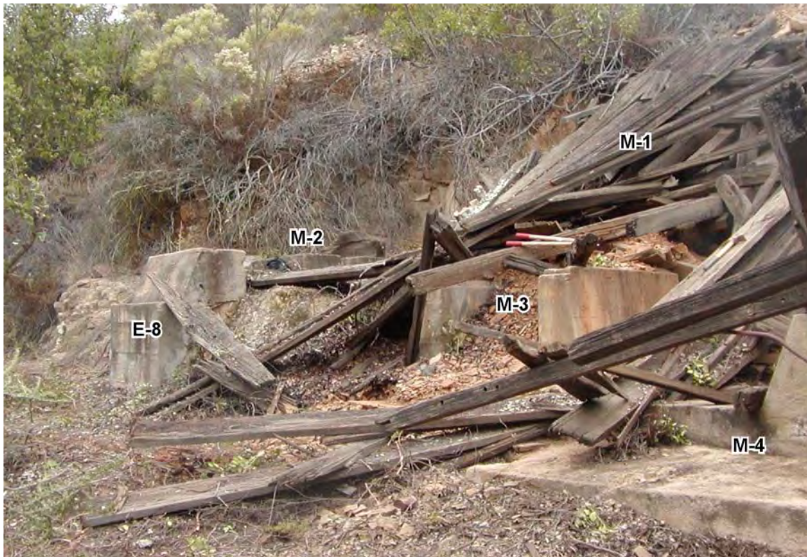
Figure 6. Core processing area showing the collapsed ore bin (M-1), and concrete footings for machinery used in ore processing.
