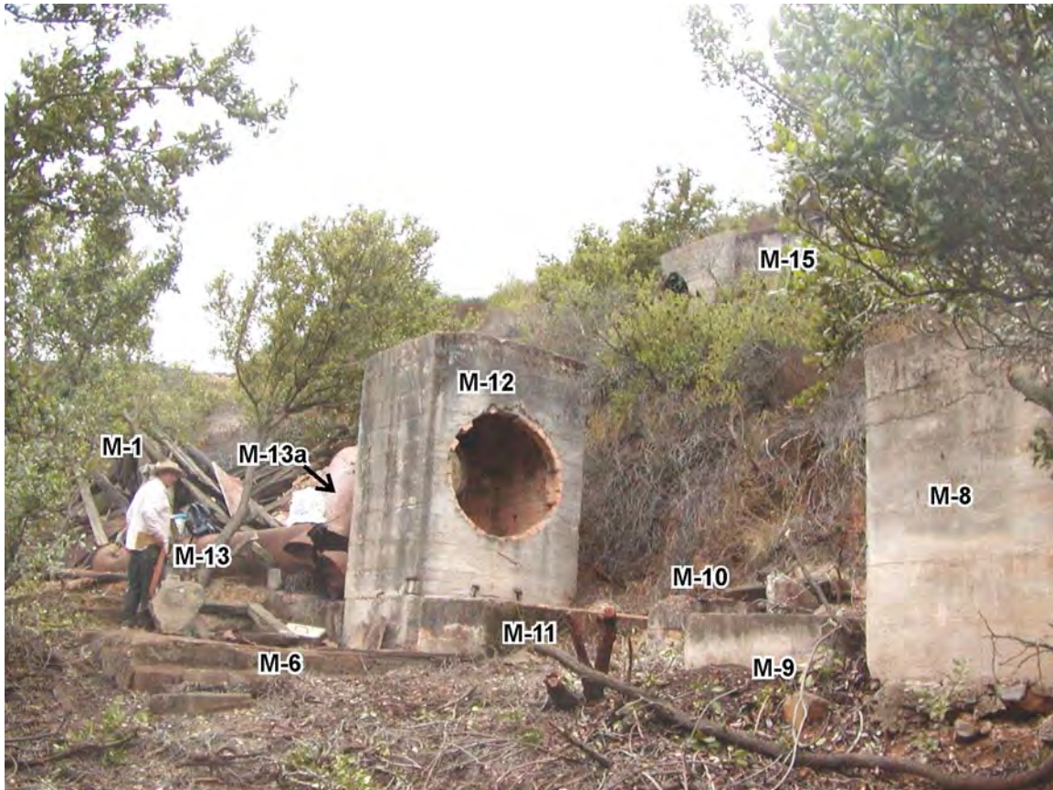
Figure 7. Core processing area showing the remains of the rotary roaster in the foreground. The dust chamber is in the background.
