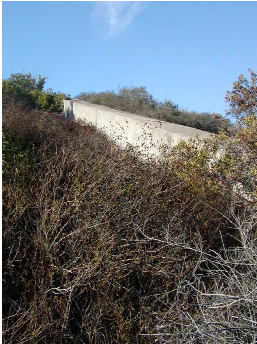
Figure 8. The southwest side of Feature M-15, the concrete dust chamber.
