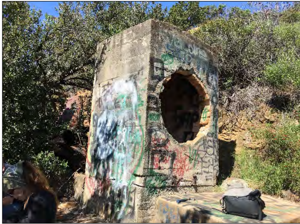
Ore roaster support structure.
