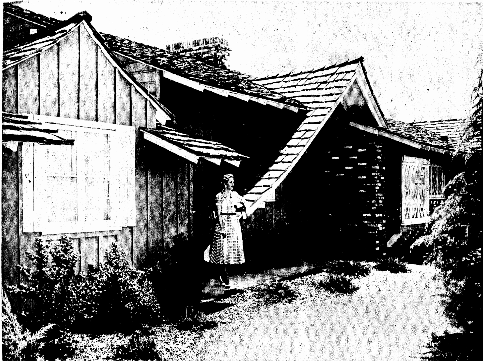
THIS ENGLISH COLONIAL ROOF LINE IS AT 3028 GARRISON ST. WHERE MRS. EDWARD STROP POSES AT EAVED EXTENSION OVER ENTRY.
