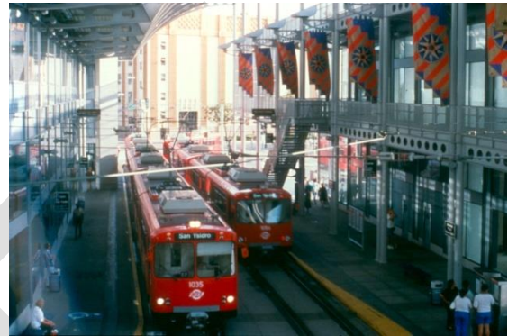
The American Plaza Trolley Station downtown provides an architecturally integrated, “front door” experience for transit patrons.
