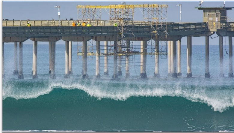
Ocean Beach Pier Improvements
