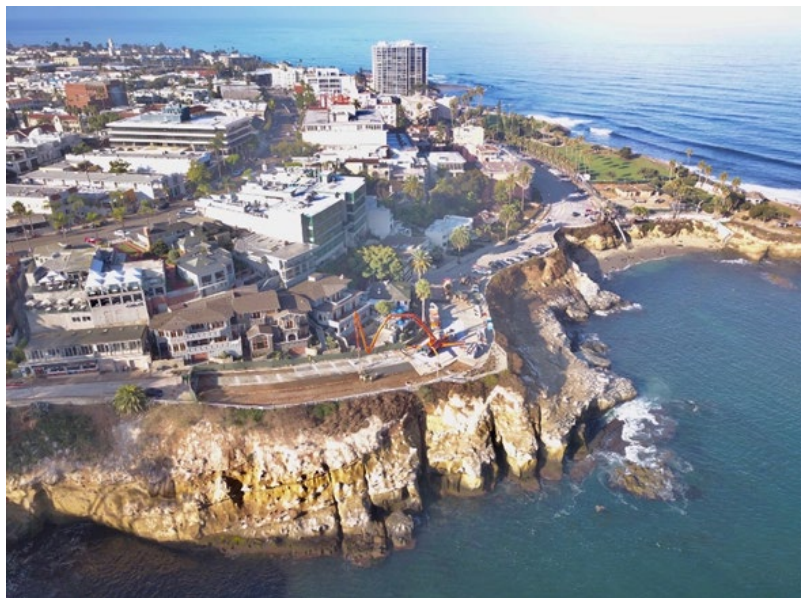
Coast Sea Cave Emergency Stabilization Project (La Jolla)
