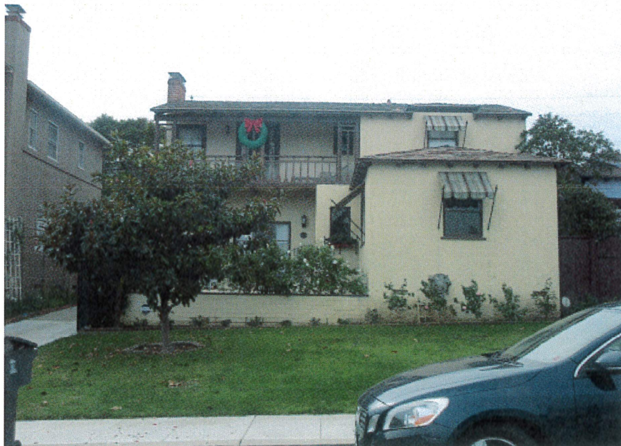
Photo 1: Looking southwest at the primary facade.
