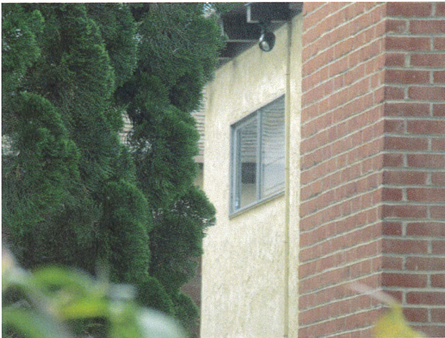
Photo 2: Detail photo showing the heavy textured restucco exterior finish.
