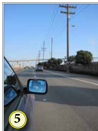
5 The northern segments with asphalt are in fair condition
