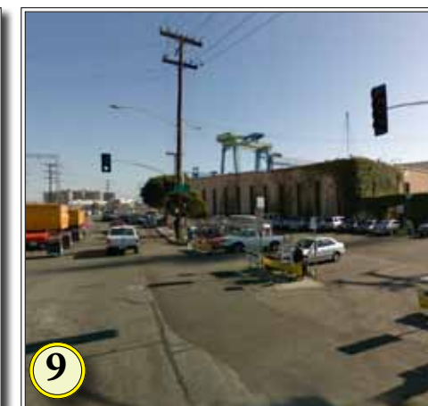
9 Intersections and road edges are poorly defined
