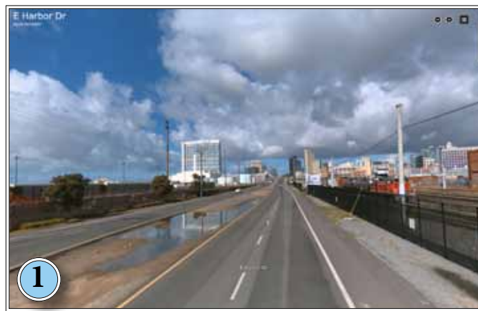
1 Nearly all of the median along Harbor Drive in the study area is devoid of curbs, gutters and storm drains
