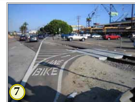
7 The existing rail lines create additional challenges for cyclists
