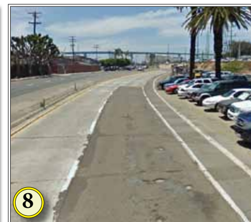
8 Asphalt overlays have been patched numerous times, creating an even more uneven surface
