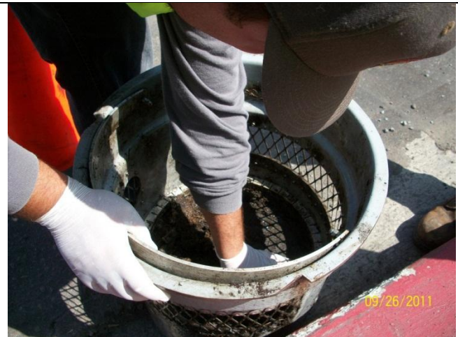
D. Remove DII basket from catch basin, remove soiled filter media
