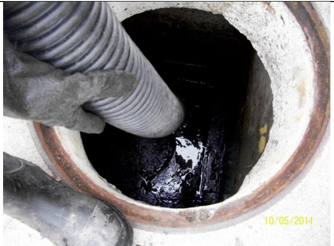
F. Vacuum wash water off of catch basin floor
