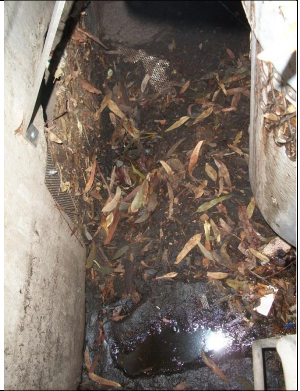
B. Catch basin floor from above
