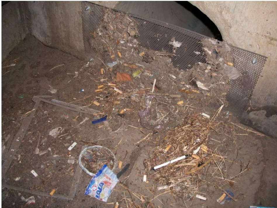
Figure 3-6. Outlet Pipe Screen Installed at Downstream Services BEY-1
