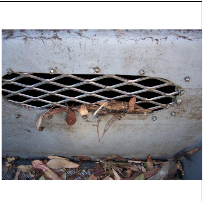
D. Overflow mesh from inside grate inlet basket
