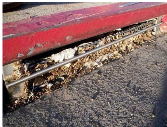
d) Post-storm inspection- Accumulation of gross solids and debris on front of ARS.
