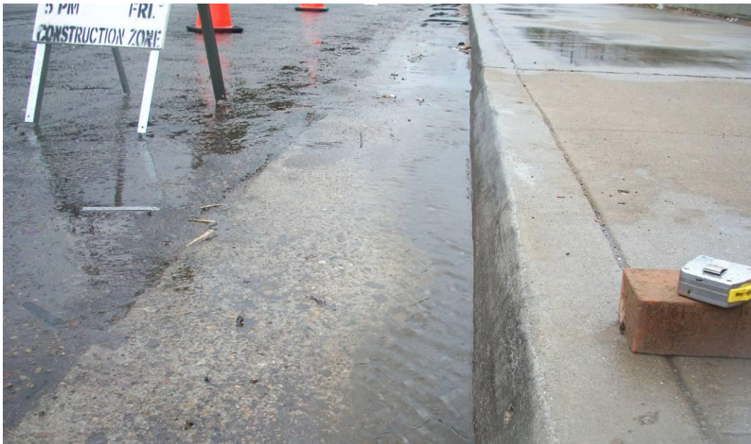
Figure 3-8. Flow Measurement Path at Downstream Services Site BEY-1
