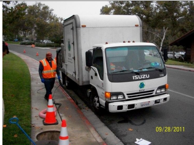
A. Park vac truck, close shoulder, open manhole
