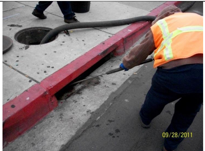
D. Pressure wash DII basket, vacuum wash water
