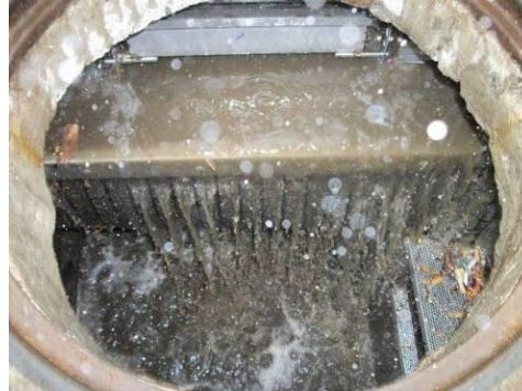
b) Initial point of flow bypass- View down manhole of basket.
