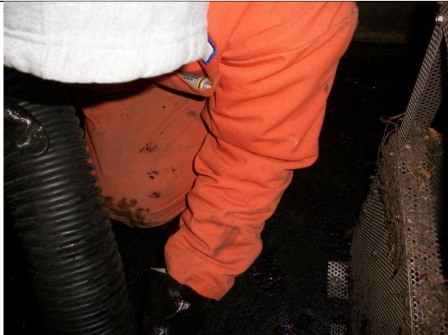
C. Vacuum gross solids off of CPS and catch basin floor
