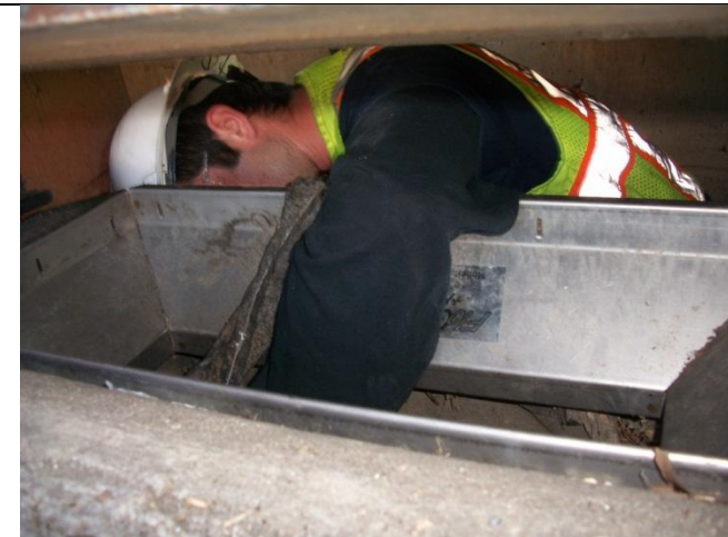
D. Manually agitate settled, compacted solids on fabric
