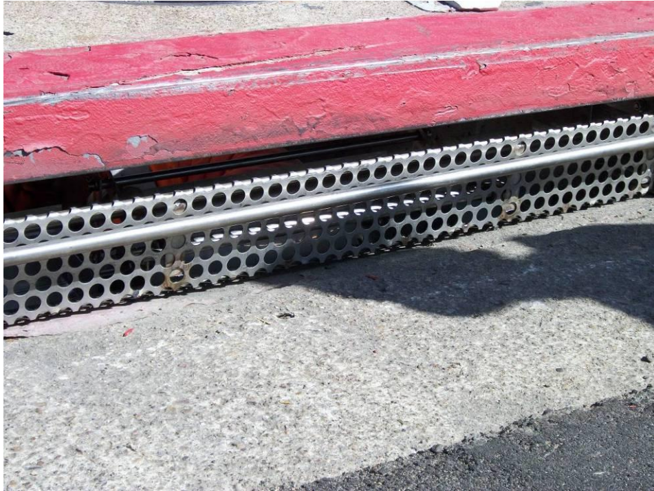
Figure 2-25. United Storm Water Drain Pac Curb Inlet Basket Installed at ECB-F Location
