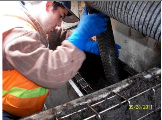
B. Vacuum gross solids out of DII baskets
