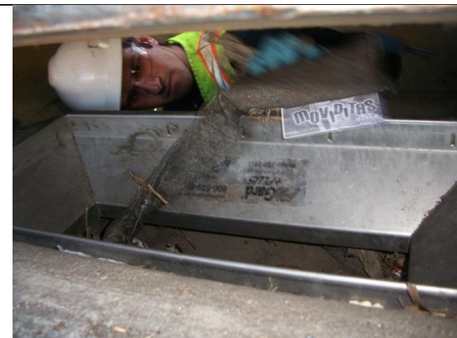
F. Remove and replace soiled media packets
