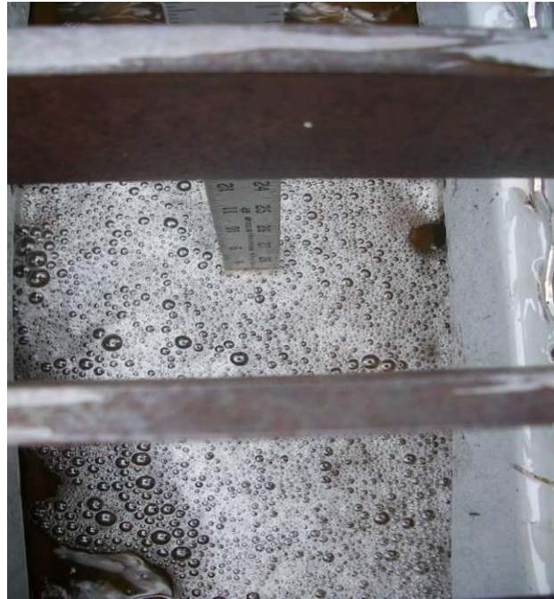
b) Flow bypass continued intermittently; depth of water in BMP shown.
