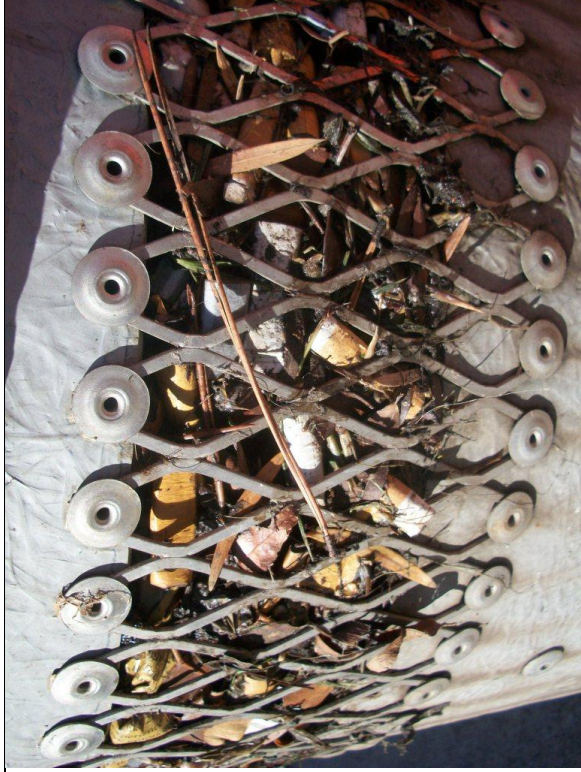
C. Curb inlet basket overflow mesh from rear
