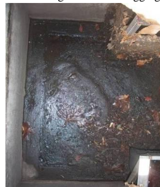
f) Post-storm inspection- Gross solids in bottom of catch basin.
