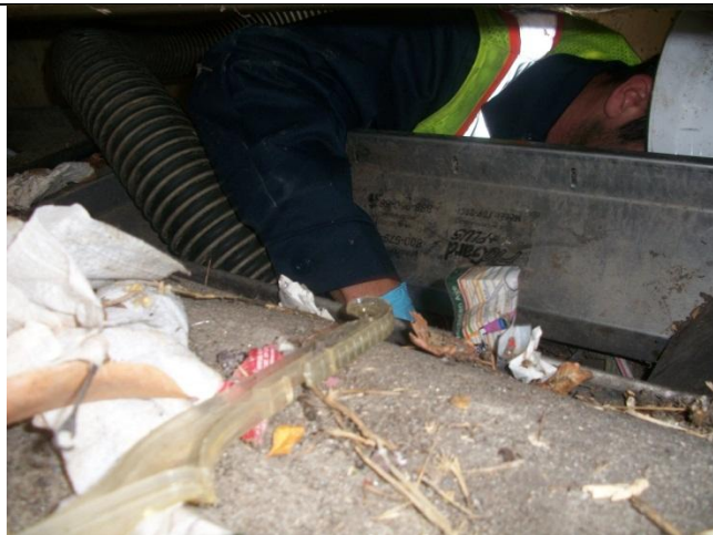
C. Vacuum gross solids out of DII baskets
