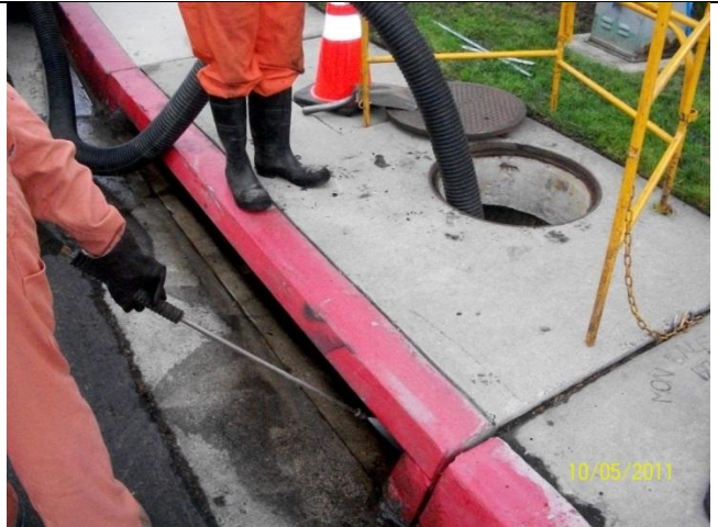
D. Pressure wash DII baskets, vacuum wash water
