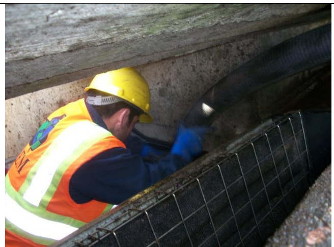
F. Vacuum loosened solids from DII fabric and media
