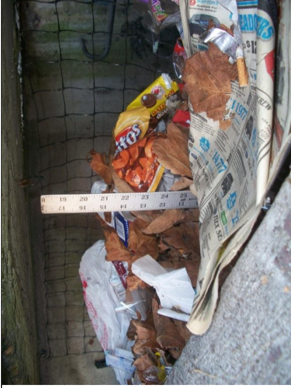
B. Curb inlet basket and storm web from street
