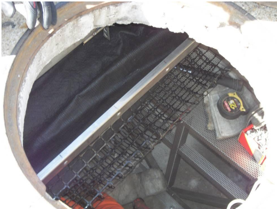
Figure 2-25. United Storm Water Drain Pac Curb Inlet Basket Installed at ECB-F Location
