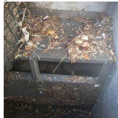
d) Post-storm inspection- Accumulation of gross solids and debris on front of ARS.
