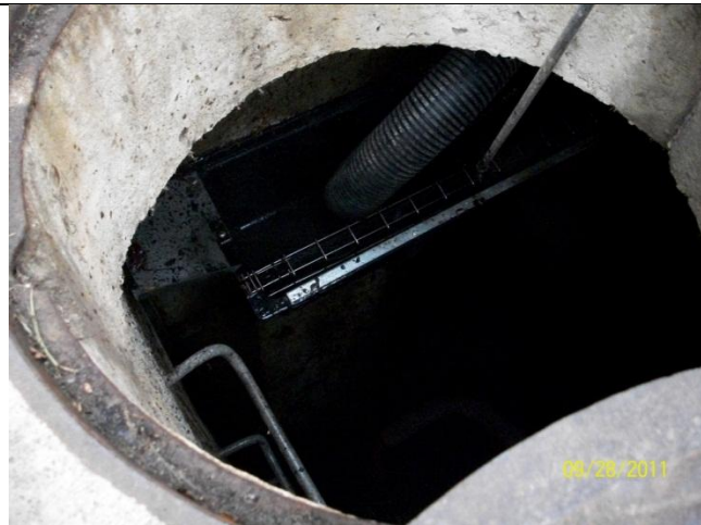
C. Pressure wash DII media, vacuum wash water
