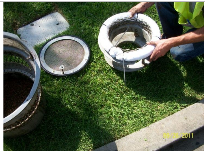
F. Replace soiled adsorbent boom and filter media, reassemble DII basket
