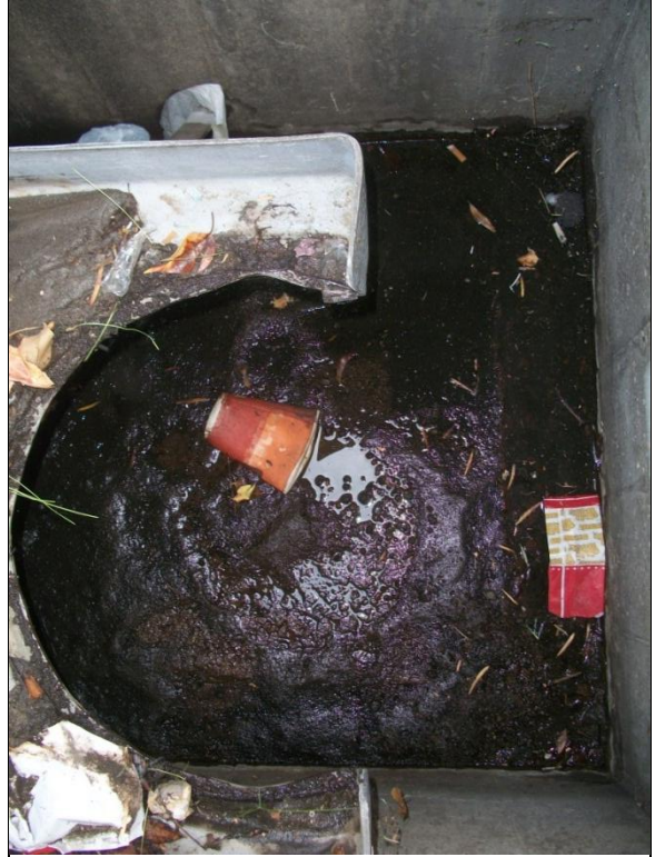
B. Curb inlet basket and media boom from above
