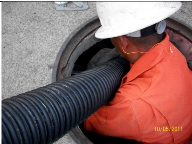
C. Vacuum gross solids out of DII basket, catch basin, and off of CPS
