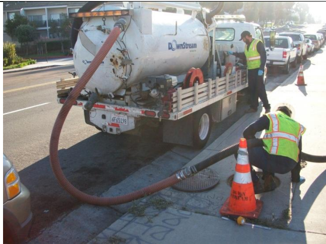
A. Park vac truck, stage tools, open manhole
