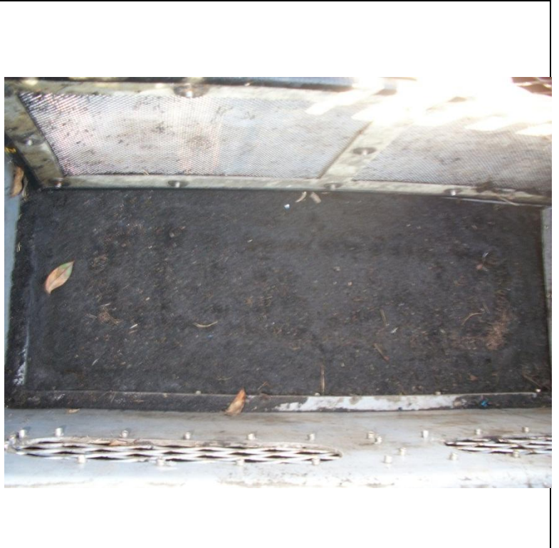
B. Grate inlet basket filter media (beneath screen) from above
