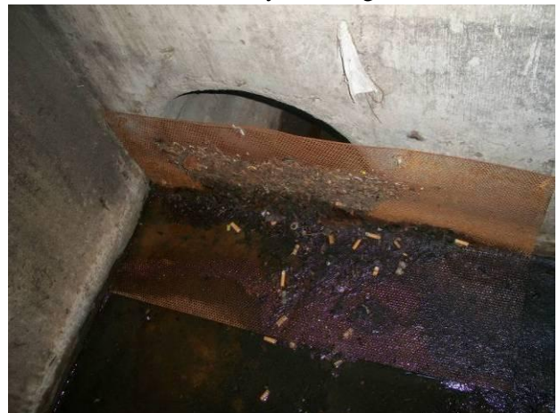
b) Flow bypass of BMP; smaller gross solids are re-suspended and bypass, larger gross solids retained by webbing.
