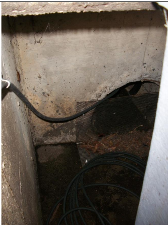
C. Catch basin floor from above, roach at left
