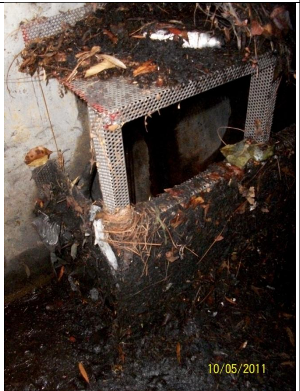
D. CPS from inside catch basin
