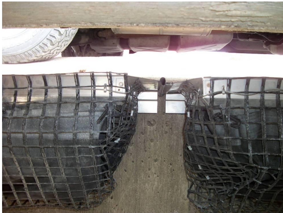
Figure 2-14. Downstream Services FloGard Plus Curb Inlet Filter Installed at BEY-1 Site (View from Catch Basin)
