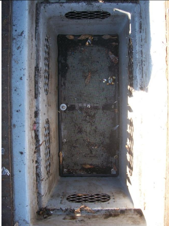
A. Grate inlet basket from above
