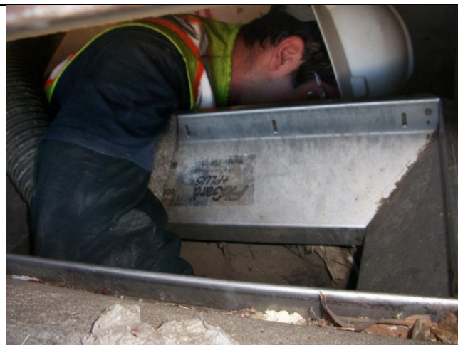
E. Vacuum loosened solids from DII fabric
