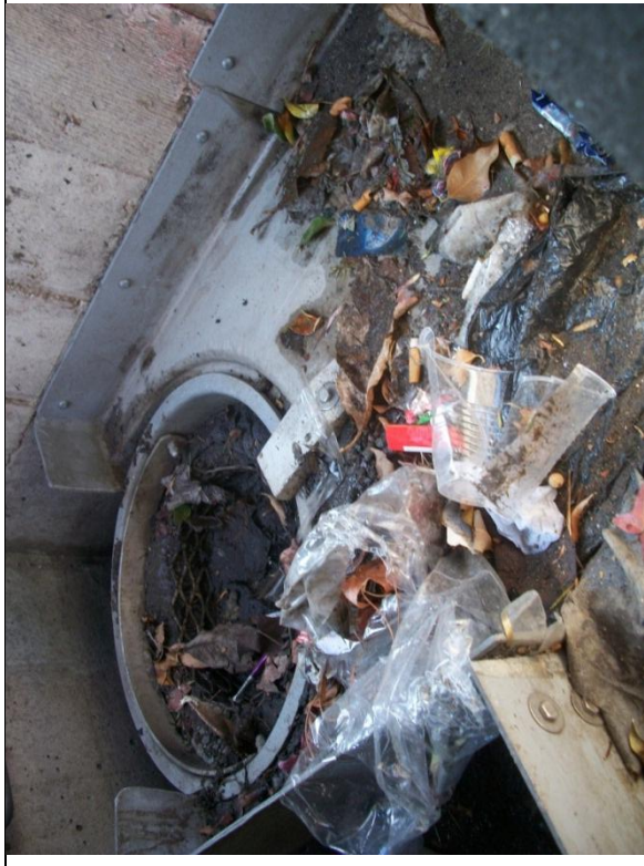
A. Curb insert basket and collection tray from street
