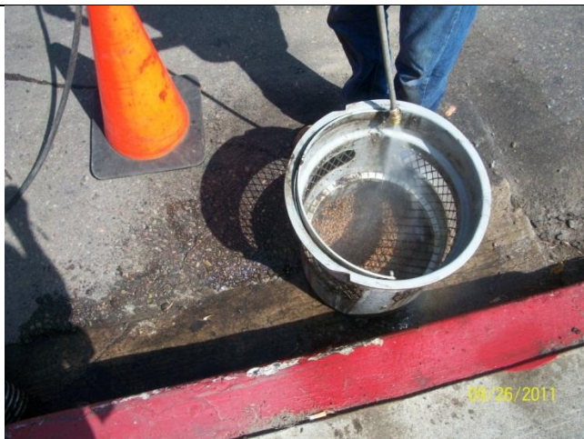
E. Pressure wash DII basket in gutter, vacuum wash water
