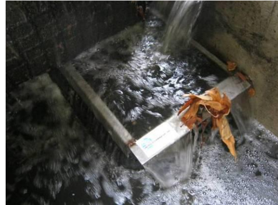
b) Flow bypass of BMP- Lower wing basket below concrete shelf shown.
