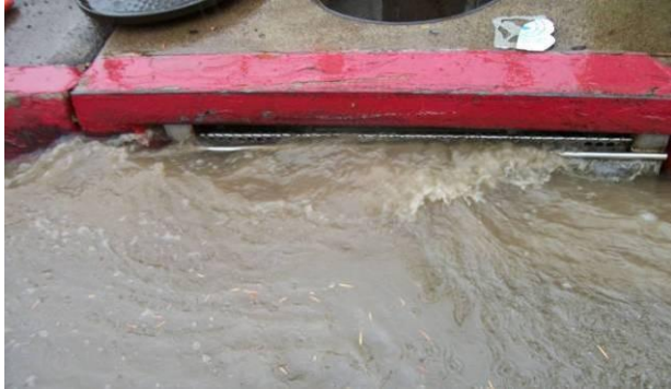
a) ARS remained in closed position for duration of storm event.
