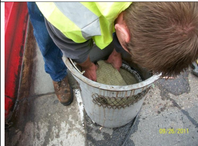
E. Remove and replace soiled filter media
