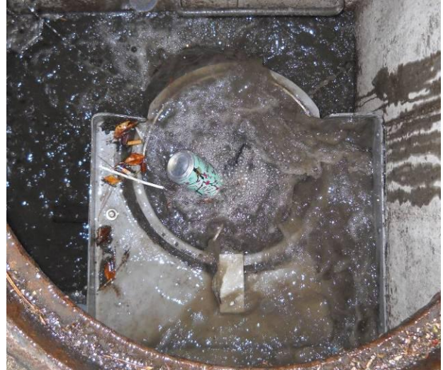
b) Flow bypass of BMP.
