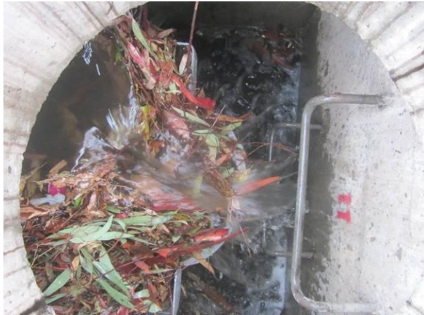
a) Flow bypass of insert product; full of gross solids.
