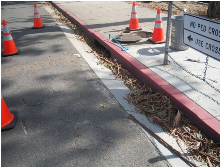
C. Curb gutter, eucalyptus bark
