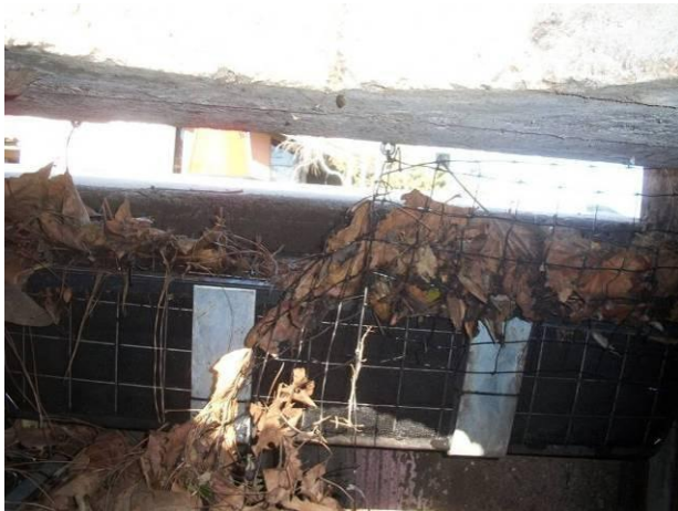
a) At initial point of bypass- View down manhole; product full of water, larger gross solids retained by webbing.
