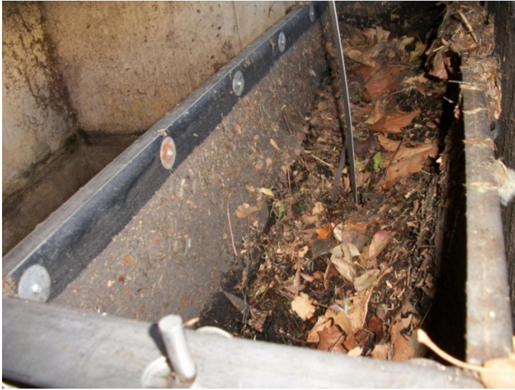
A. Interior of curb inlet basket from side
