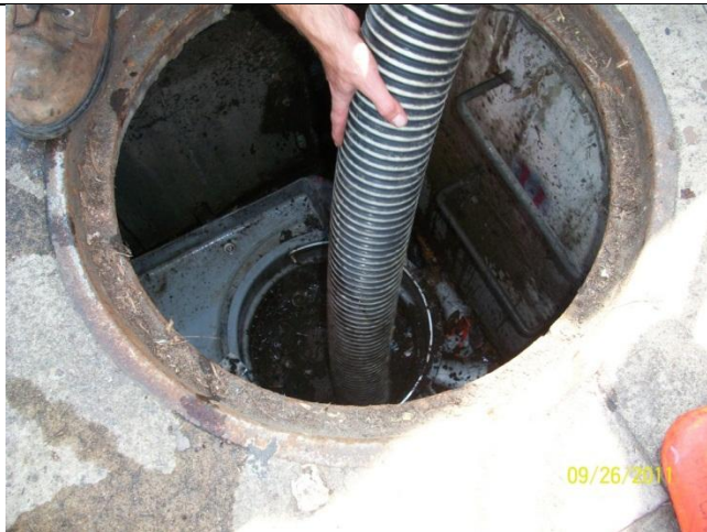
C. Vacuum gross solids and wash water out of DII basket
