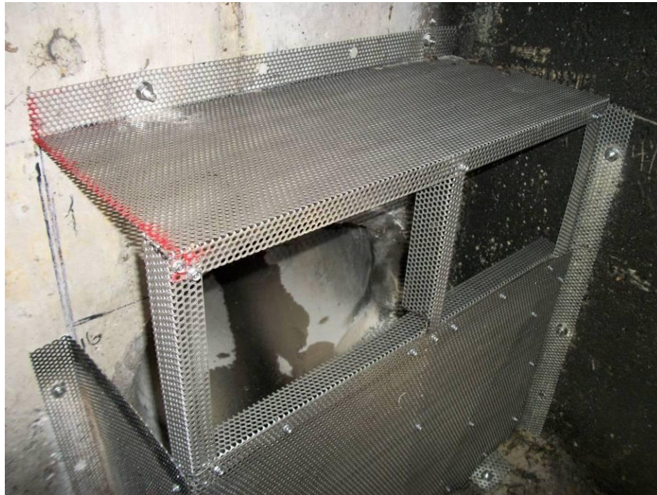
Figure 2-21. United Storm Water Connector Pipe Screen (CPS) Installed at BER-TC Site
