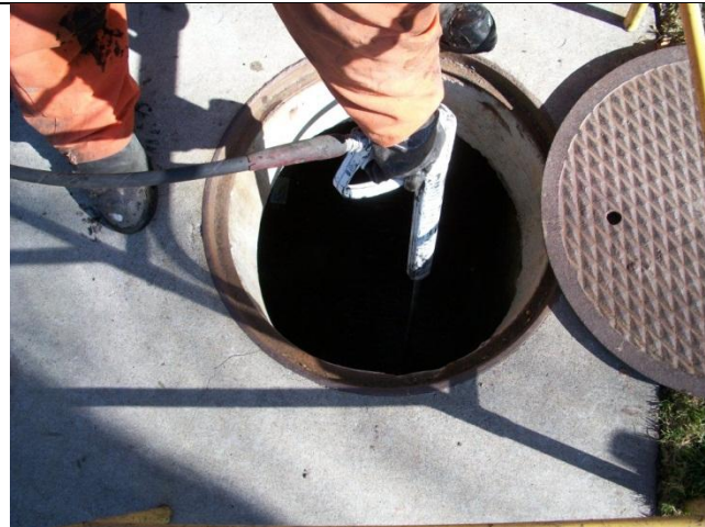
E. Pressure wash CPS and catch basin floor
