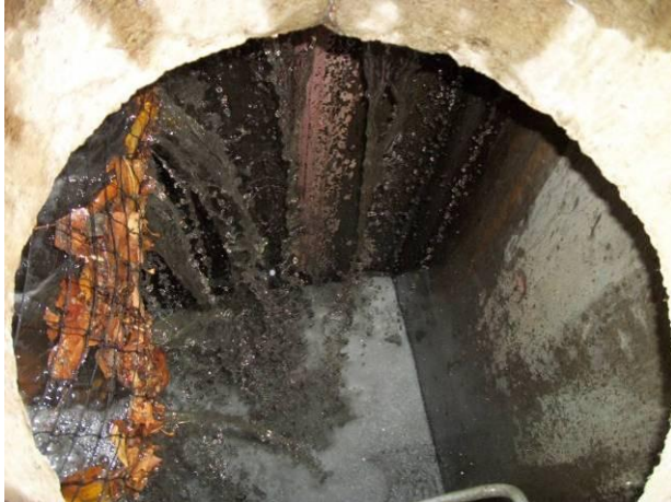
a) At initial point of bypass- View down manhole; product full of water, larger gross solids retained by webbing.
