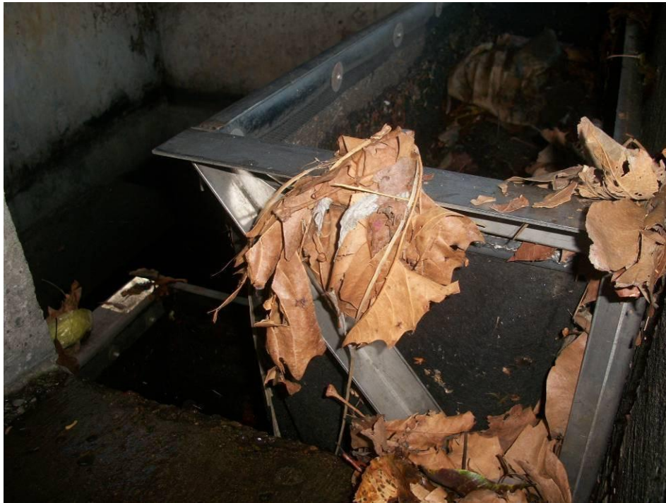
Figure 2-22. Configuration of United Storm Water Drain Pac Curb Inlet Baskets at BER-TC Site
