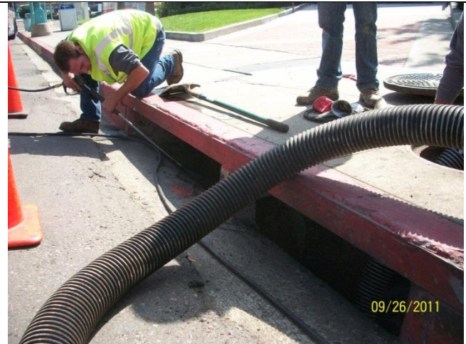
B. Pressure wash collection tray into DII basket
