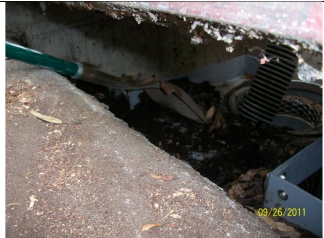
B. Push gross solids on collection tray into DII basket
