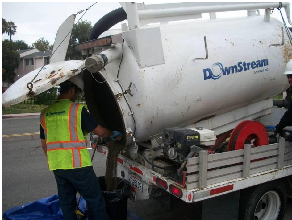
Figure 3-1. Collection of Gross Solids from Vacuum Truck
