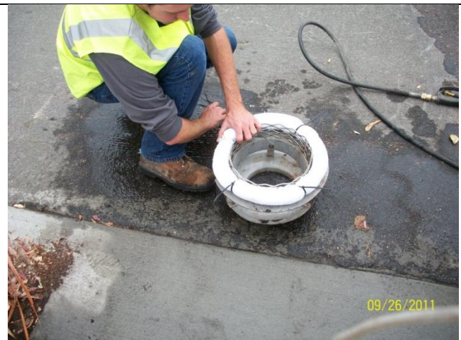
F. Remove and replace soiled adsorbent boom
