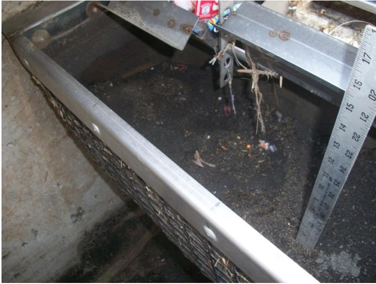
A. Curb inlet basket from above
