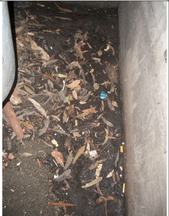
D. Catch basin floor from inside catch basin
