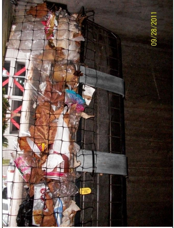
C. Curb inlet basket and storm web from rear
