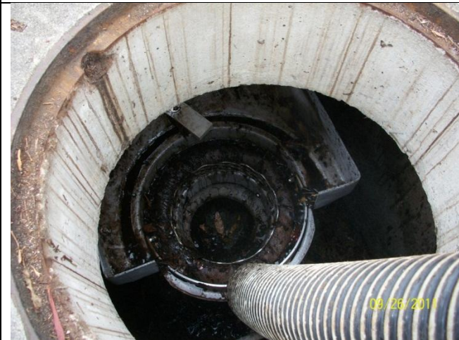
C. Pressure wash collection tray, vacuum gross solids and wash water out of DII basket
