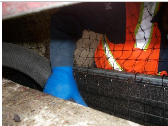
E. Vacuum loosened solids from DII fabric and media
