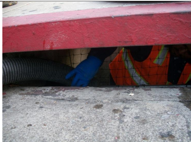
C. Vacuum gross solids out of DII basket
