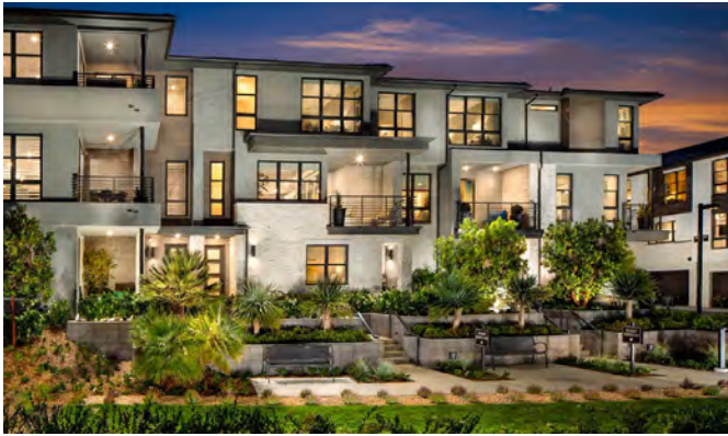
The Heights at Promontory by The New Home Company at Civita, Mission Valley
