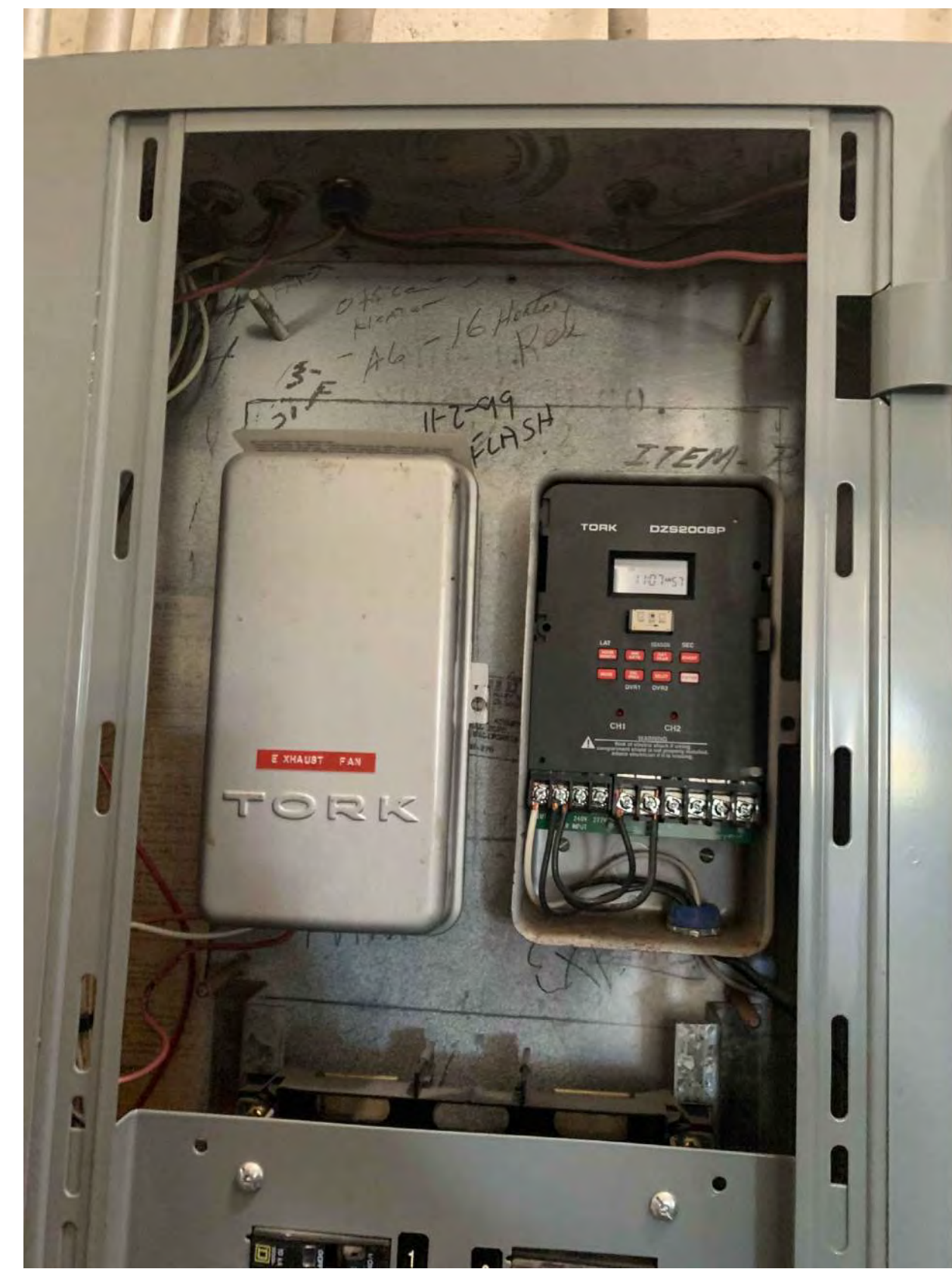
EXISTING PANEL HP1 LIGHTING CONTROLS
