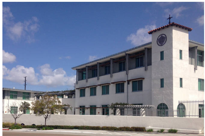
St. Augustine High School has occupied its current location in the community since 1923.
