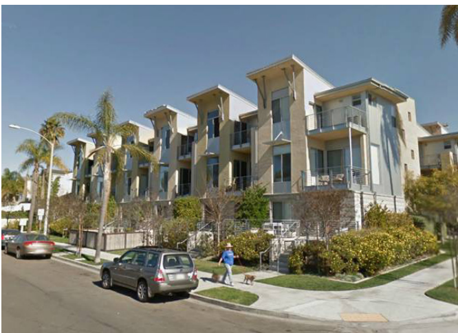
Medium density row home development along Hamilton Street.
