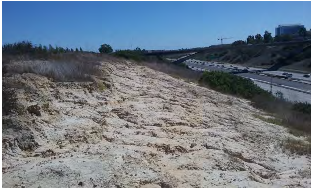
I-805 Slope Looking South
