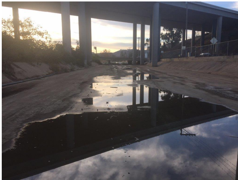
Photo 4. Sorrento Valley Reach 3 (Soledad Creek Channel) (MMP Map 11&12) Maintenance Project, Post-maintenance, 11/13/2016
