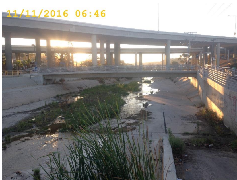
Photo 3. Sorrento Valley Reach 3 (Soledad Creek Channel) (MMP Map 11&12) Maintenance Project, Pre-maintenance, 11/11/2016
