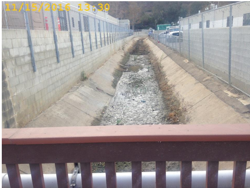
Photo 5. Sorrento Valley Reach 7 (Flintkote Channel) (MMP Map 9) Maintenance Project, Pre-maintenance, 11/15/2016
