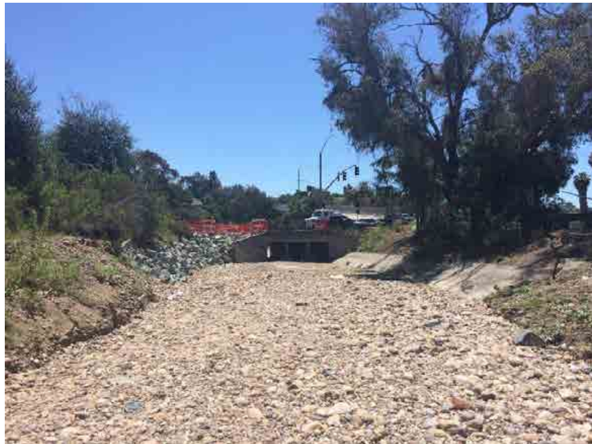
Photo 12. Auburn Creek Channel (MMP Map 77) Post-Maintenance 4/18/16
