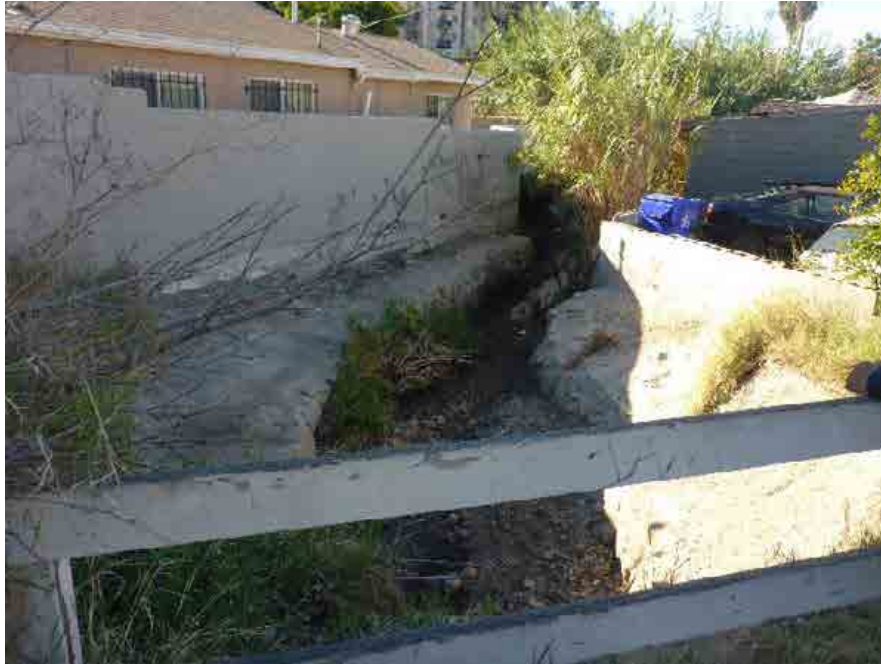
Photo 7. Auburn Creek Channel (MMP Maps 67 & 68) Pre-Maintenance 11/11/15
