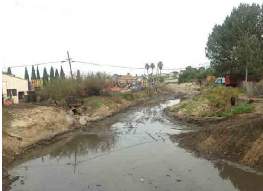
Photo 18. Chollas Creek Channel (MMP Map 93) Post-Maintenance 01/18/16
