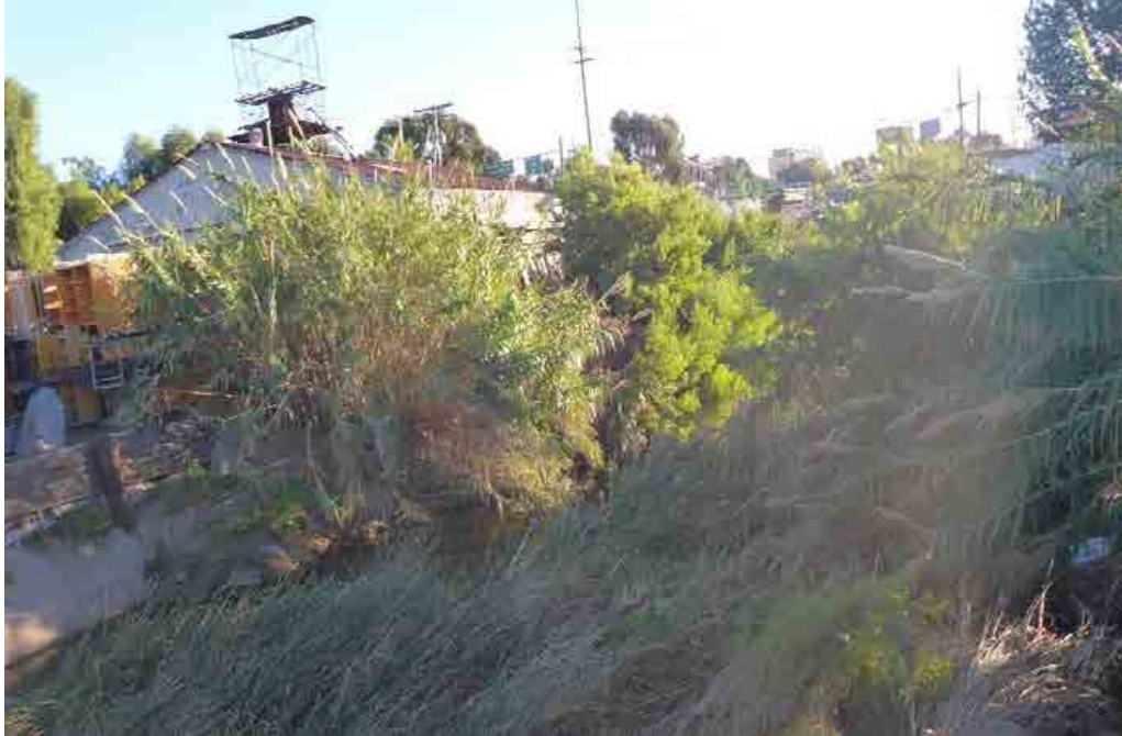
Photo 15. Chollas Creek Channel (MMP Map 91) Pre-Maintenance 12/2/15
