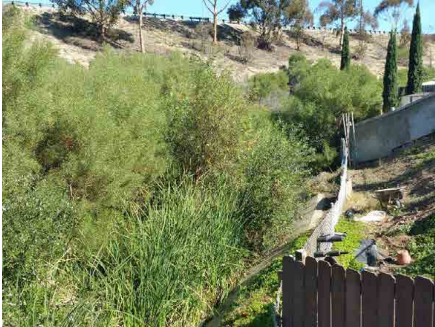
Photo 13. Via de la Bandola Channel (MMP Map 130a) Pre-Maintenance 11/5/15
