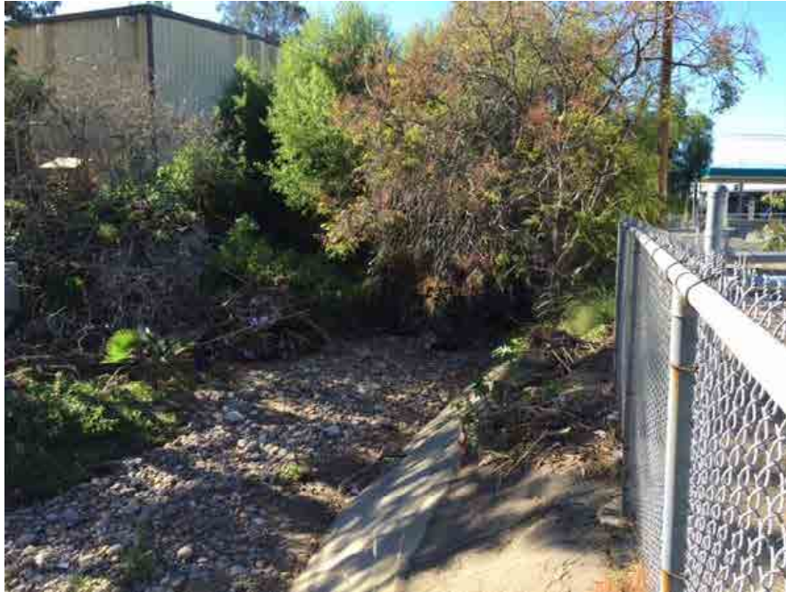
Photo 9. Auburn Creek Channel (MMP Map 70) Pre-Maintenance 11/11/15
