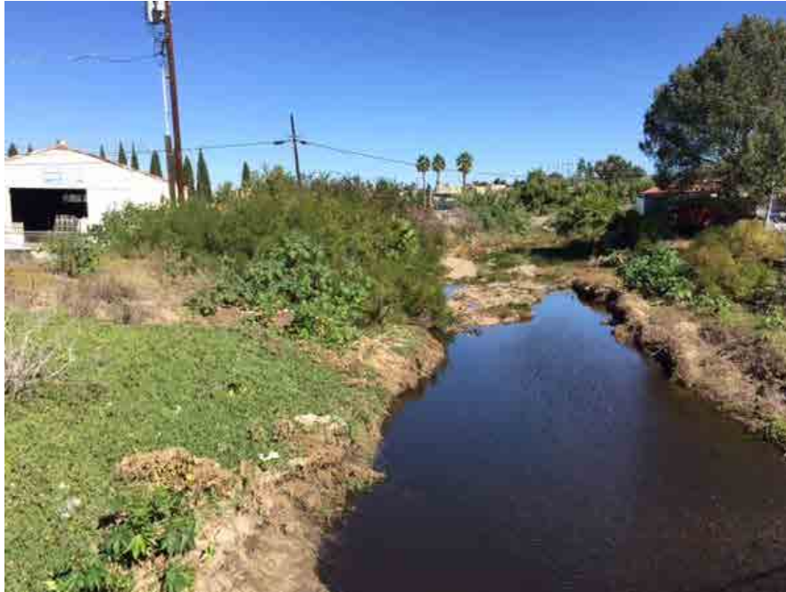
Photo 17. Chollas Creek Channel (MMP Map 93) Pre-Maintenance 11/12/15
