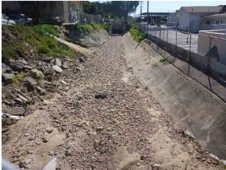
Photo 10. Auburn Creek Channel (MMP Map 70) Post-Maintenance 3/24/16
