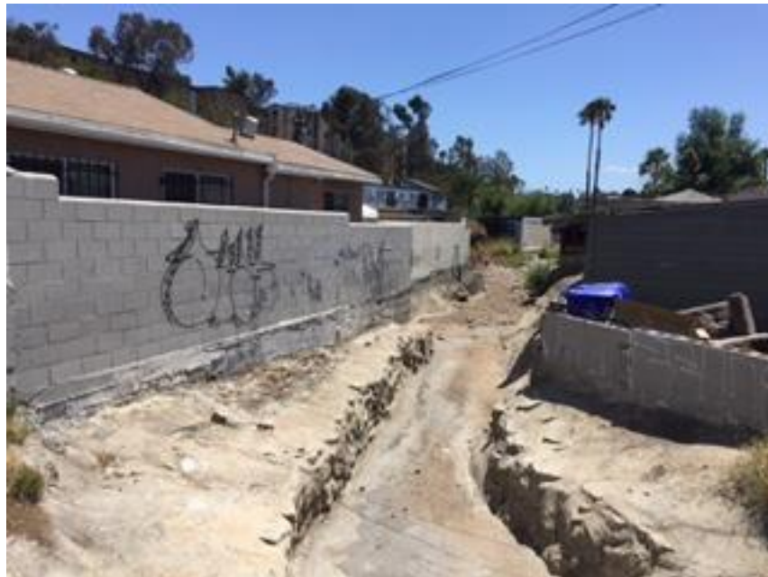
Photo 8. Auburn Creek Channel (MMP Maps 67 & 68) Post-Maintenance 06/13/16
