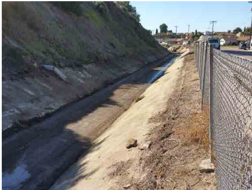
Photo 26. Parkside Channel Post-Maintenance 12/26/15
