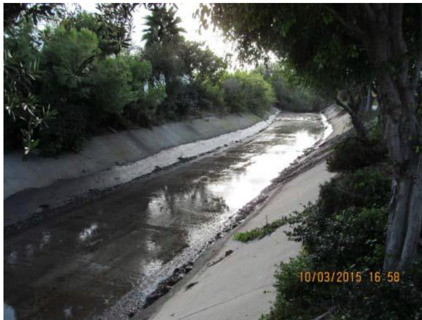
Photo 6. Alvarado Channel (MMP Maps 59, 60, 64) Post-Maintenance 10/03/15
