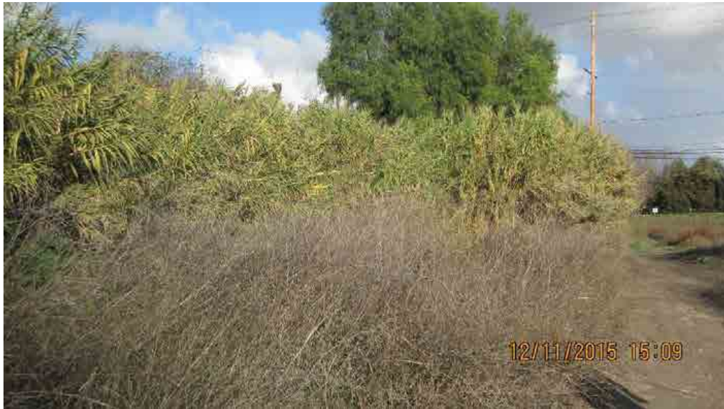
Photo 21. Jamacha Channel (MMP Map 115) Pre-Maintenance 12/11/15
