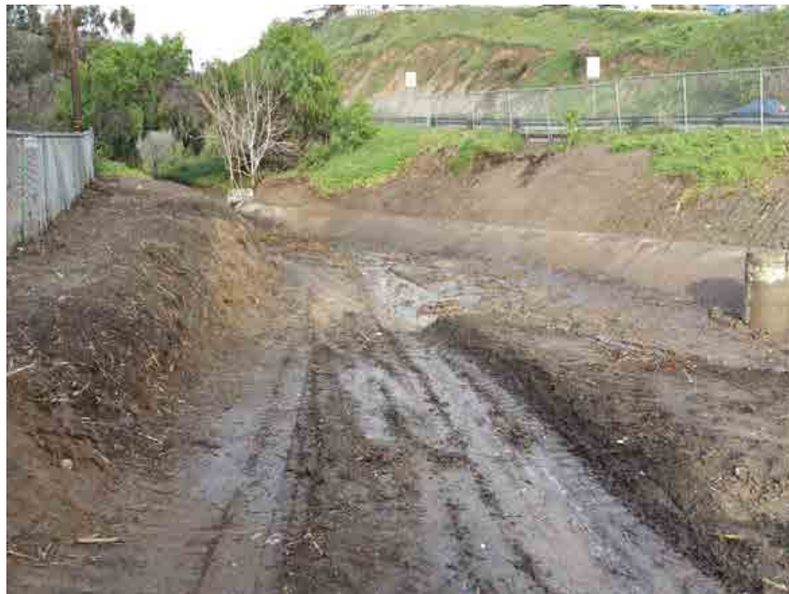
Photo 28. Washington Channel Post-Maintenance 2/1/16
