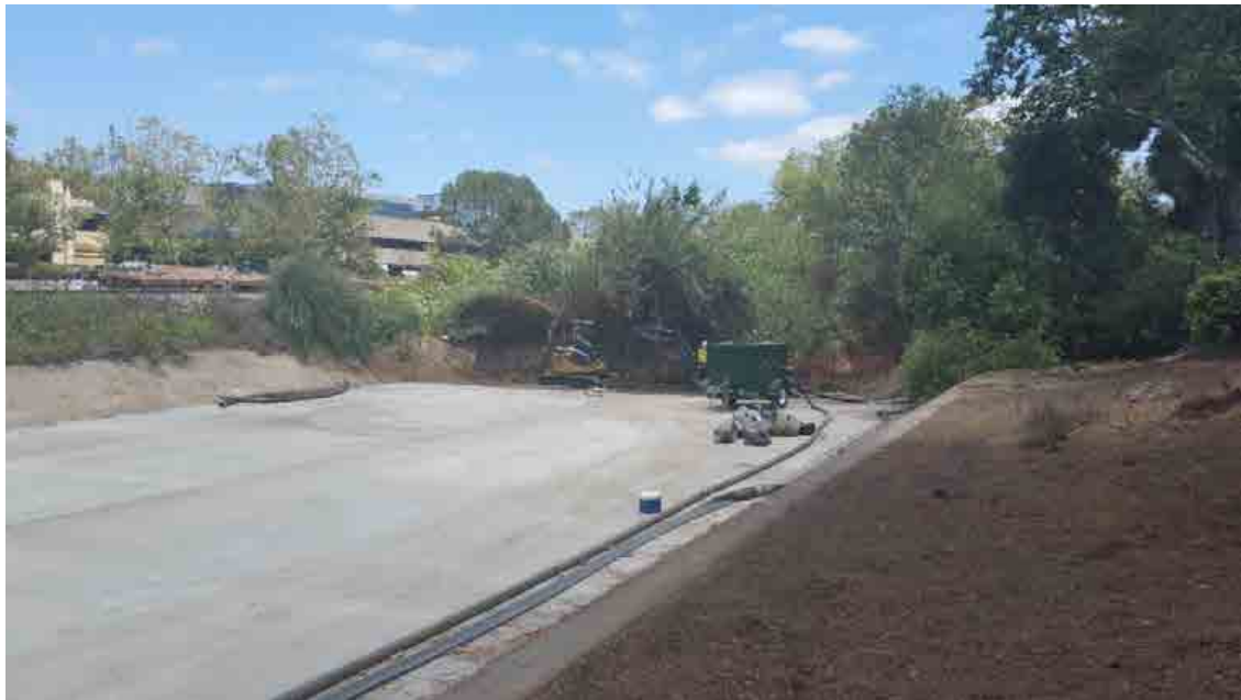
Photo 36. Sorrento Valley (Soledad Creek) Map 12 Emergency Concrete Repair During/ Post-Maintenance 6/13/16
