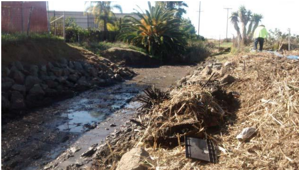
Photo 24. Nestor Creek Channel (MMP Map 134) Post-Maintenance 2/5/16
