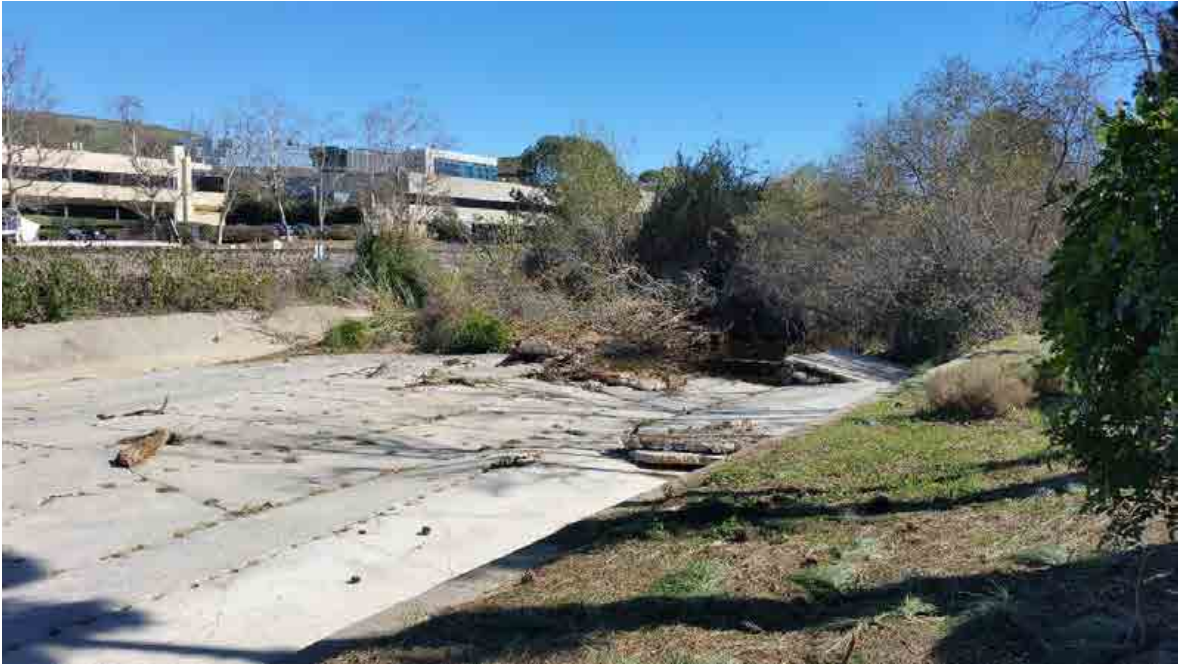
Photo 35. Sorrento Valley (Soledad Creek) Map 12 Emergency Concrete Repair Pre-Maintenance 2/5/16
