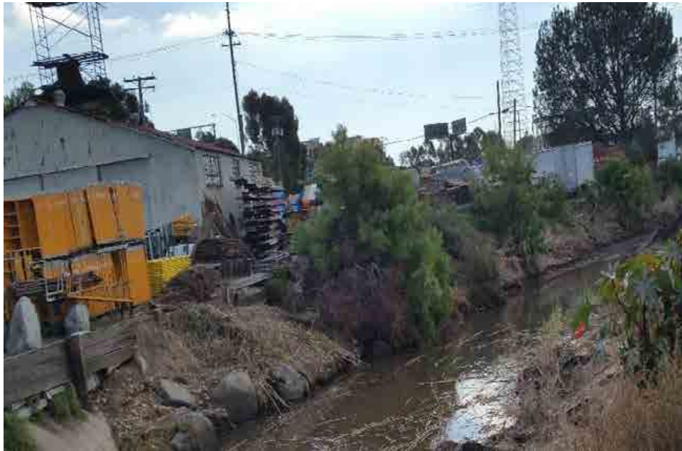
Photo 16. Chollas Creek Channel (MMP Map 91) Post-Maintenance 01/16/16
