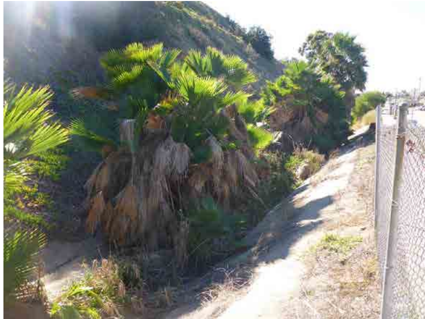
Photo 25. Parkside Channel Pre-Maintenance 12/4/15
