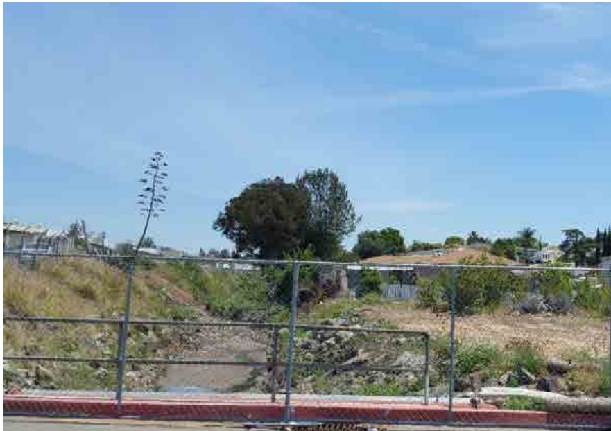
Photo 32. Chollas Creek Channel (MMP Map 71) Post-Maintenance 5/11/16
