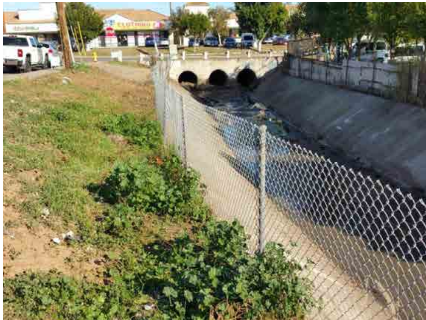
Photo 20. Cottonwood Channel (MMP Maps 120-121) Post-Maintenance 1/1/16
