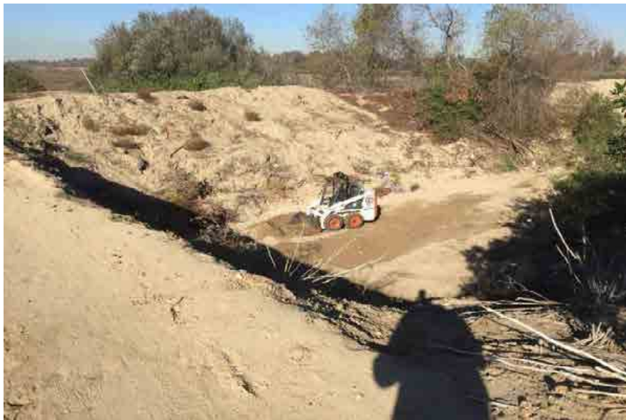
Photo 4. Tijuana River Valley Pilot Channel and Smuggler's Gulch During Maintenance 12/3/15
