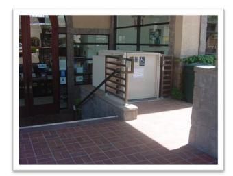
If platform lifts are provided, they shall not be attendant operated and shall provide unassisted entry and exit from the lift.
