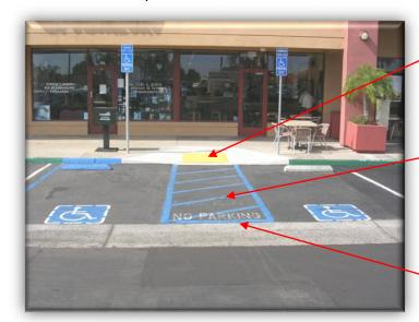
There must be a detectable warning at entry onto the vehicular way.
