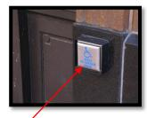
Where doors do not comply with the maximum opening force or the required distance past the strike edge, a power assisted push button may be considered an acceptable means of equivalent facilitation by the building official.
