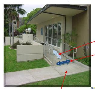
Running slope shall not be steeper than 1:12 (8.33%).
