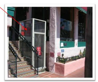
Elevators may be provided as an accessible component along accessible route of travel in an existing building or facility, to provide access where existing site constraints or other constraints make use of a ramp technically infeasible.
