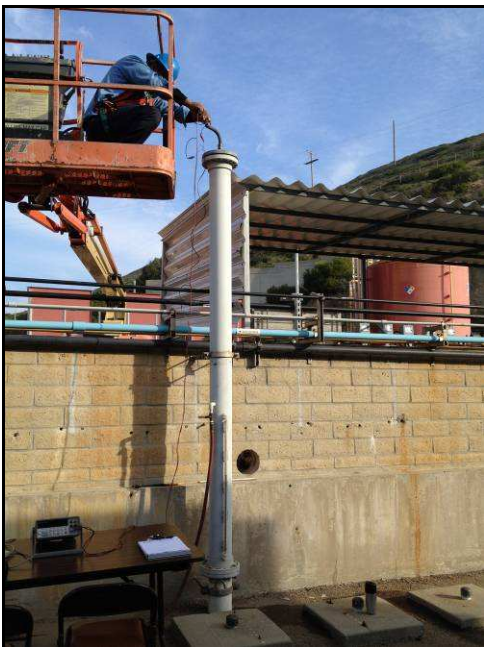
Photo 4-4: Transducer is Inserted Into Static Water Well for Testing
