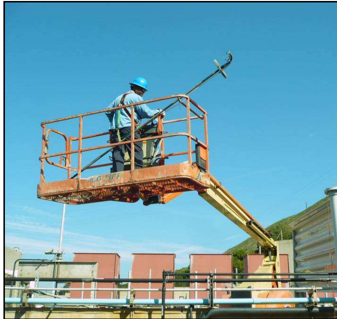
Photo 4-3: Transducer Being Moved to Testing Well
