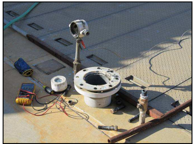
Photo 4-2: Flume Access After Transducer Has Been Removed
