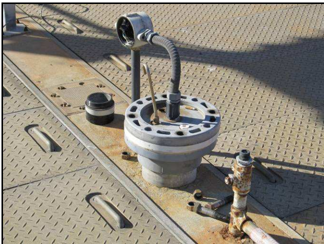
Photo 4-1: Gould Transducer in Operational Configuration
