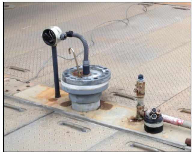
Photo 4-2: Gould Transducer in Operational Configuration
