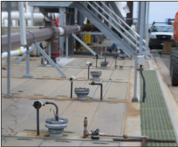
Photo 4-1: Topside View of the Four Partial Flumes
