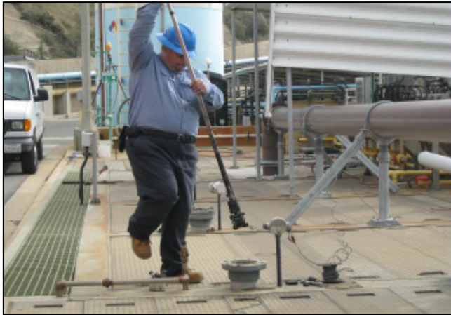
Photo 4-3: Transducer is Removed From Flume
