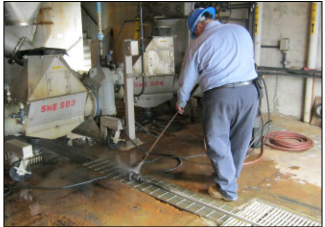
Photo 4-4: Transducer is Cleaned
