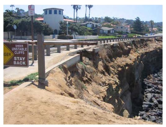
Photo 8 - Top of Bluffs, showing damage to curb, Site 7.
