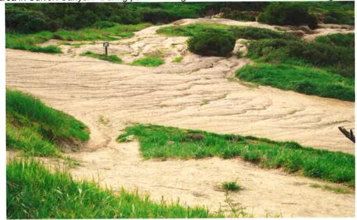
Figure 21. Erosion rills cause by runoff from the Loop Road, predominantly from the 24" pipe.
