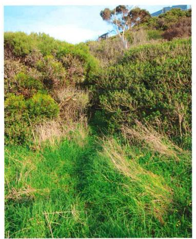
**Figure 10**. Runoff from the 18" drain goes over the edge of the Loop Road where the curb is 3" or less in height, and it then flows under the bushes and follows the "trail" down the hill, shown by laid down weeds.
