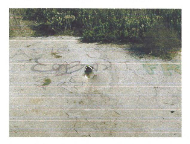
**Recommendation:** Flows from this outfall should be directed into the Hillside Park drainage system for ocean disposal of runoff along with runoff from: Drainage Basin M2, Young Hall Parking lots, and other drainage basins and locations in the Park.
