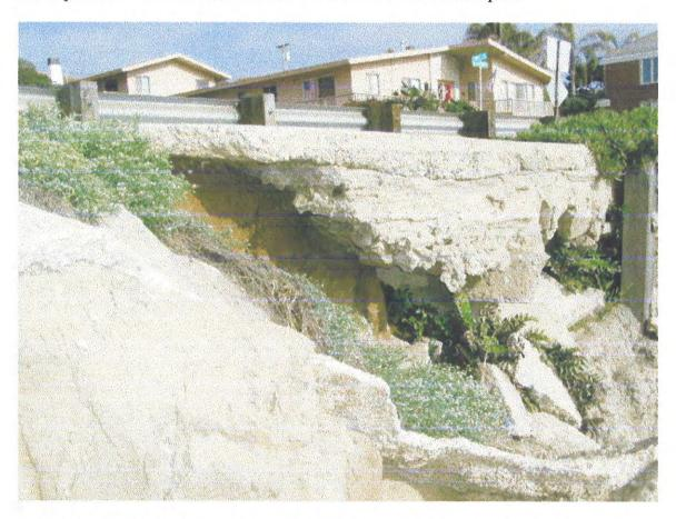
**Recommendations:** Rick Engineering recommends a major upgrade of the drainage system that discharges over the cliff at Location 9 that would include the replacement of four sections of pipe totaling 730 feet in length. This upgrade needs to be implemented in order to protect the cliffs from further erosion, and prevent Sunset Cliffs Boulevard from being undermined.
