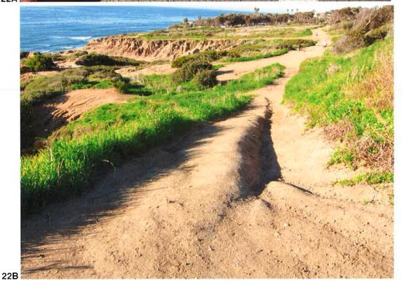
**Figure 22A & 22B.** Low curbs transition to 6" high curbs where the ramp from the sludge line trail joins the Loop Road (Figure 22A). The low curbs enable road runoff, made up in large part by discharges from the 24" pipe, to flow down the transition trail (Figure 22B) and into Culvert Canyon where it contributes to
