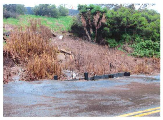
**Figure 7.** The 18" pipe discharges on this slope among the concrete rubble and dead Arundo plants. Runoff from the 18" pipe mostly stays on the road until the asphalt curb on the western side of the road decreases from approximately 6" in height to 3" and then is nonexistent.
