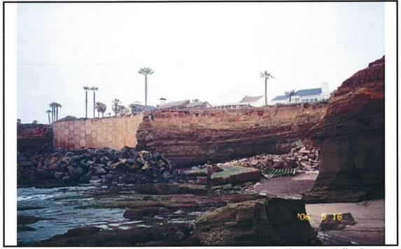
Figure 4B: MSE wall for bluff stabilization along with rip-rap at base near Adiar Street. Terrace deposits of Bay Point Formation seen overlying Point Loma Formation.
