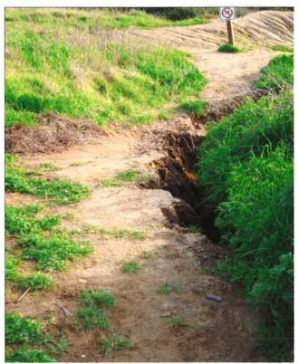
**Figure 14.** This new erosion gully from runoff from the 18" drain coming off the Western Loop Road was first noticed after the major December 2010 storm. The upper, southward running portions of this recently
