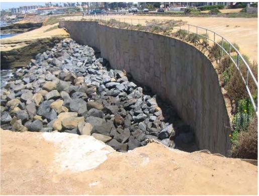
PH24: USACE sea wall/riprap. There was a cove behind it that extended close to the road. The Corps built the wall farther seaward and filled behind it. The fill appears to be quarry rock and dirt. Dedi would prefer to see this are be used as a parking area, since it is 'man made' and it would be hard to restore this are to natural conditions.
