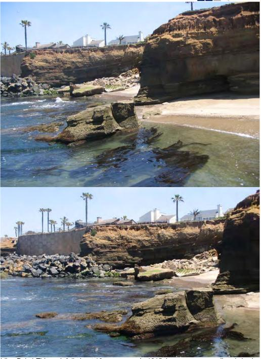
PH25/26: (Spalding Point) This arch fell about 10 years ago. In 1915 there was a seawall and viewing platform. This collapsed because the seawall failed (Dedi suspects that this is indirect erosion caused by the seawall/shore protection scouring around it).
