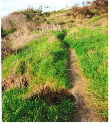
• Figure 12A. Runoff from the 18" pipe is undercutting this trail that is being considered as a secondary trail for the Park, and has caused a significant collapse of the trail and the slope adjacent to it.
