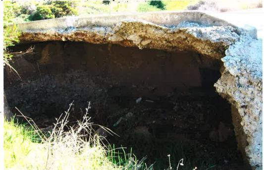
**Figure 25B.** Close up of the undermining of the Loop Road Arizona Crossing. Most of the water causing this damage is from the 24" drain.
