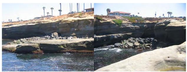
PH10/11: Riprap to fill coves. In 1984, the Corps filled in all the crevices and eroded areas along entire SCB stretch.
