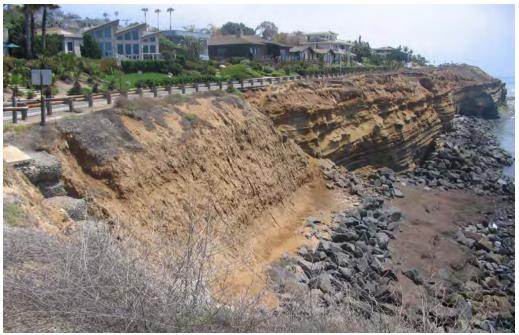
PH35: South of Monaco: No stratification along cliff face; The road was built on cove and filled it with rock and fill.
