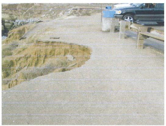
**Recommendation:** Increase the slope of Parking Lot #2 and soil towards Sunset Cliffs Boulevard to maximize the runoff drains away from the ocean. Install curbs and remove impervious paved surfaces and compacted soil where possible, and replace them with vegetation or a trail surface that does not produce erosive runoff.
