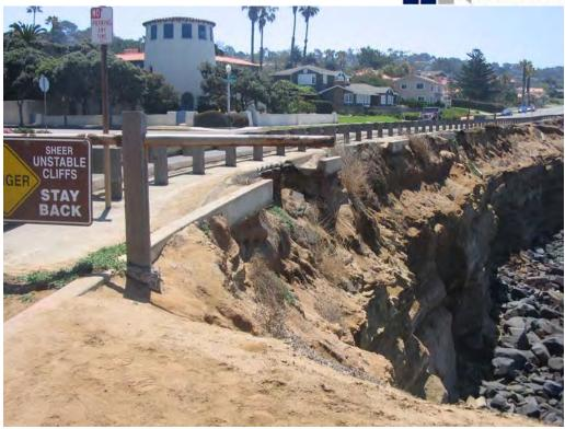
PH4: Bluff Failure caused by 2 caves joining on both sides of bluff protrusion and water impact through these formations.
