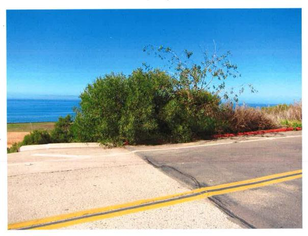
**Figure 24.** Due to low curb height at the northern edge of the Loop Road Arizona Crossing, runoff during moderate to high flow periods tends to flow around the northern edge of the Arizona Crossing apron and undermine it. The black Acacia branches cover the point where the runoff goes off the road.
