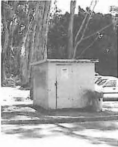
An existing grounds maintenance shed.
