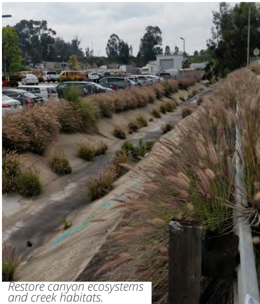
Repair flood damaged areas in trails and construct erosion control.
