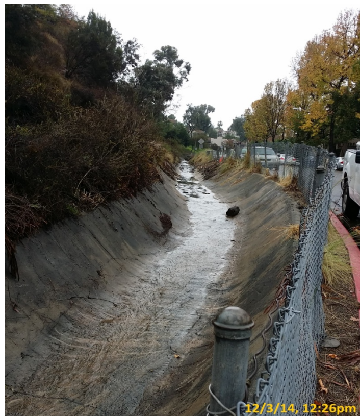
Photo 10: Reservoir Drive Channel Emergency Post-Maintenance 12/3/14
