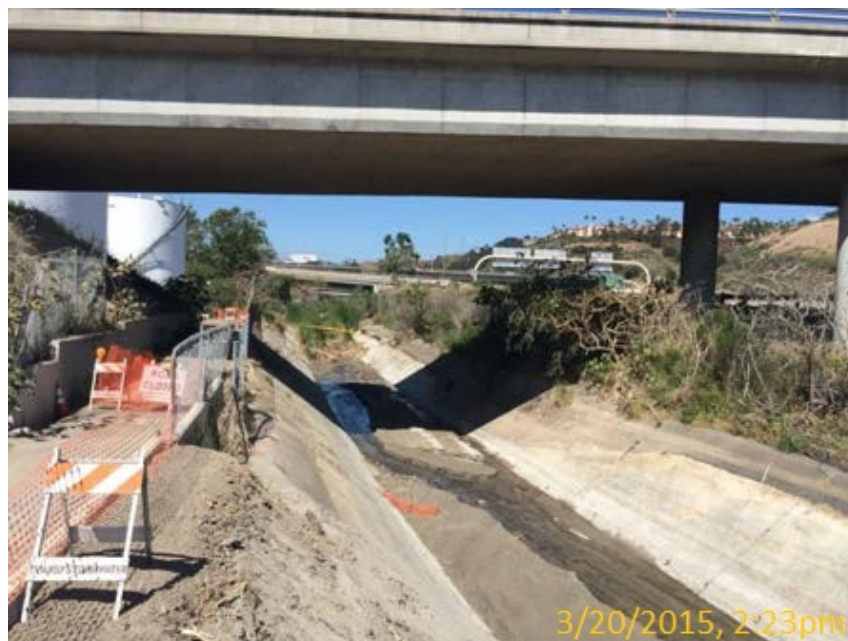
Photo 4. Murphy Canyon Creek Channel Post-Maintenance 3/20/15
