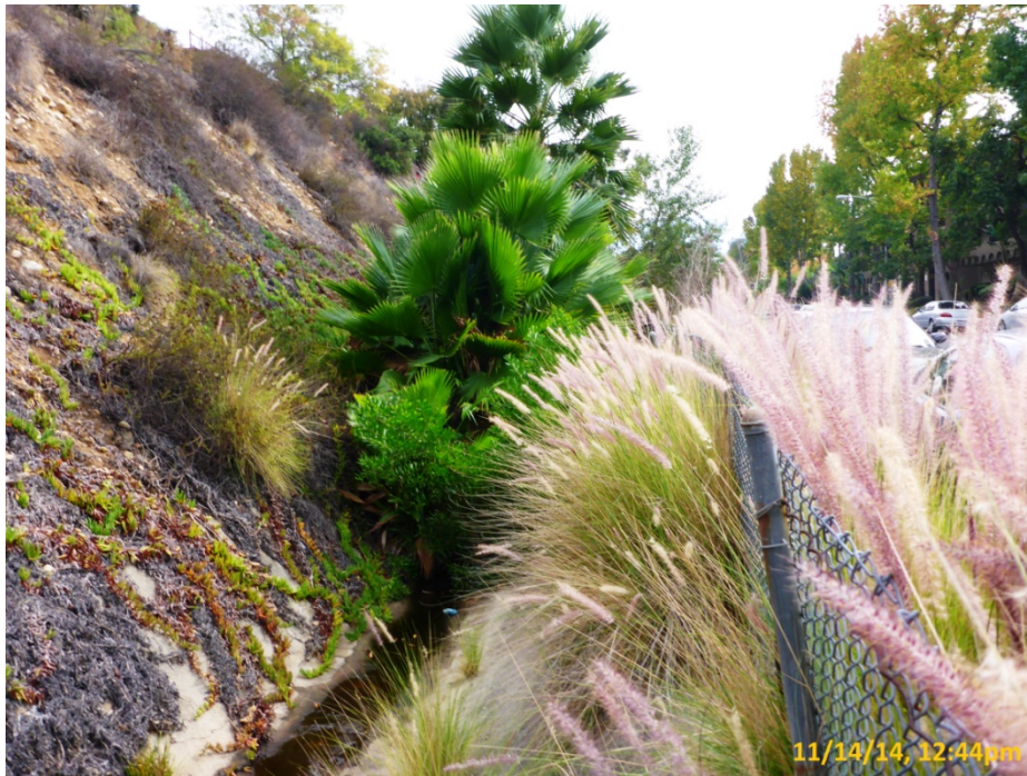
Photo 9: Reservoir Drive Channel Emergency Pre-Maintenance 11/14/14
