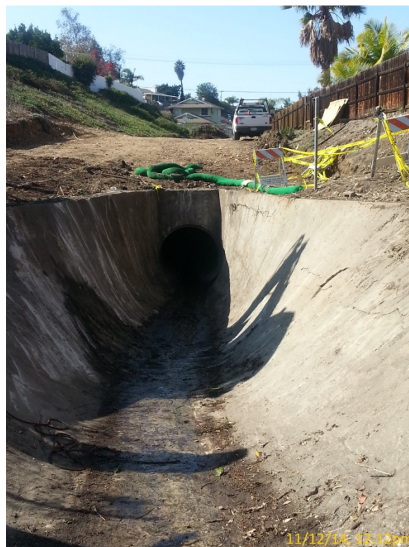
Photo 8: San Carlos Creek Channel Emergency Post-Maintenance 11/12/14
