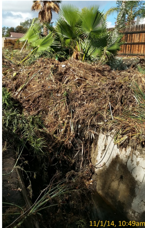
Photo 7: San Carlos Creek Channel Emergency Pre-Maintenance 11/1/14
