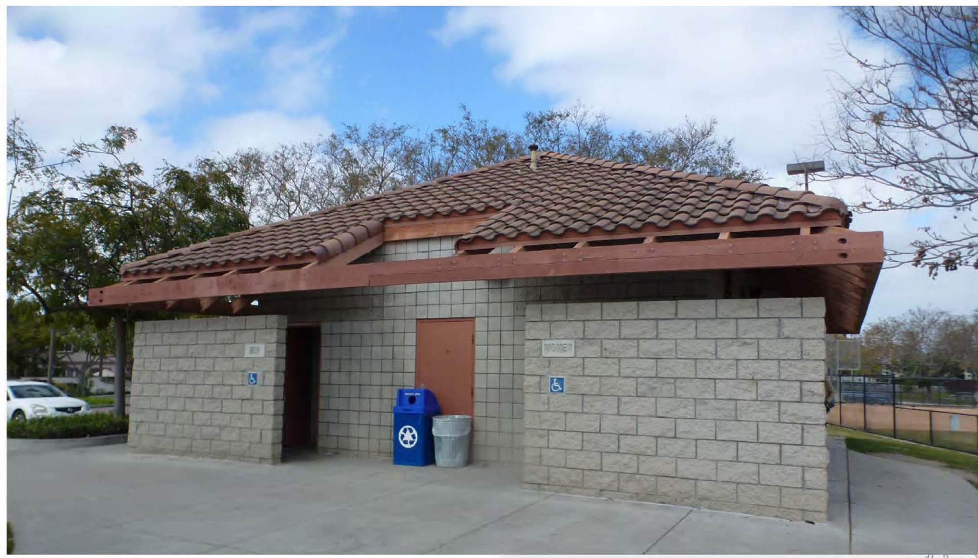
EXISTING RESTROOM BUILDING
