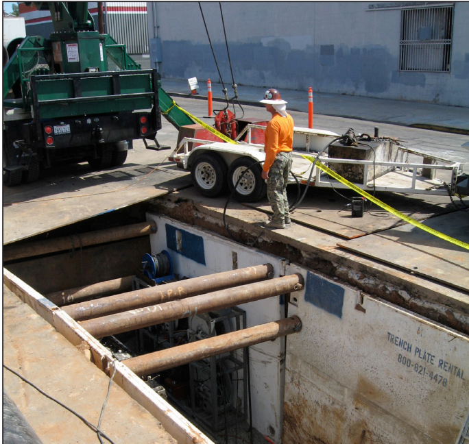
Figure 5: Example of trenching
