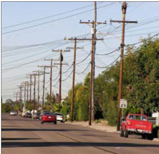
Figure 3: Street with utility poles
