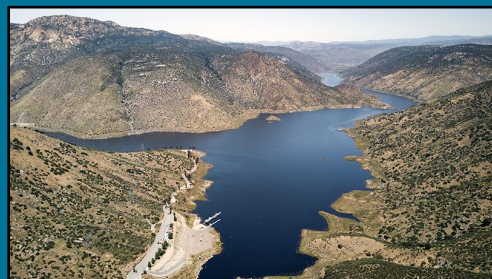
El Capitan Reservoir Courtesy City of San Diego
