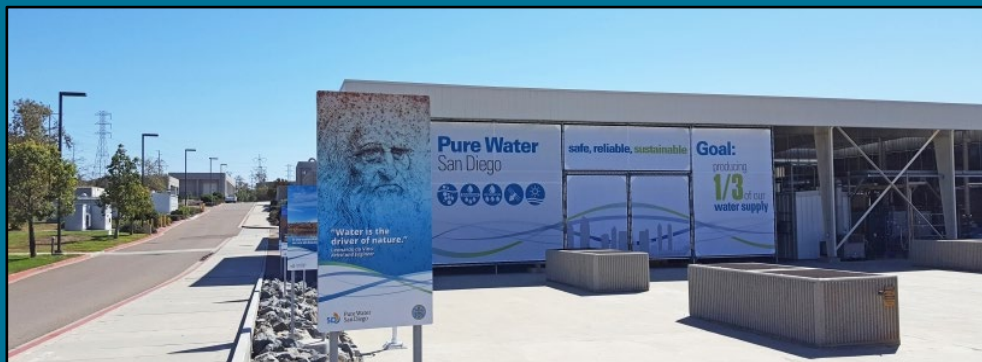
North City Water Reclamation Plant Courtesy City of San Diego
