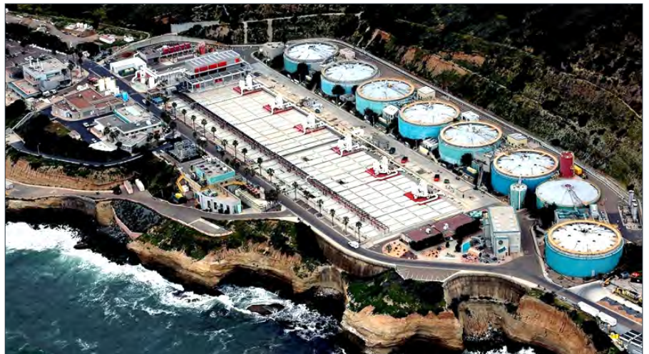
The Point Loma Wastewater Treatment Plant
