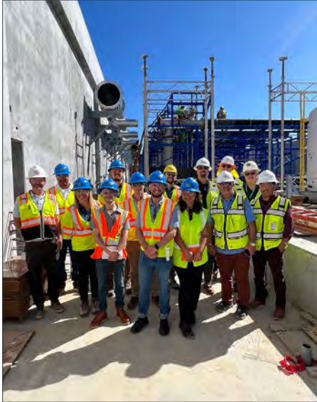
Representatives from offices of Sen. Toni Atkins, Gov. Newsom, Asm. Chris Ward check out the construction progress.
