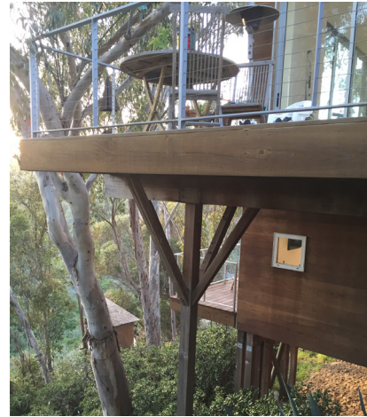
Residential development along hillsides can limit their impact in these areas by using building types such as houses on stilts, which avoid the typical grading associated with flat slab construction.
