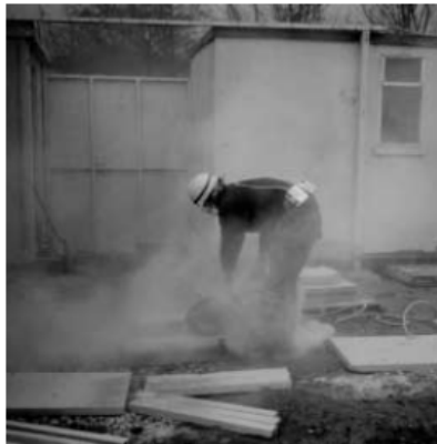
Concrete Cutting Photo Source: Health & Safety Executive (CIS# 54)
