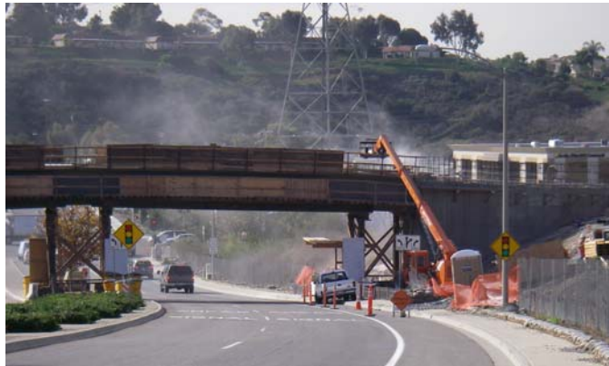
Sandblasting Photo. Source: Weston, 2006.
