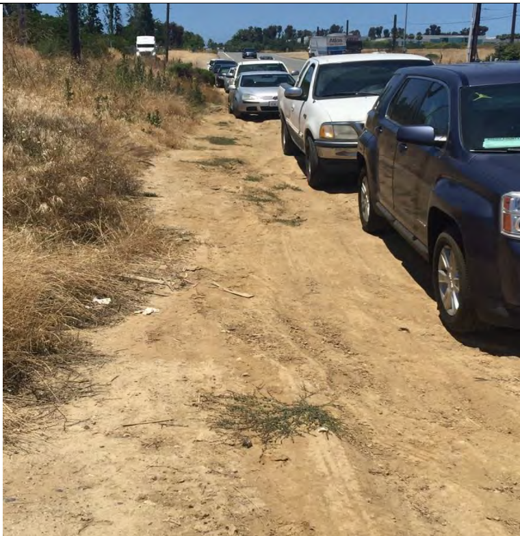
Overview photo of road ruts PWP 3 through PWP 7
