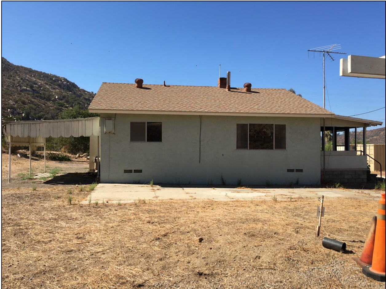
Figure 22. View of the northeast elevation; note the carport addition on the left (south) and the enclosed patio addition on the right (north) (Photo credit: Dudek).
