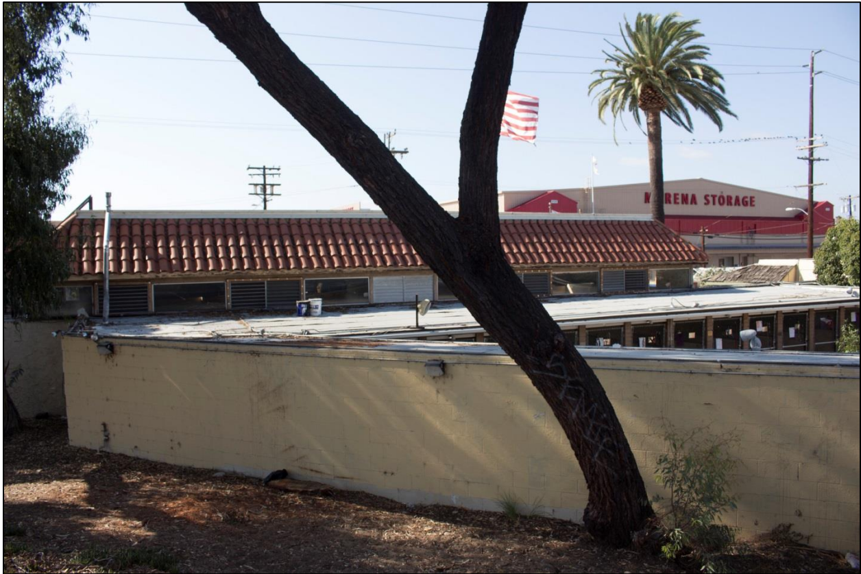
Figure 9. Western portion of southwest elevation; view looking northeast (Photo credit: Dudek).
