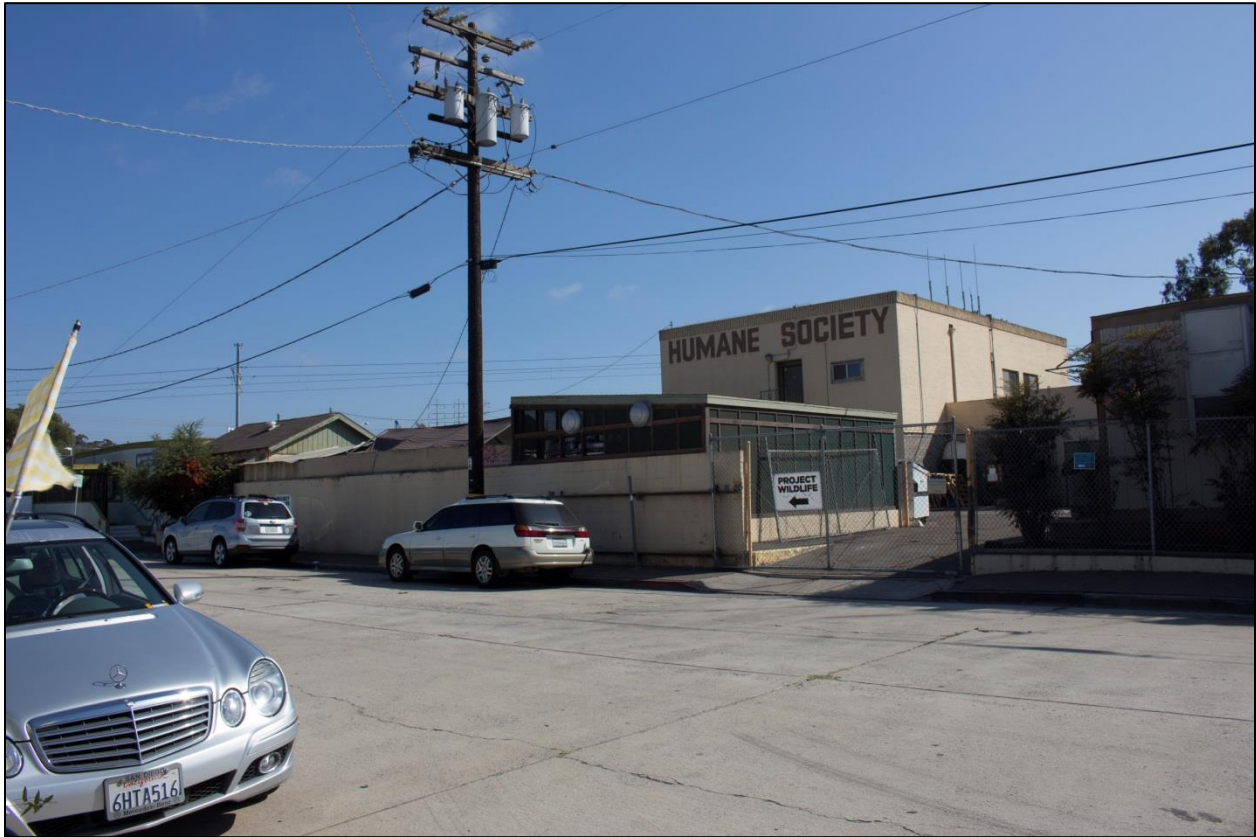
Figure 8. View of part of the east elevation; looking southwest from Custer Street (Photo credit: Dudek).
