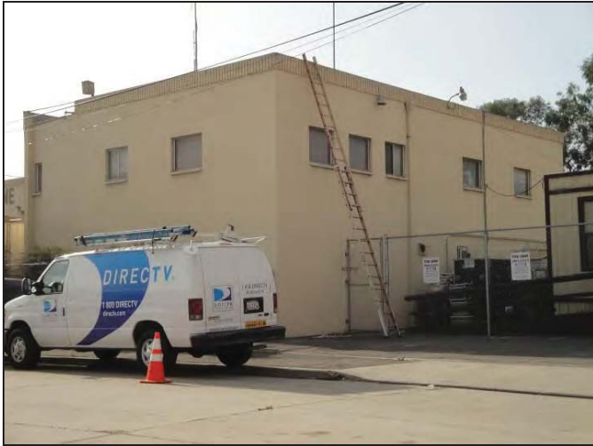
View southwest toward 877 Sherman Street from Custer Street. Taken on November 1, 2011 (Photo Accession #521-01-1413).
