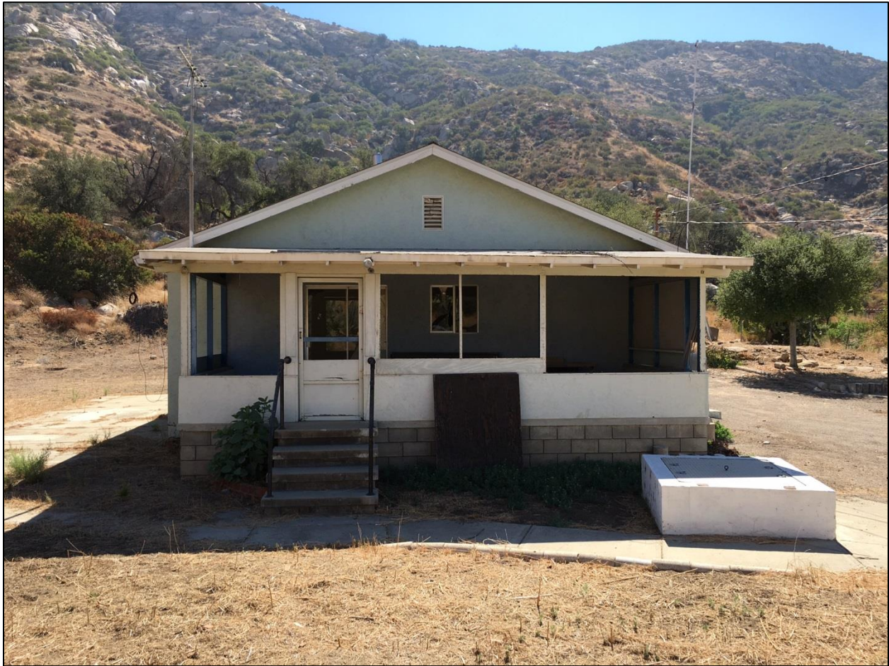
Figure 23. View of the northwest elevation, with the full-width enclosed patio addition (Photo credit: Dudek).
