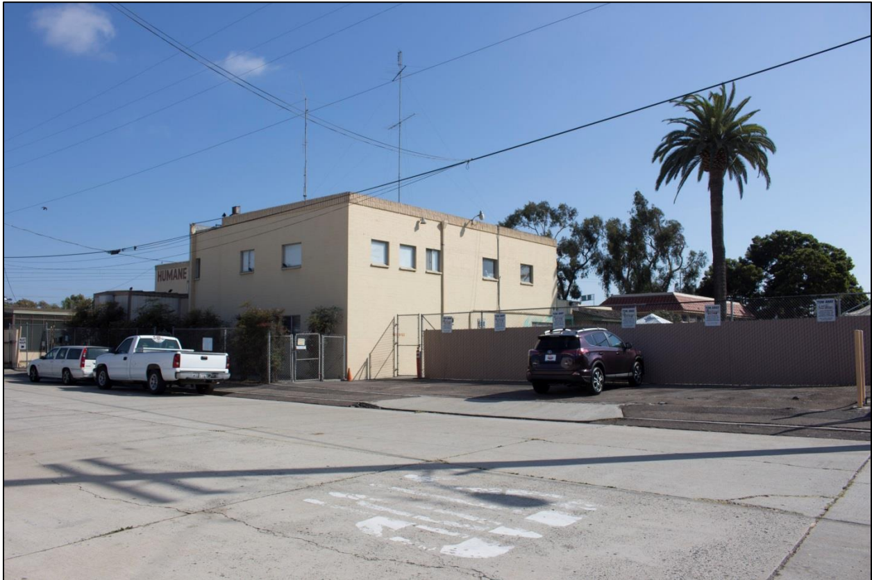
Figure 7. View of the main and east elevations; looking southwest from the intersection of Custer Street with Sherman Street (Photo credit: Dudek).
