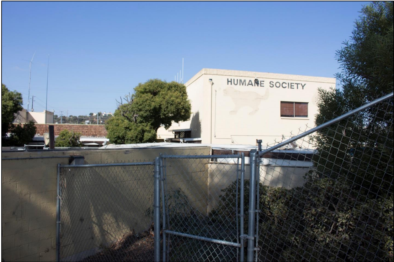
Figure 10. Eastern portion of southwest elevation; view looking east (Photo credit: Dudek).
