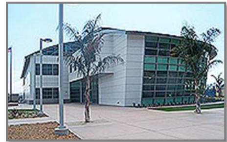
Related Facilities at the Harbor Drive Site. The Harbor Drive site already accommodates Pump Station No. 2 (the largest wastewater pump station in San Diego) and the Environmental Monitoring and Technical Services Division facility (shown above), which houses the City's water quality laboratory. Co-locating a new plant at this site saves costs, increases flexibility and reduces risks.
