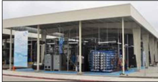
Figure 2-1. Water Purification Demonstration Project
