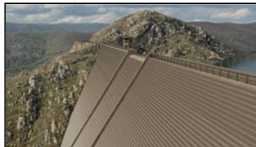
San Vicente Dam Raise. The San Vicente Reservoir expansion (architectural rendering shown above) and its integration with regional facilities make this reservoir an ideal candidate for indirect potable reuse.
