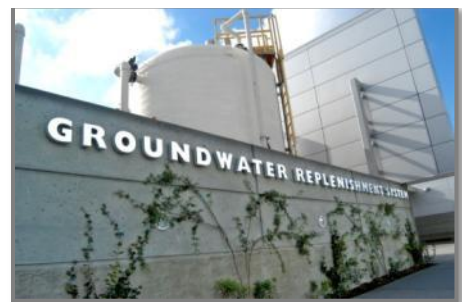
Orange County, CA Groundwater Replenishment Facility. The Groundwater Replenishment facility is just north of San Diego, and is recharging enough purified recycled water into the groundwater supply to serve 600,000 residents – with a superior water quality that is improving the basin.
