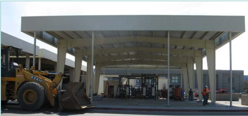
The Advanced Water Purification Facility's canopy is now installed.
