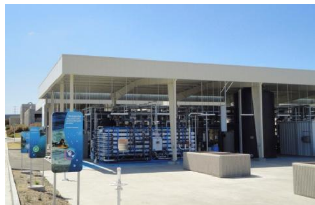
The advanced water purification facility is a component of the Water Purification Demonstration Project.
