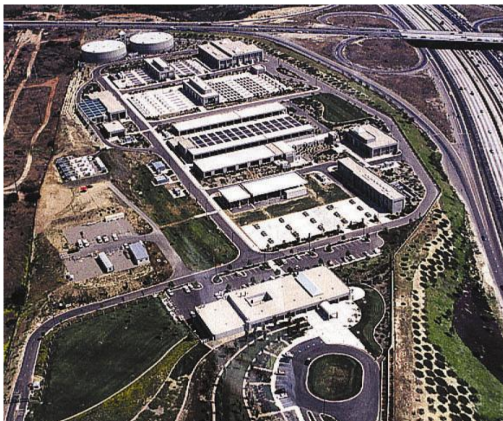
Aerial of NCWRP
