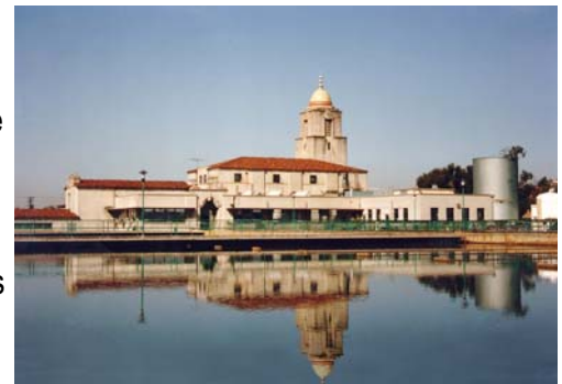
Alvarado Water Treatment Plant
