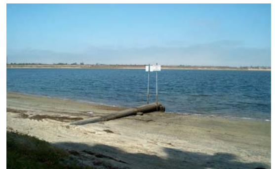
Figure I-31. Storm drains SD10-3 at North Pacific Passage.
