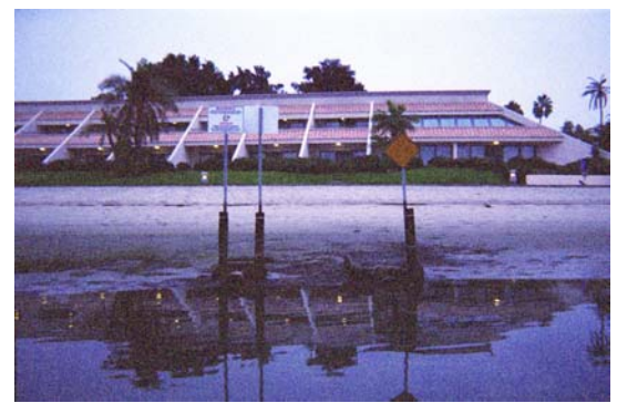
Figure I-30. Storm drain SD10-1 and SD10-2 at North Pacific Passage.
