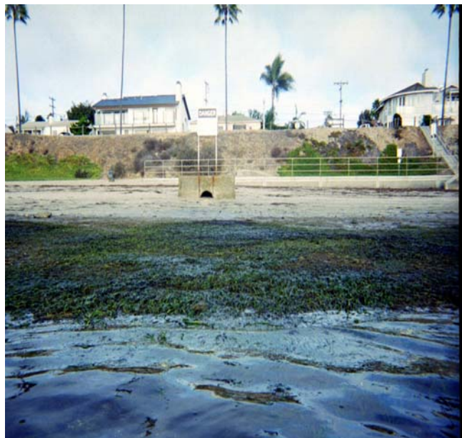
Figure I-16. La Cima Drive storm drain (SD4-2) and sampling site location.
