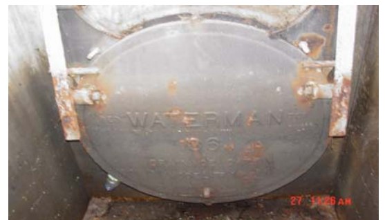
Figure I-32. Storm drain SD10-3 at North Pacific Passage showing debris in check valve.
