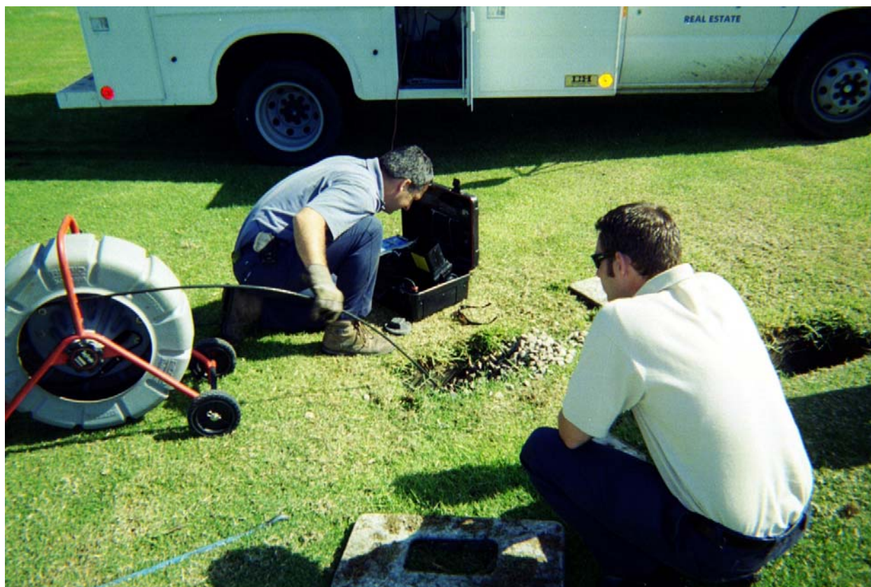
Figure 4. Photograph of typical CCTV investigation in Mission Bay Park.
