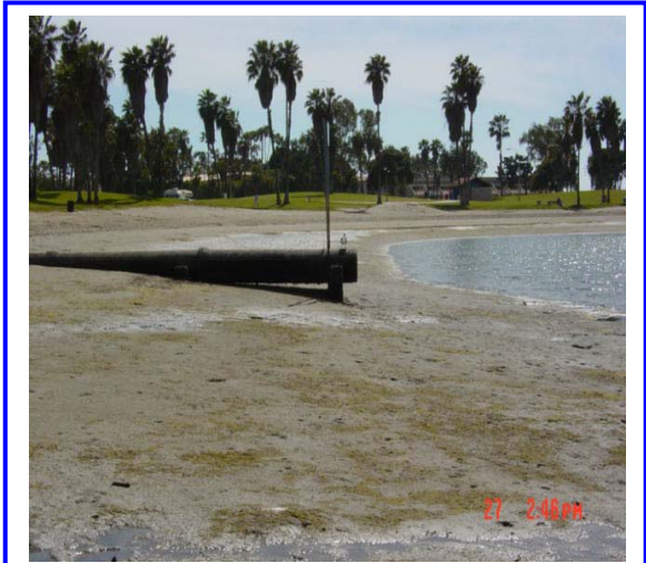
Figure I-28. Photograph of storm drain SD9-2 on the east side of Leisure Lagoon.
