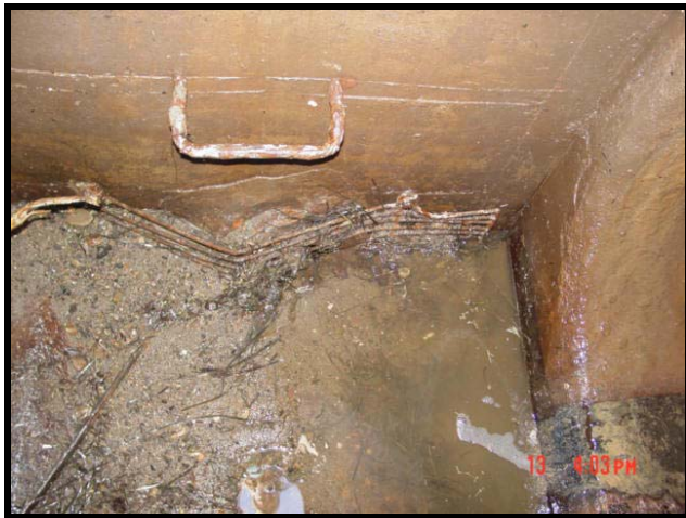
Figure I-1. Photograph of water entering a storm drain diversion vault (on the right side of the photograph), the diversion berm (on the left side of the photograph), and grate. The vault shown here is filled with sediment that had washed up from the Bay.
