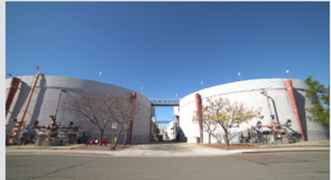
The Metropolitan Biosolids Center.
