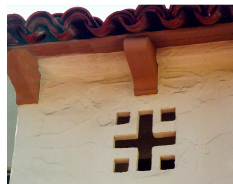
Architectural details incorporated into style of the building.
