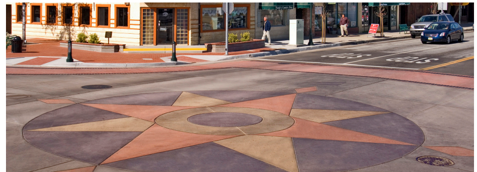
Crosswalk striping and intersection specialty paving enhance the area and distinguish the pedestrian realm from vehicular areas.
