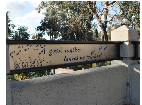
Public art incorporated into bridge railing.
