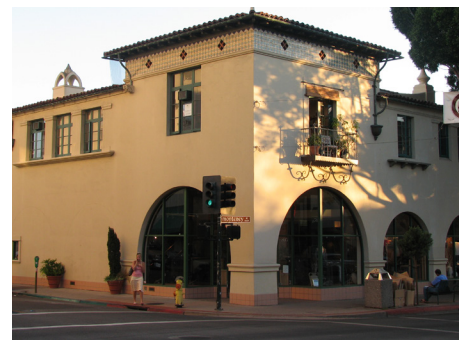
Tile roof, tile detailing, arches, and windows reflect historic architectural character.
