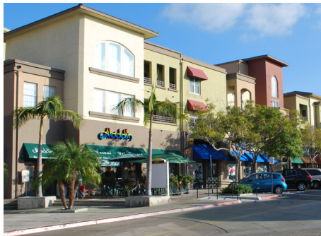
Ground floor uses activate street frontage.
