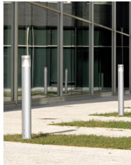
Bollards light paths and entry areas.
