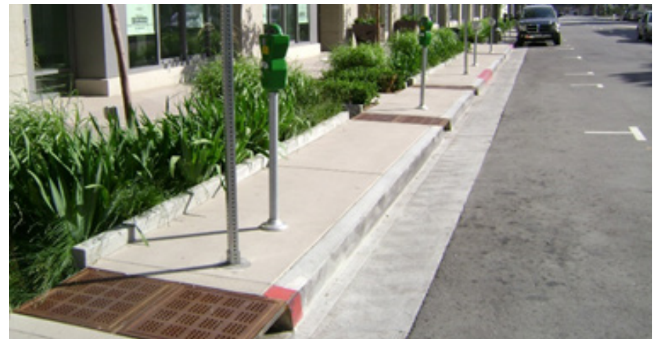
Flow-through planters are used to provide filtration of surface runoff.
