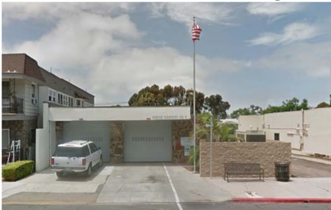
Google Maps: Fire Station 8 in Mission Hills
