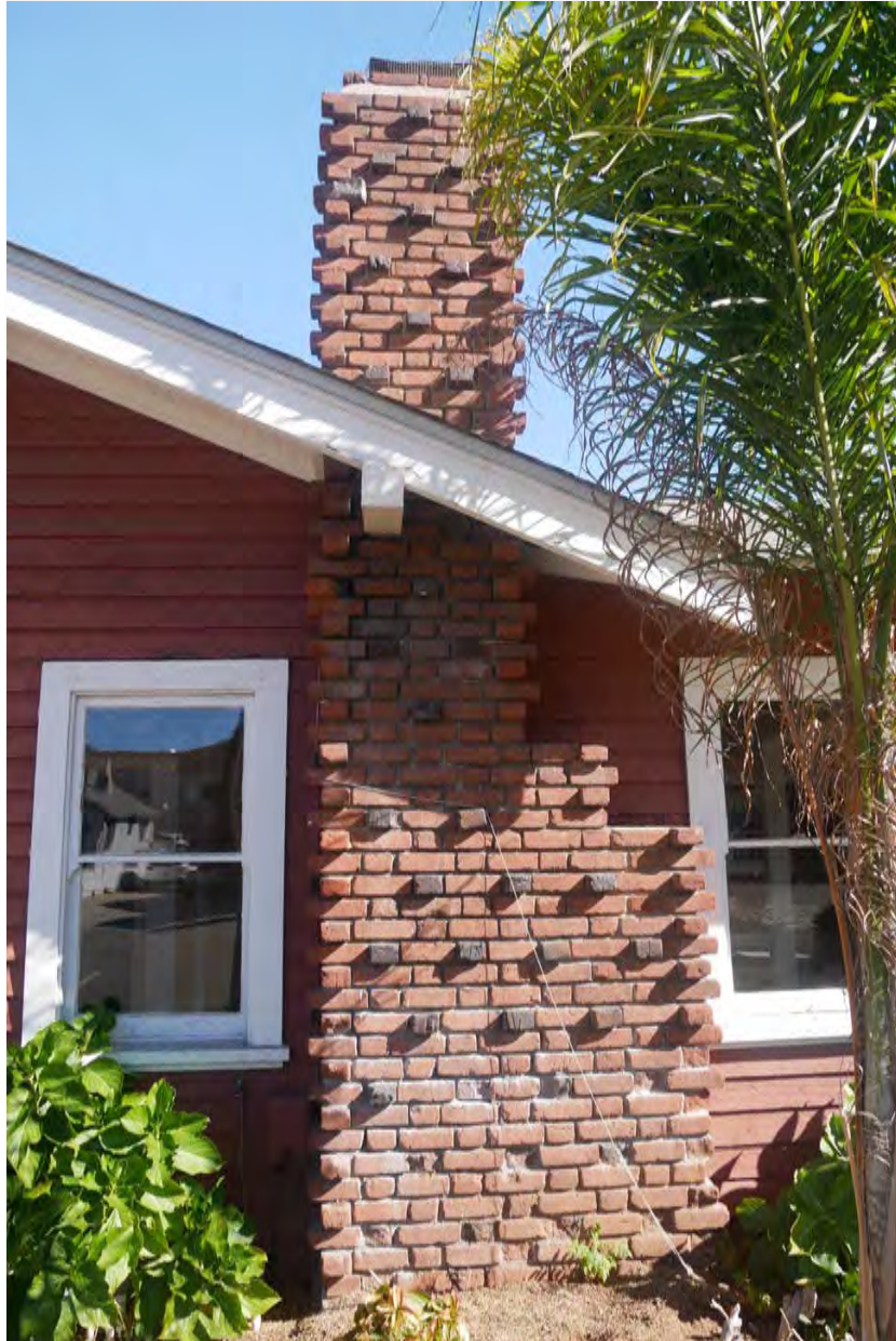
Photograph #5: West elevation, chimney
