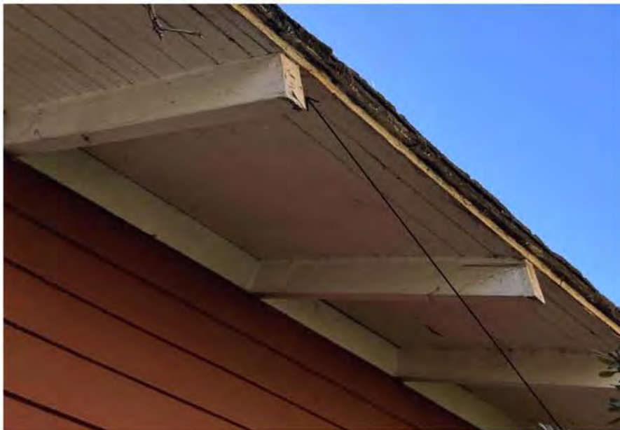
Roof Outrigger failure. Siding must be removed, framing repaired and outrigger replaced in kind
