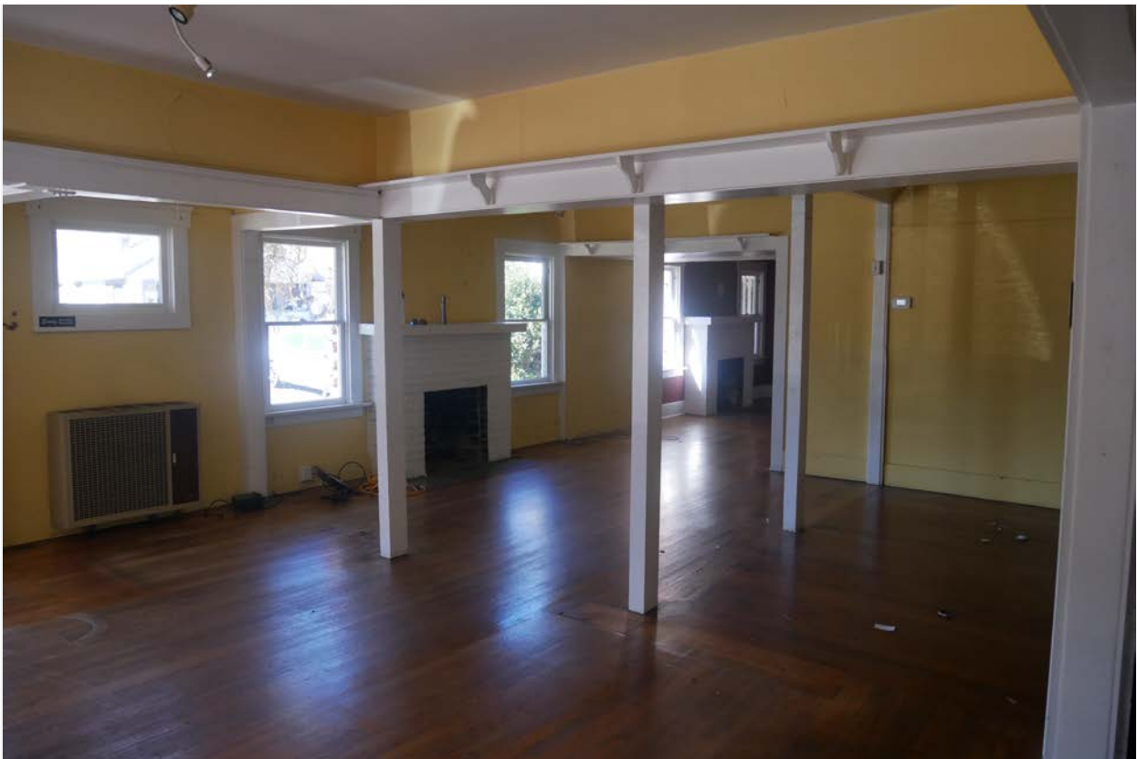
Photograph #43: Interior, walls removed between units
