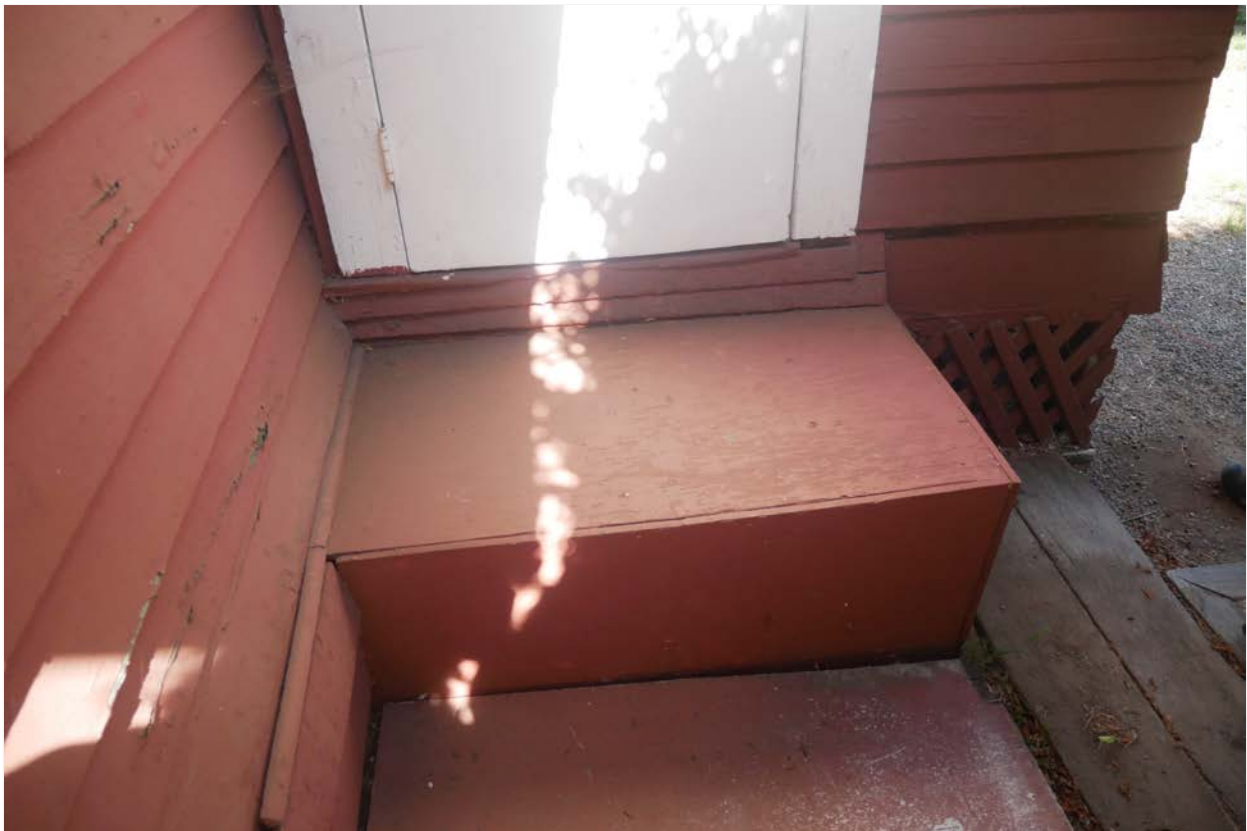
Photograph #13: South elevation, enclosed rear porch door stoop
