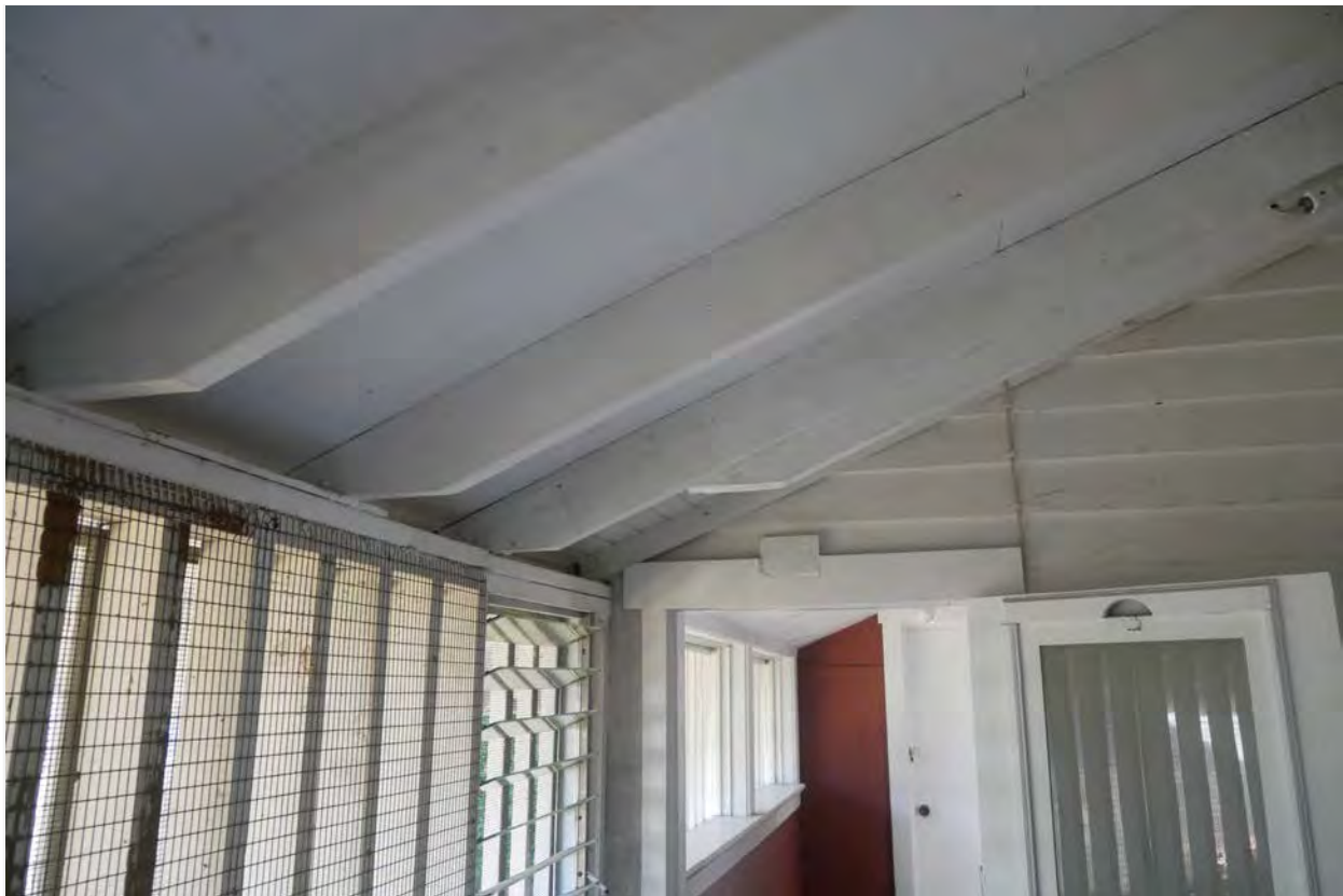
Photograph #36: Rear yard, recess infill, looking southeast
