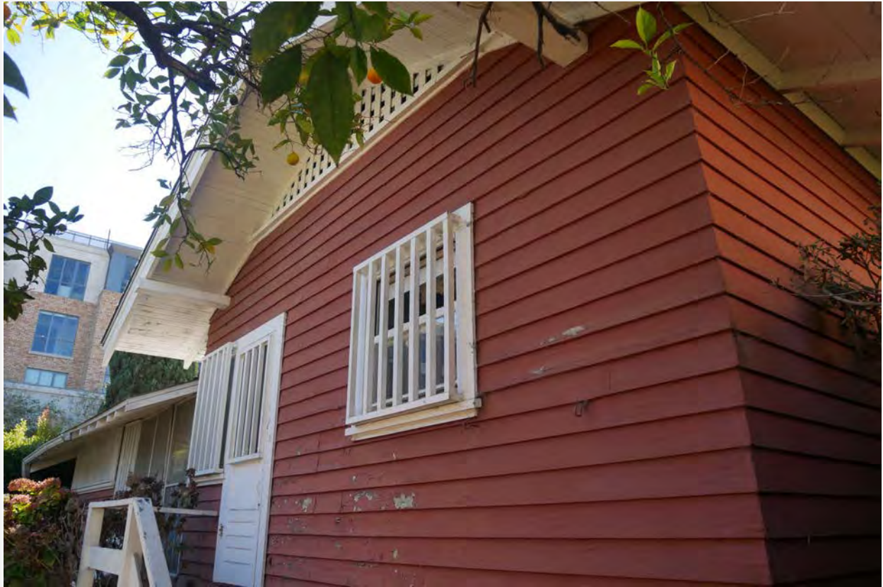
Photograph #18: East elevation, enclosed rear recess
