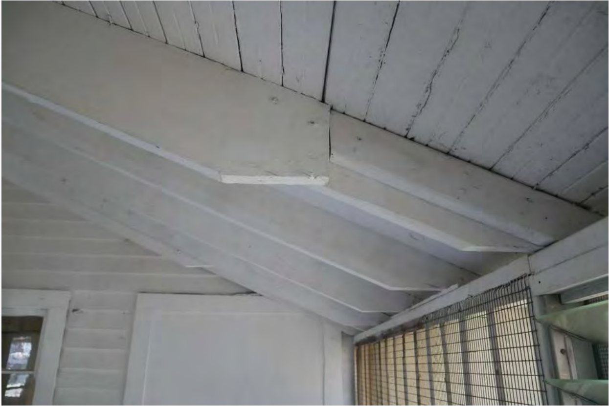
Photograph #32: Rear yard, recess infill, looking north
