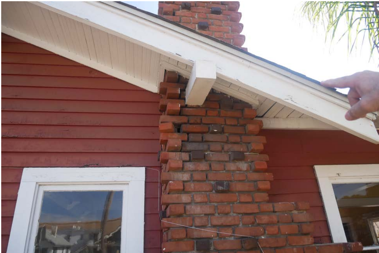
Photograph #23: West elevation, chimney roof intersection
