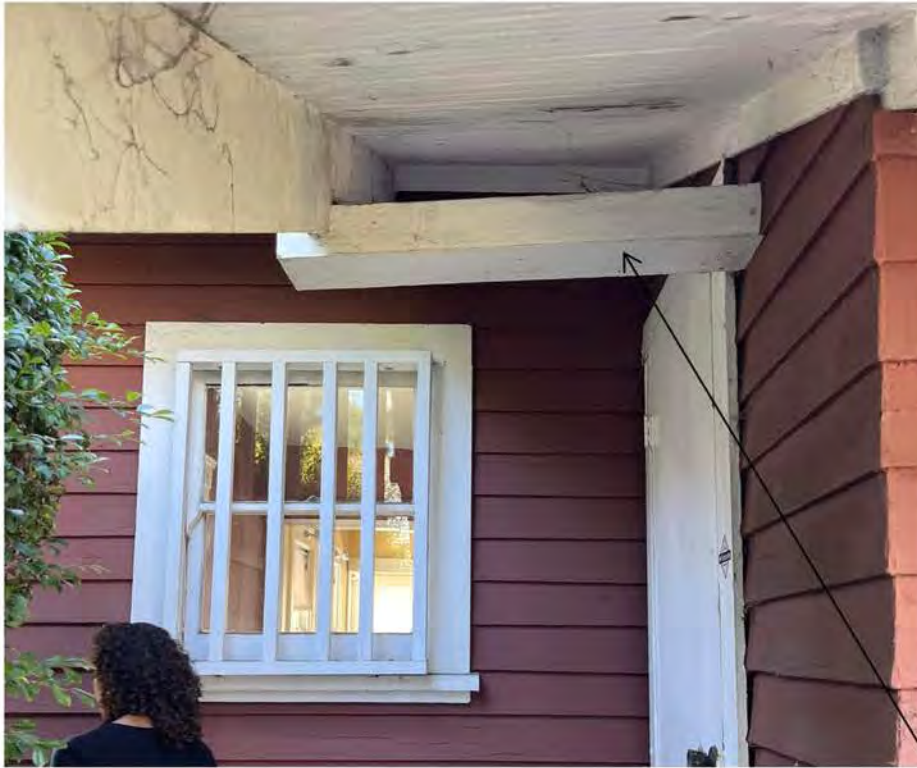
Roof Outrigger failure. Siding must be removed, framing repaired and outrigger replaced in kind
