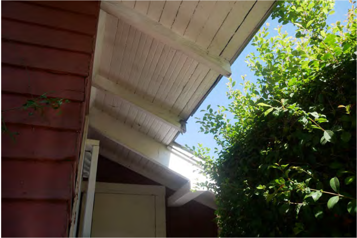
Photograph #16: South elevation, enclosed rear porch roof edge
