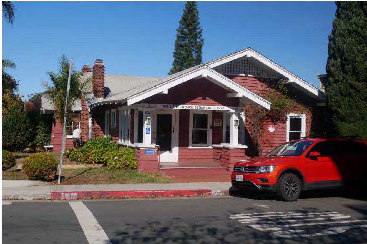
Photograph #2: South elevation, Fort Stockton Drive
