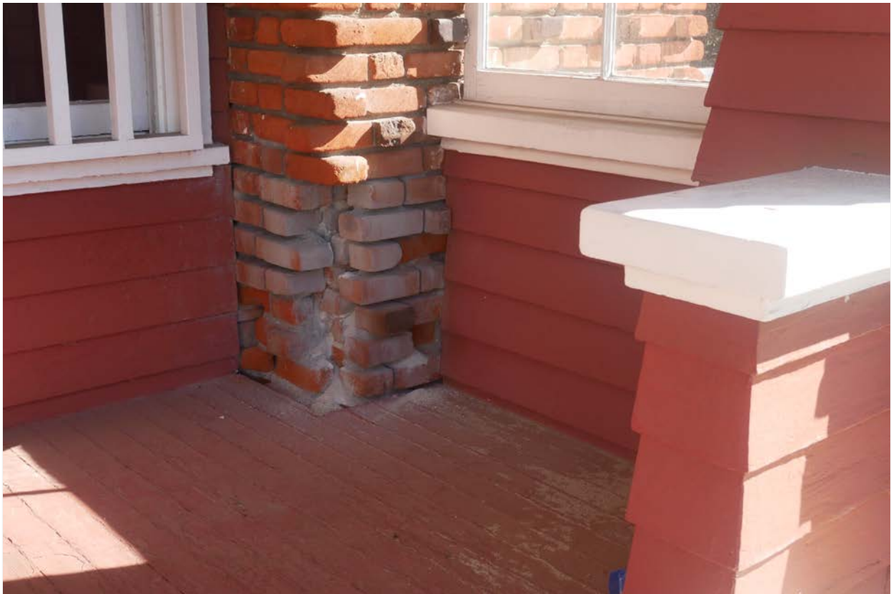
Photograph #7: West elevation, Goldfinch Street, front porch
