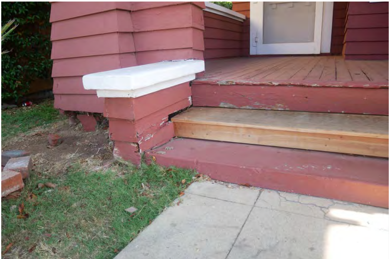
Photograph #9: West elevation, Goldfinch Street, front porch
