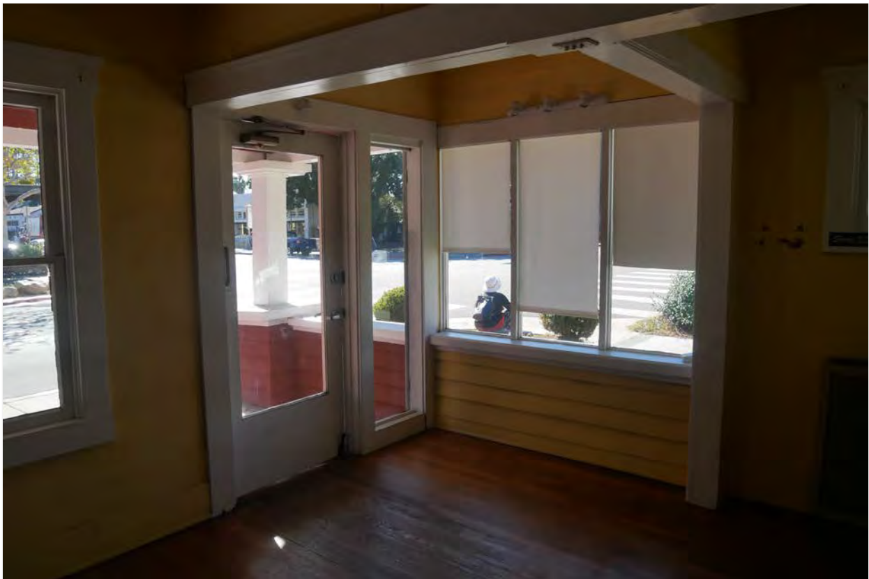
Photograph #45: Interior, walls removed at former porch recess
