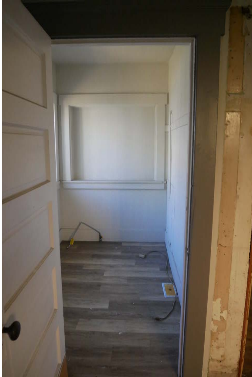
Photograph #47: Interior, porch window into exterior recess blocked in
