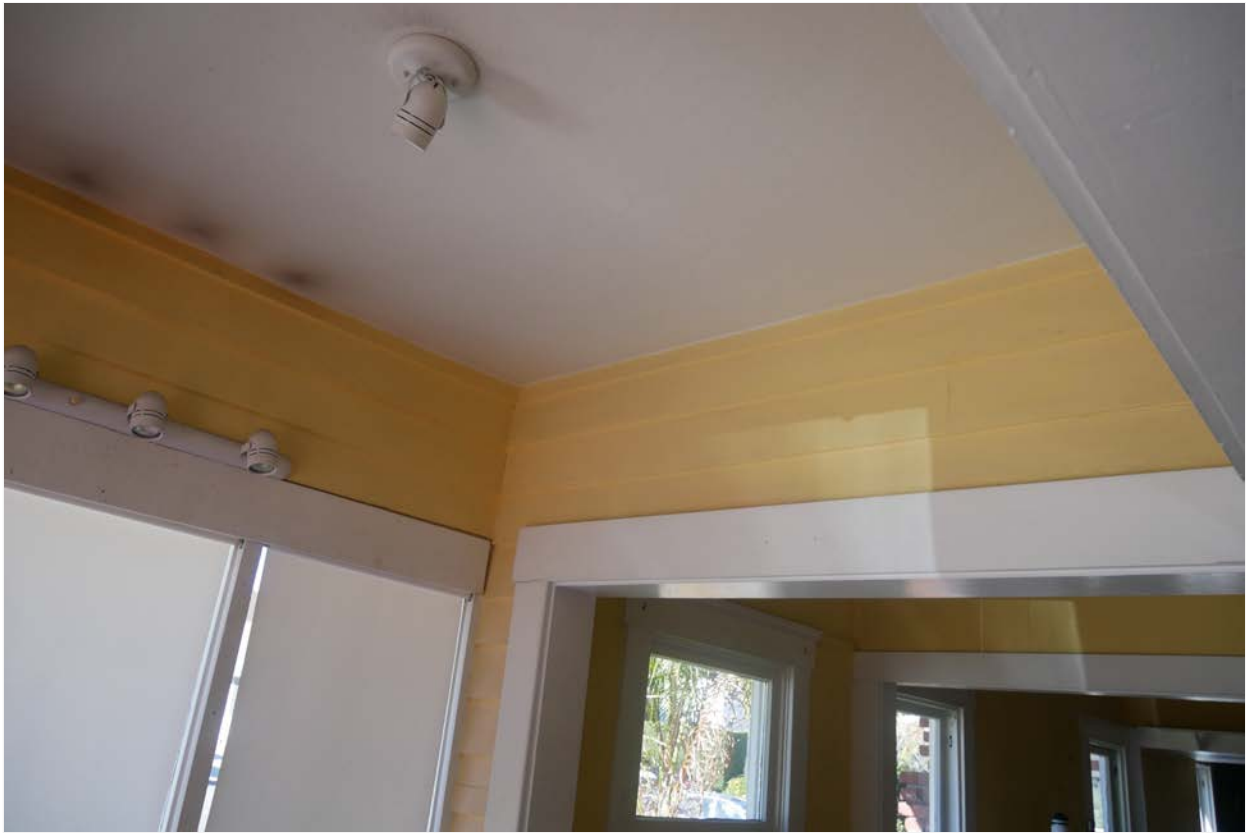
Photograph #44: Interior, walls removed at former porch recess
