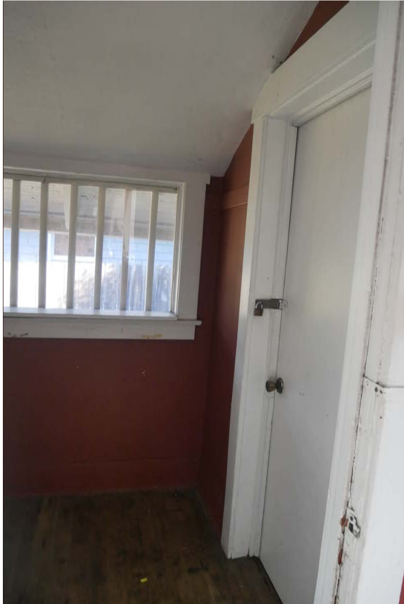
Photograph #30: Enclosed rear porch with plastic windows, from interior looking east
