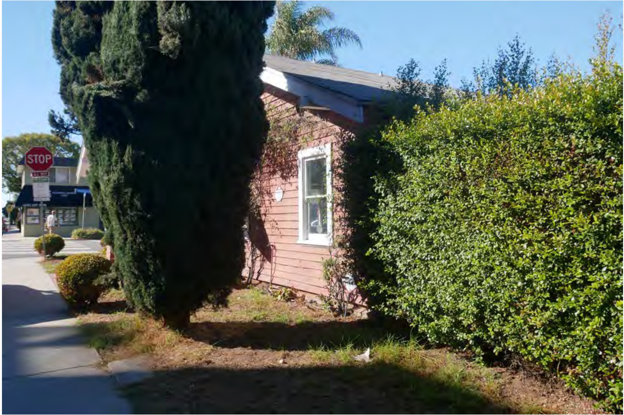
Photograph #12: South elevation, Fort Stockton Drive
