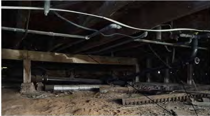
Archaic plumbing system. It would be more economical to address at time of foundation replacement
