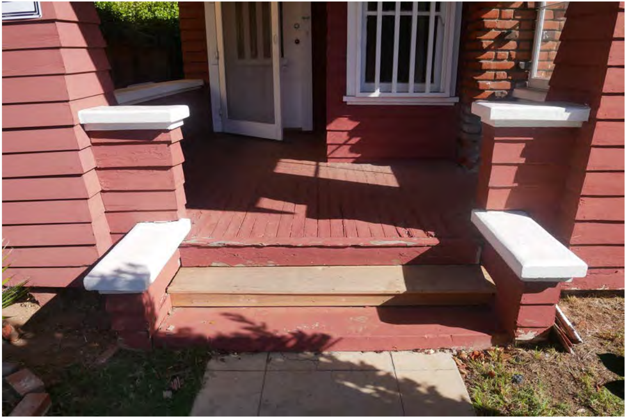
Photograph #6: West elevation, Goldfinch Street, front porch
