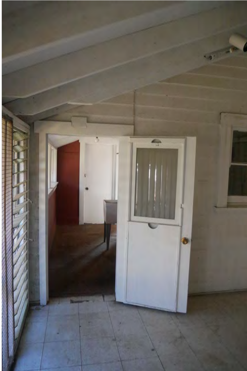
Photograph #37: Rear yard, recess infill, looking south into enclosed rear porch
