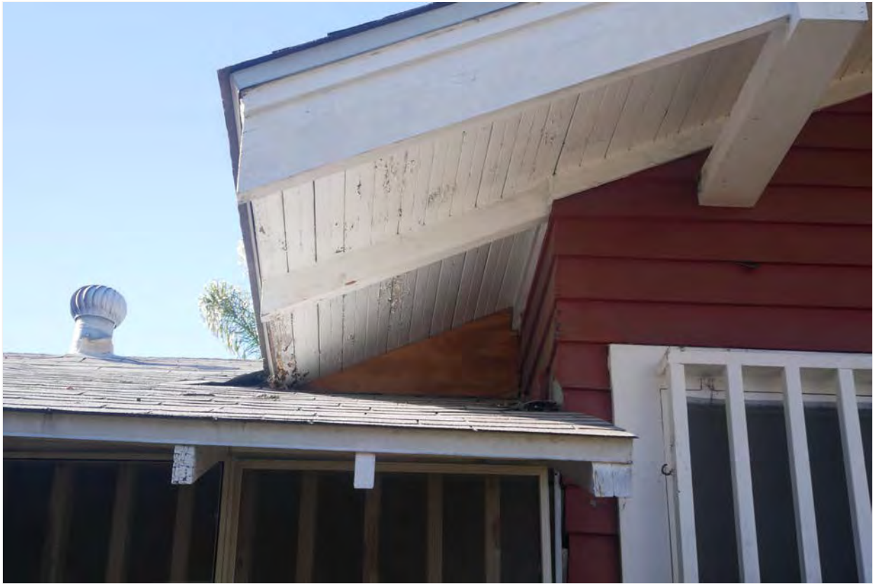
Photograph #22: East elevation, roof extension intersection
