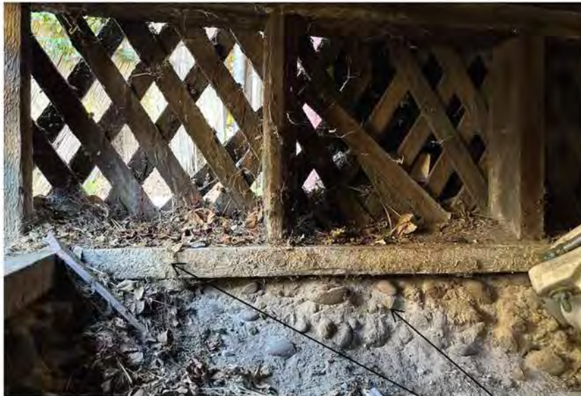
Archaic plumbing system. It would be more economical to address at time of foundation replacement
