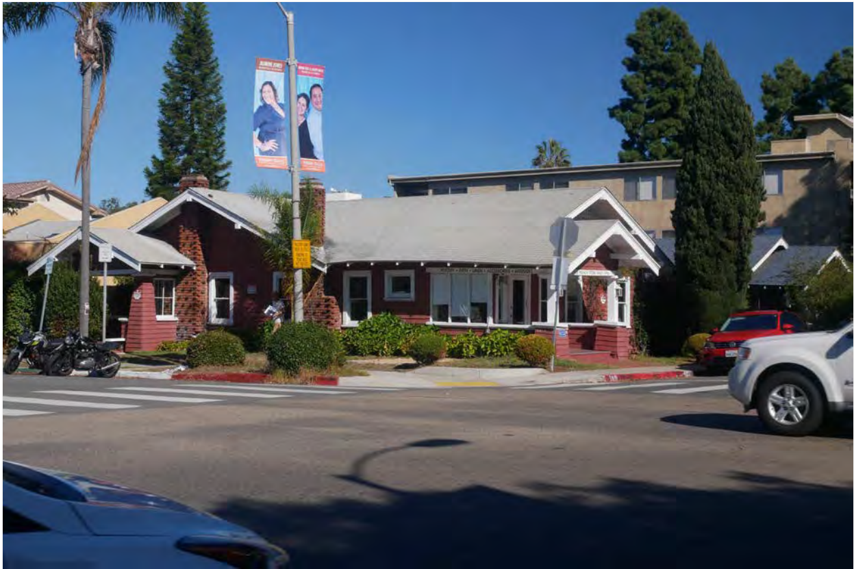
Photograph #1: Southwest corner at Fort Stockton Drive and Goldfinch Street
