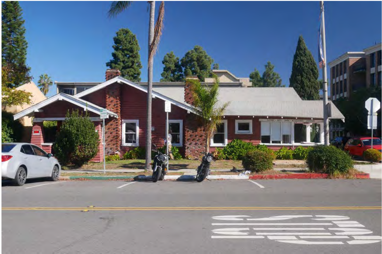
Photograph #3: West elevation, Goldfinch Street
