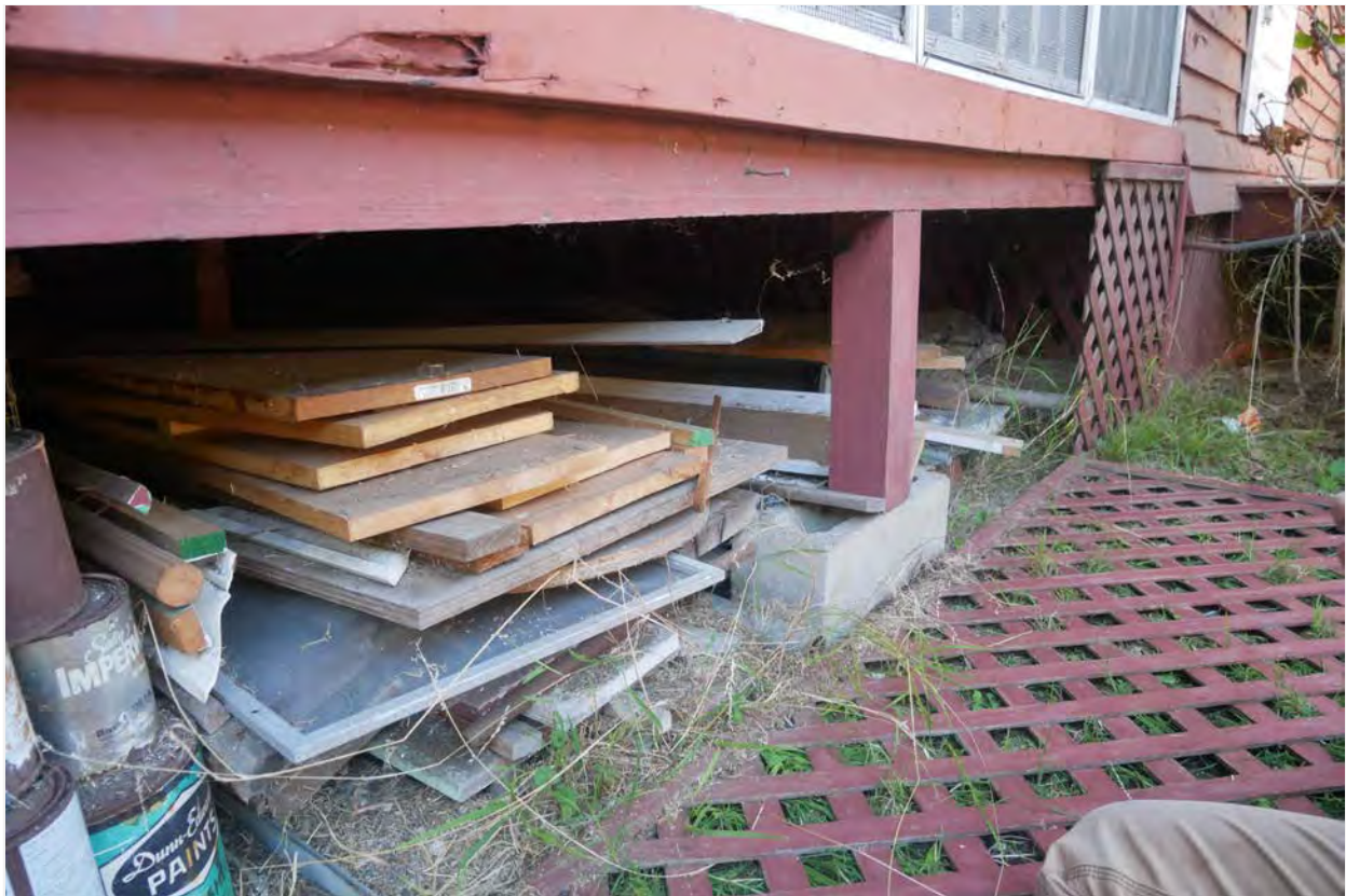
Photograph #19: East elevation, porch infill
