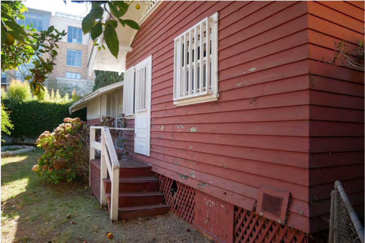
Photograph #20: East elevation
