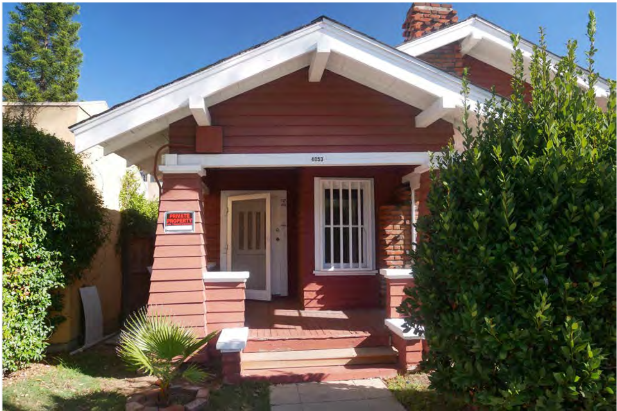
Photograph #4: West elevation, Goldfinch Street
