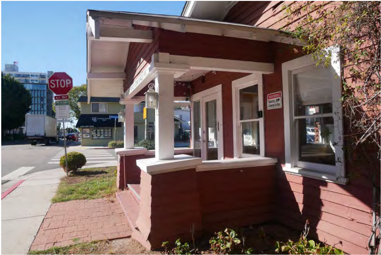
Photograph #10: South elevation, Fort Stockton Drive, front porch
