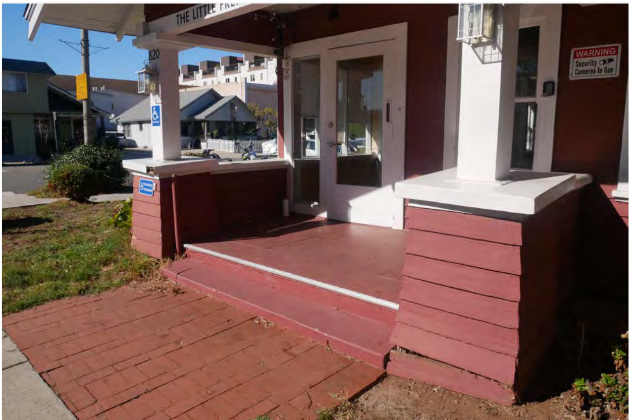
Photograph #11: South elevation, Fort Stockton Drive, front porch
