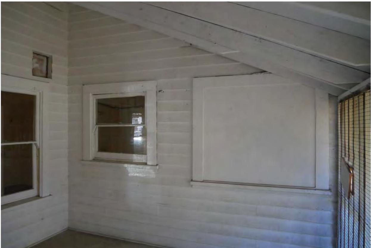
Photograph #33: Rear yard, recess infill, looking north
