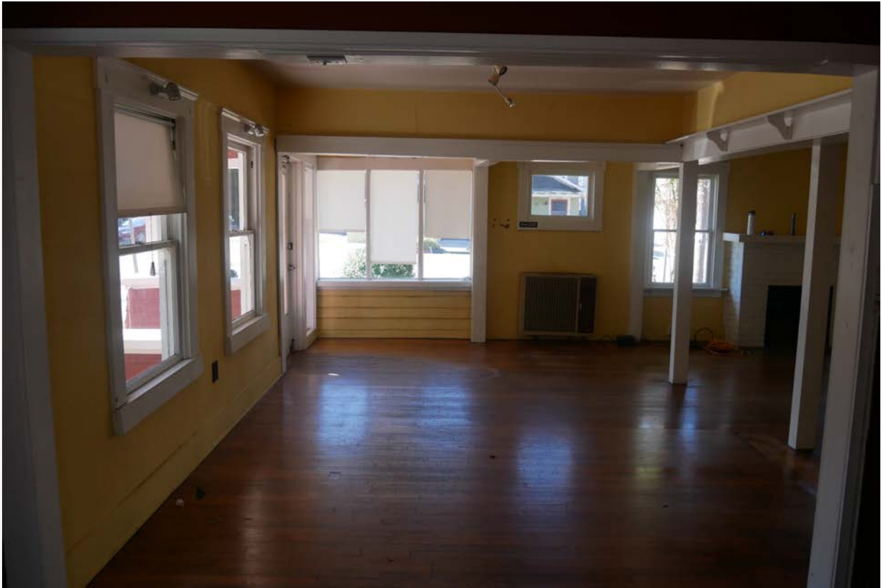
Photograph #42: Interior, walls removed at former porch recess
