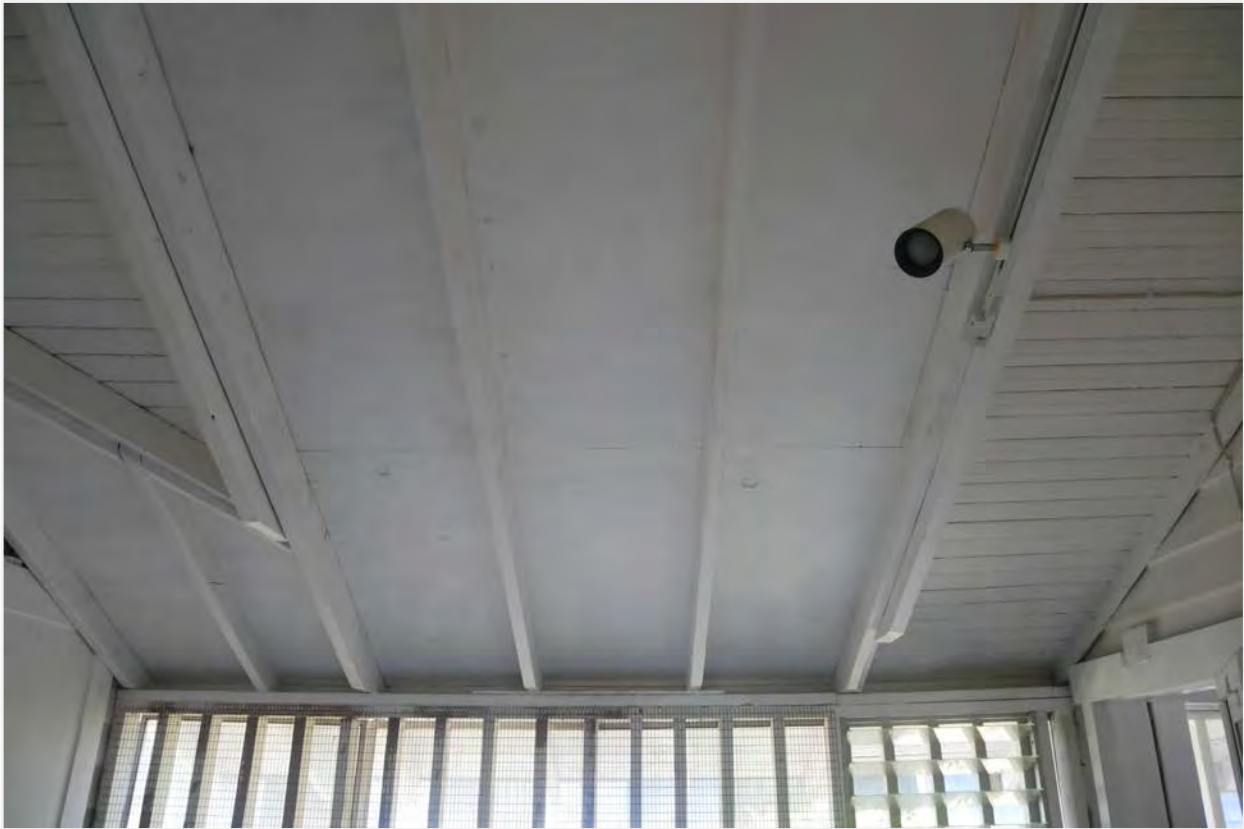
Photograph #40: Rear yard, recess infill, looking at roof
