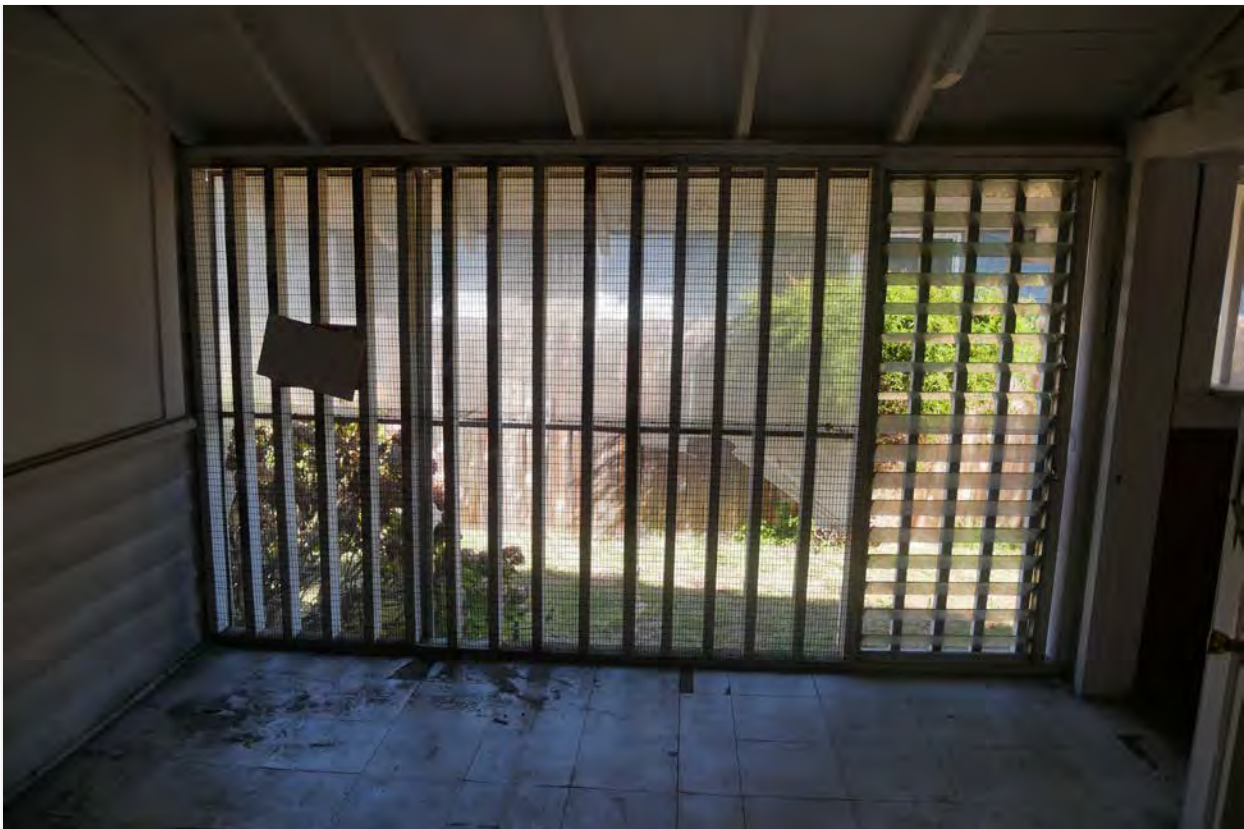
Photograph #41: Rear yard, recess infill, looking east
