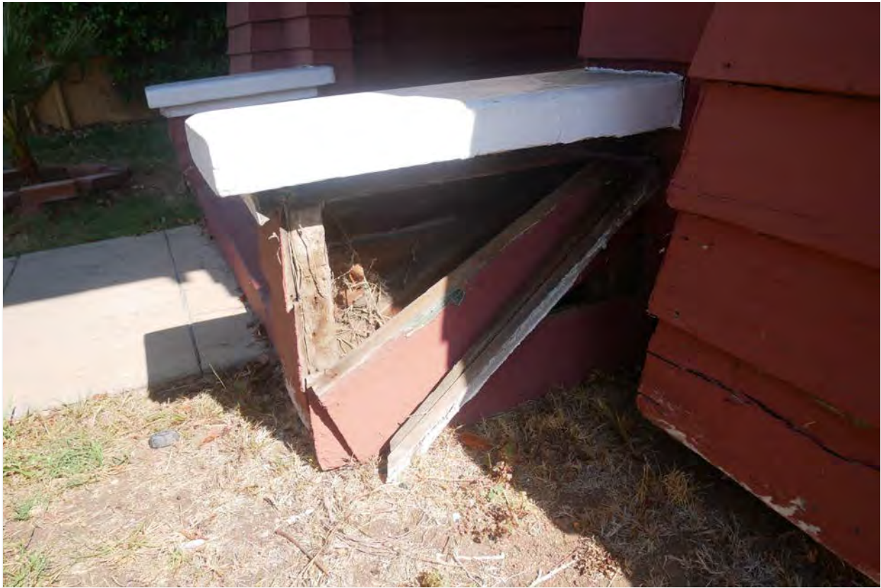
Photograph #8: West elevation, Goldfinch Street, front porch
