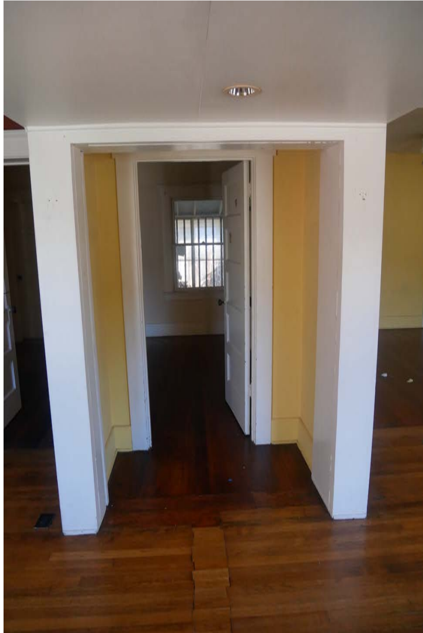
Photograph #46: Interior, walls removed between units and into bedrooms
