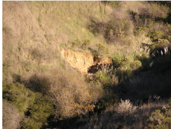
Figure 4-44. Evidence of Scour in the Drainage below the Autoport Mall Outfall
