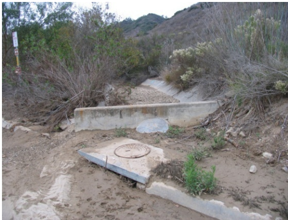
Figure 4-41. Photos of Deposition on Flintkote Avenue
