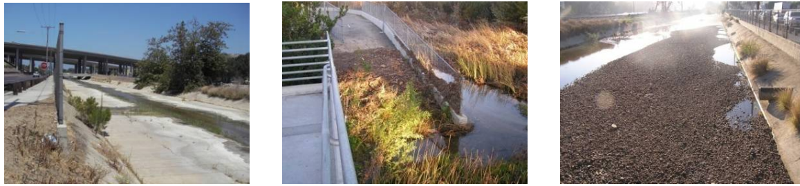
Figure 1-7. Concrete Channel at Carroll Canyon Creek
