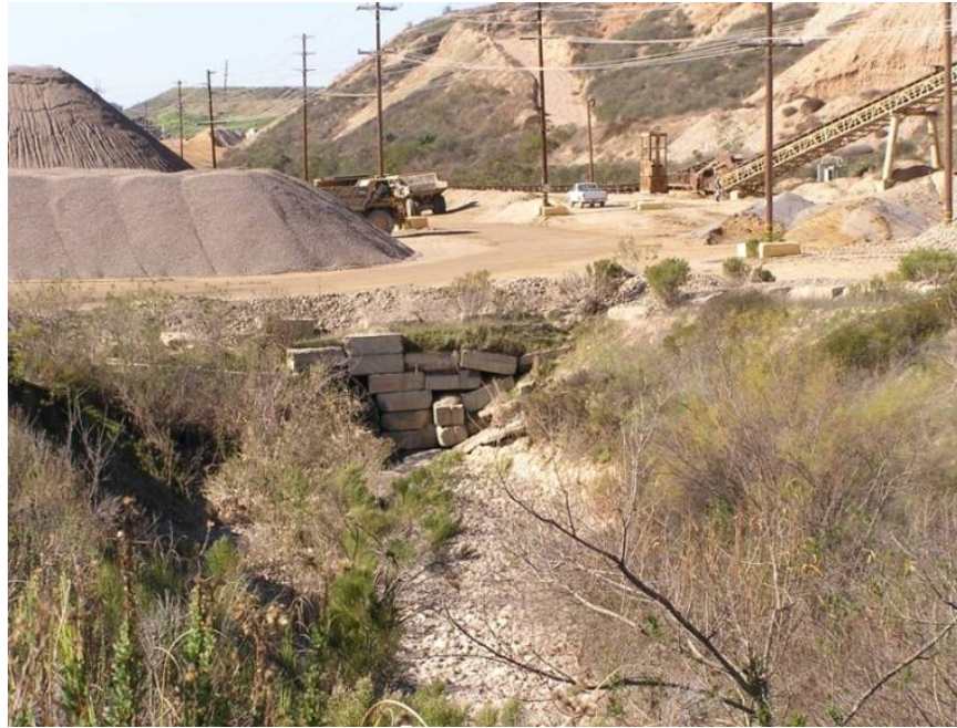
Figure 4-55. Aggregate Stockpiles near a Tributary to Carroll Canyon Creek
