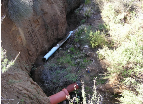
Figure 4-9. MS4 Point of Discharge
