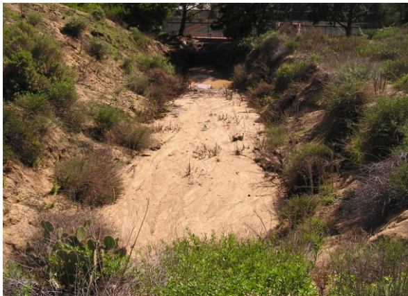
Figure 4-11. Sediment Basin (view looking into and above the basin)
