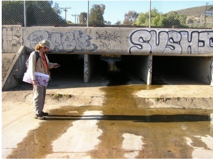
Figure 4-35. Roselle Street Drainage Outfall at Carroll Canyon Creek
