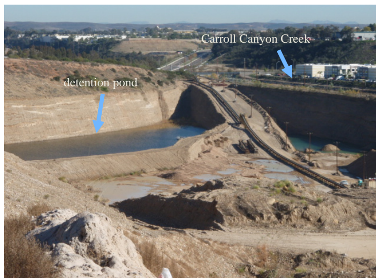
Figure 4-58. Mining Operations at Vulcan's Carroll Canyon Facility
