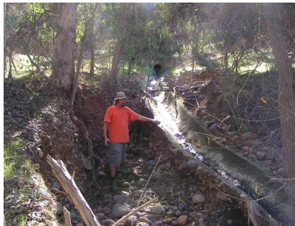
Figure ES-2. Eroded Brow Ditch in Carroll Canyon
