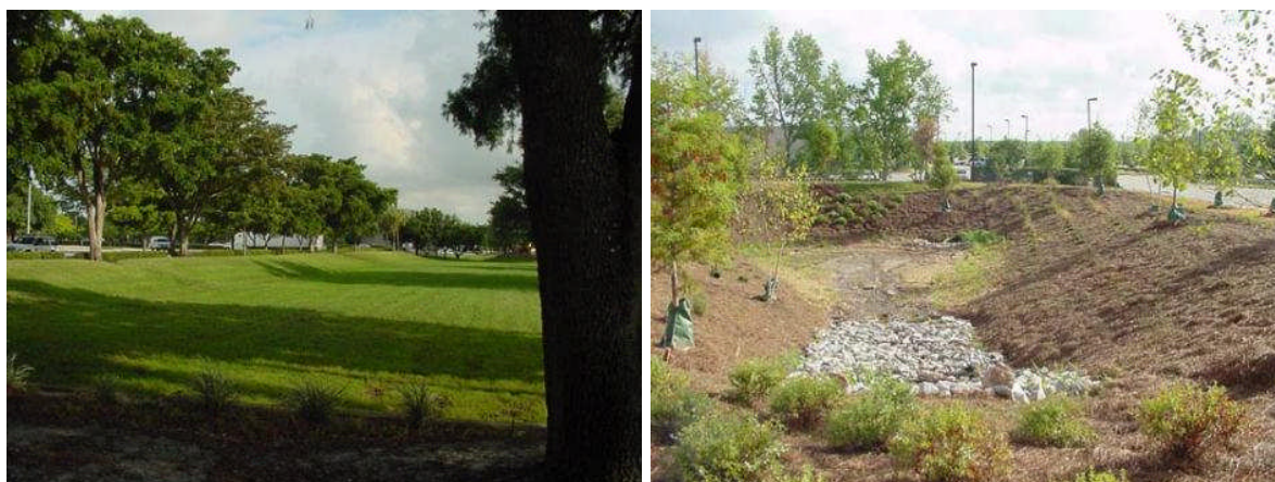
Figure I-14. Examples of dry extended detention basins
