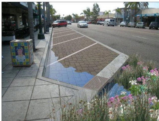
Figure I-5. Permeable pavement parking area in the right-of-way
