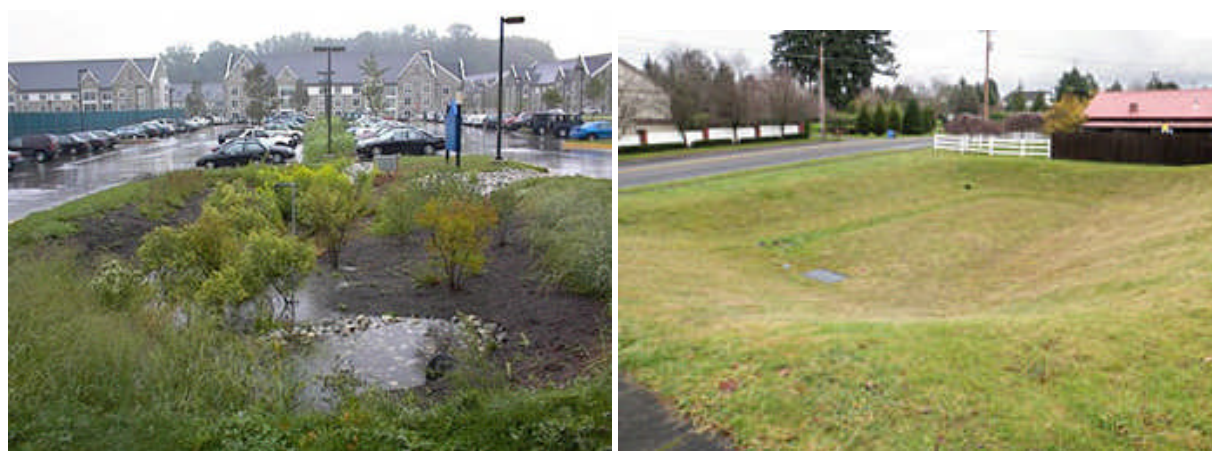
Figure I-12. Typical surface infiltration basins
