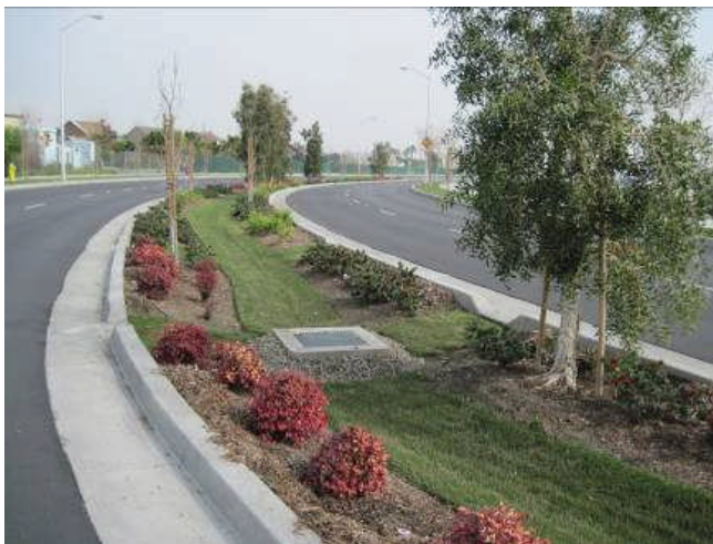
Figure I-3. Road median bioswale
