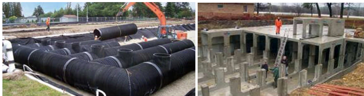
Figure I-15. Examples of subsurface detention systems
