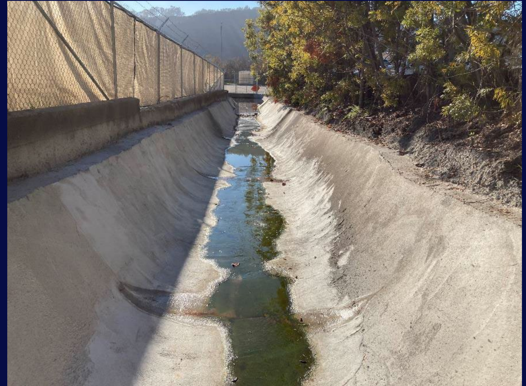
Post-Maintenance Concrete Conditions (1/5/22)
