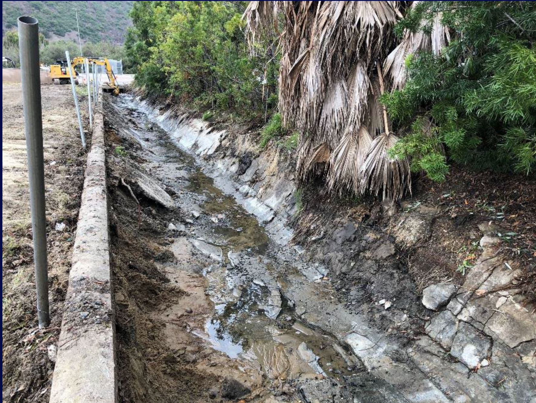
Pre-Maintenance Concrete Conditions (10/6/21)
