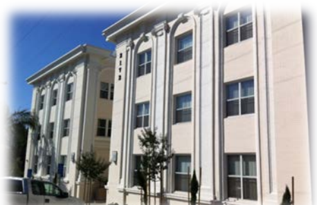
Image 12: Completed pictures of Parker-Kier major rehabilitation project.
