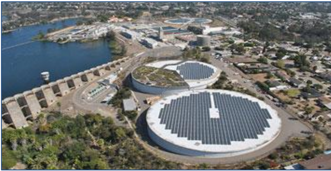
Alvarado Water Treatment Plant project
