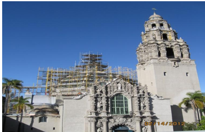
Museum of Man Dome Restoration & Repair
