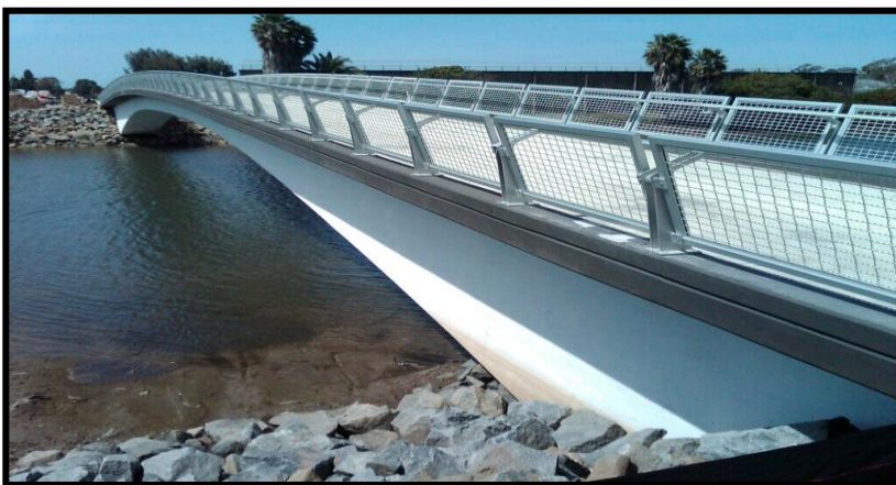
Rose Creek Bikeway and Pedestrian Bridge
