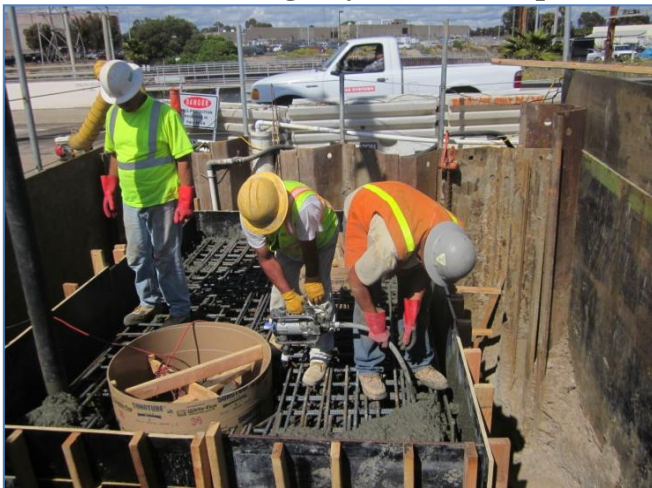
Pumping and vibrating concrete for vault 2 (south of Chollas Creek crossing).
