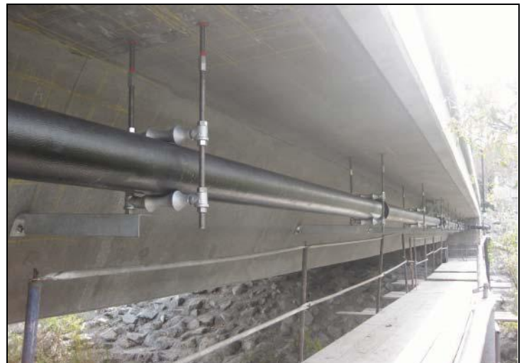
Installation of ductile iron pipe for recycled water located along bridge at Carmel Country Road.
