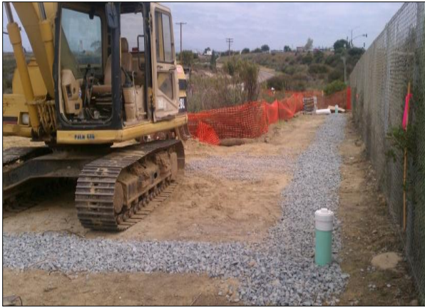
French drains in gravel pit.
