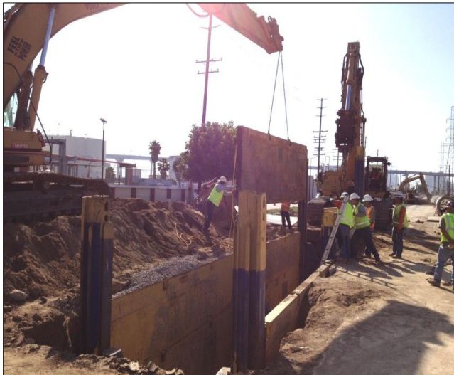
Contractor is setting slide rail system for installation of 48-inch trunk sewer pipe.
