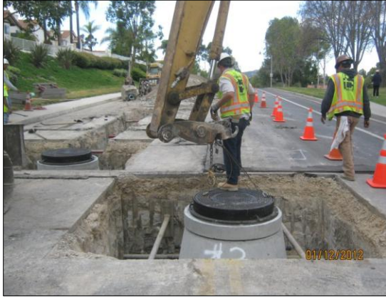
Installation of two new discharge manholes associated with sewer pump station number 73 secondary force main.
