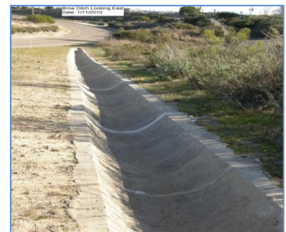
Existing concrete brow ditch.
