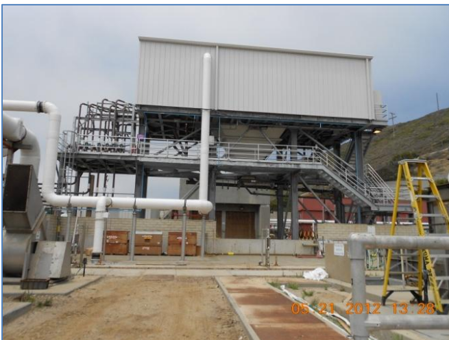
Completed Interim Grit Processing Facility (South View)
