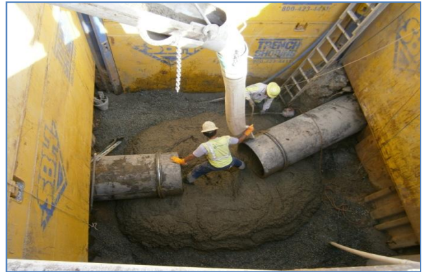
The workers are inside a pit pouring concrete to build a sewer manhole base.
